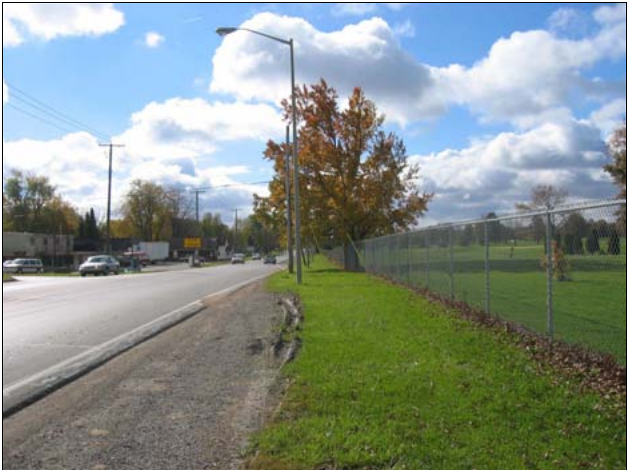
Figure IV.21 View looking south along the eastern park edge and Hessen Cassel Road. Much of the park perimeter along the street is lined with a chain-link fence. Though this clearly delineates the park edge, the fence restricts access into the park and creates an uninviting park character. (R- FWP-MCM-VT-0014.jpg) Courtesy Heritage Landscapes.
