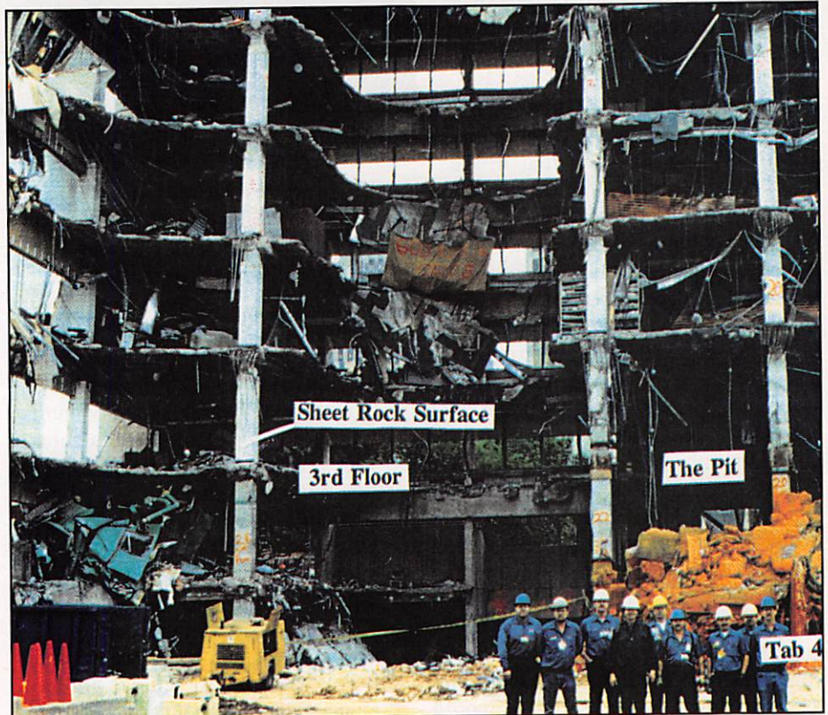
According to the official scenario, the truck bomb collapsed column B3, yet failed to rip most of the sheetrock and decorative facade off adjacent columns.
