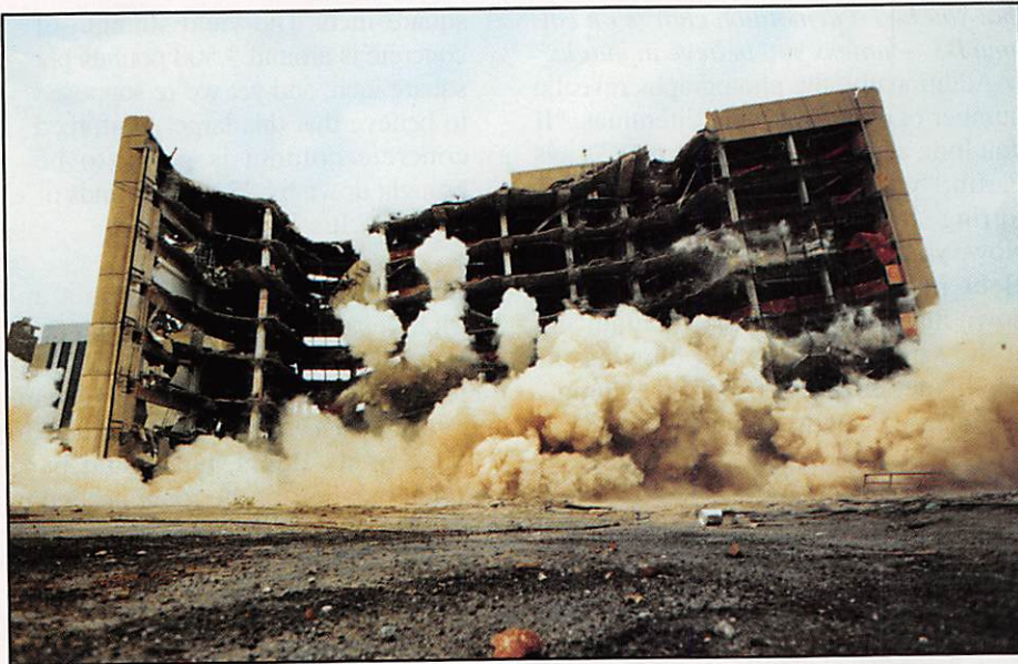
Final demolition of the Murrah Building took less than 150 pounds of explosives.
