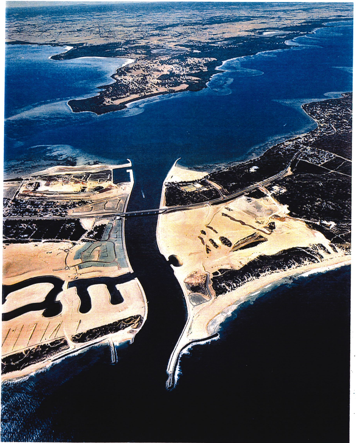
The Dawesville Channel opening into the Harvey Estuary on the upper right. Peel Inlet is on the upper left.
