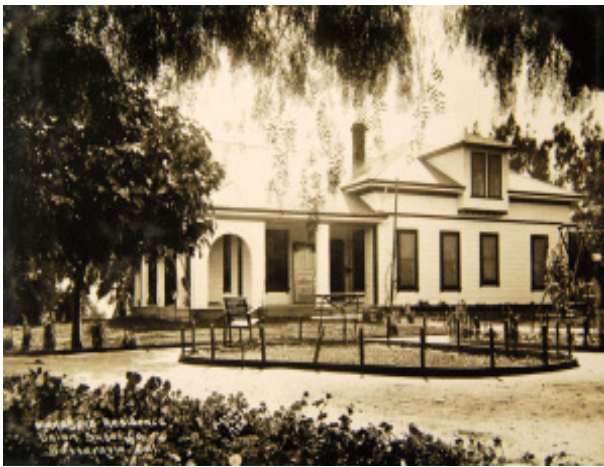
#1. This is the site of the Plant Managers large impressive house. The terrain drops off just behind where the house stood, to a large depression that once contained a natural lake.
