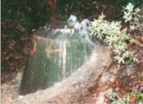
All sewer mains have provision for emergency overflow when blockages occur. Unfortunately illegal stormwater run-off also enters the system during heavy rain, directly polluting Park waterways.
