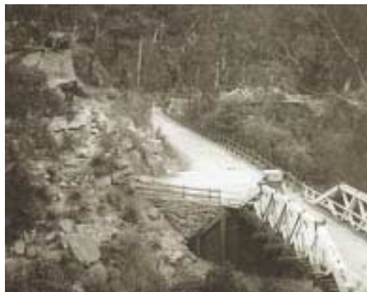
The Galston Gorge bridges in the 1920s. Both bridges used the strong McPherson strut style of construction seen clearly here on the bridge now replaced by a concrete arch.
