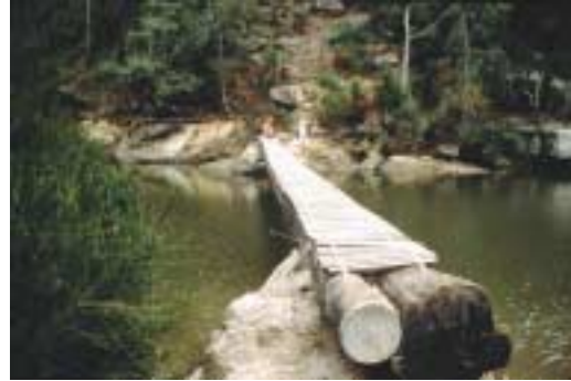
The Calna Creek twin-log bridge. This is crossed as part of Walk 10. Walk 8 passes it without crossing.
