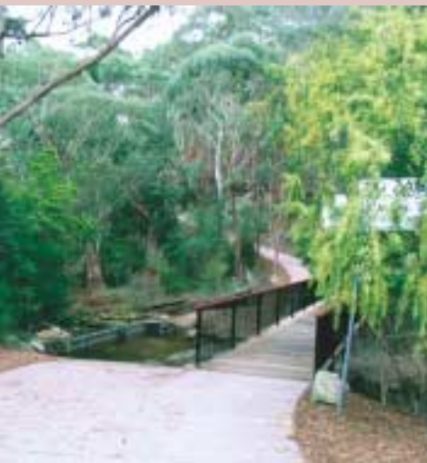
Trash rack and sediment basin beside the new bridge over Zig Zag Creek off the end of Bellamy Street, Pennant Hills
