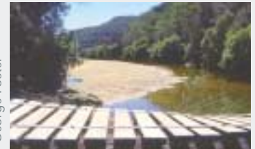
Sandbar at the entrance to Calna Creek from the twin-log bridge
