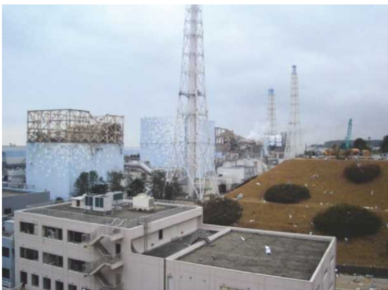
Abb. 18: Fukushima Dai-ichi am 15.3.2011; Foto: Tokyo Electric Power Company Holdings, Inc.
