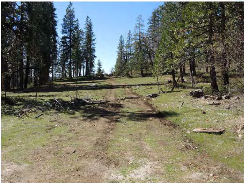
Photo 3: Unauthorized route and damaged barbed wire fence at Omo Ranch Rd. May 11, 2022
