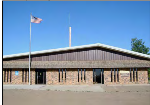
Figure 4. Grand River Ranger District office, Lemmon, SD. April 2007.
