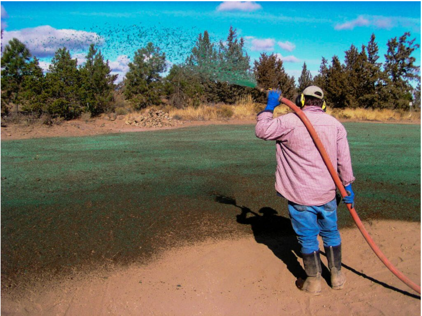
Figure 15. Hydroseeding a native plant mix including sulphur-flower buckwheat at the Deschutes National Forest Ranger District Office in Bend, OR. The broadcast hydromulch and seed was applied in fall 2011 using sulphur-flower buckwheat and other native plant seed collected about 10 miles south. The site was irrigated. Photo: C. Powers, USFS.
