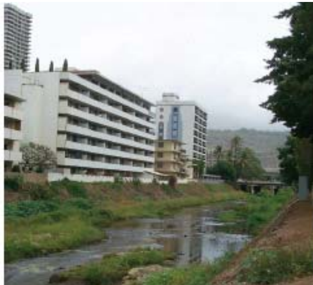
Urbanized channel in Oahu. Photograph by Anne Brasher, USGS.
