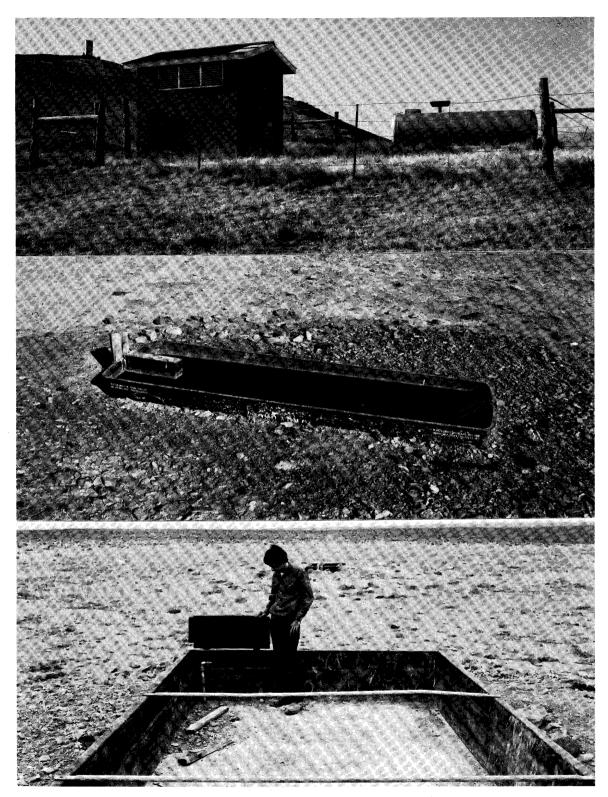
Figure 26.--A second type of water system uses a well and butane-operated pump, a metal storage tank on the hill (top), and pipeline to troughs (middle). The large shallow trough (bottom) stores water and permits cattle to escape if they fall into the trough.
