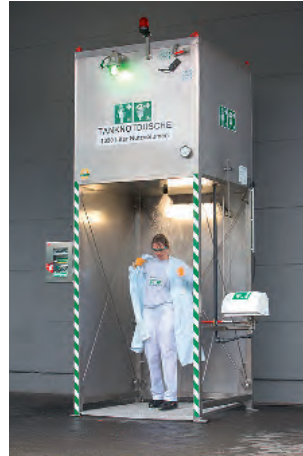
Tanknotduschen Tank safety showers
