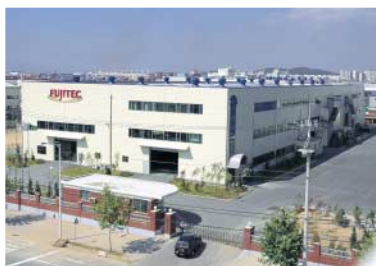
Fujitec Korea Plant
