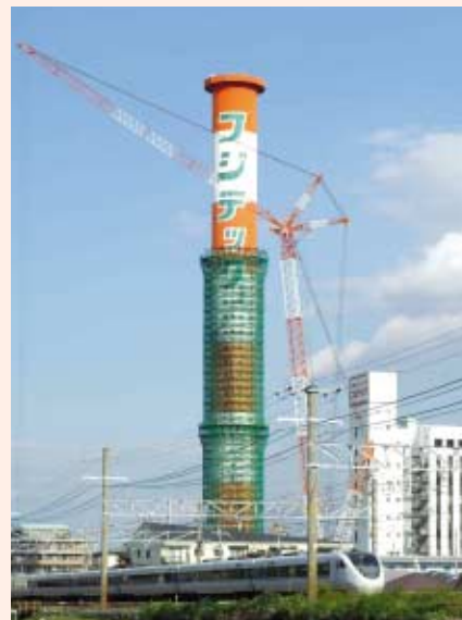
Elevator research tower currently being disassembled (Ibaraki)
