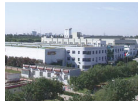
Establishment of Huasheng Fujitec Elevator Co., Ltd. (1995)
