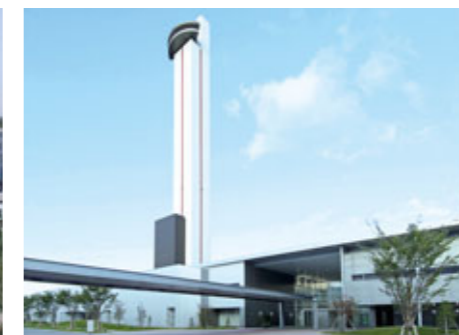
Completed construction of Head Office (Big Wing) (2006)
