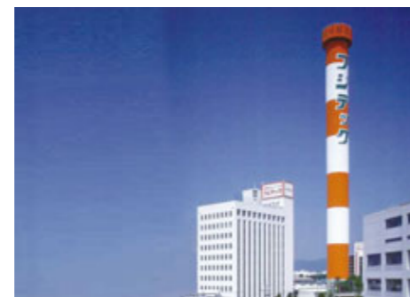
World's tallest and largest elevator research tower at that time (1975)
