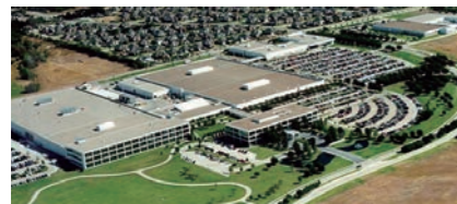
North America R&D Center (USA)
