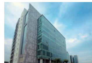
ABS Aircon Engineers Private Ltd. (India)
