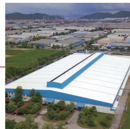
Fujitsu General (Thailand) Co., Ltd. (Thailand) Factory-2
