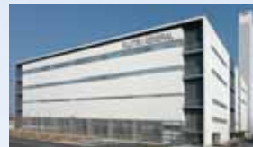
JAPAN R&D center and 198 ft. (60m) height testing tower Central R&D center for global air conditioner development. Advanced products are developed and next generation technologies are researched.
