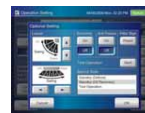
Indoor units operation monitoring
