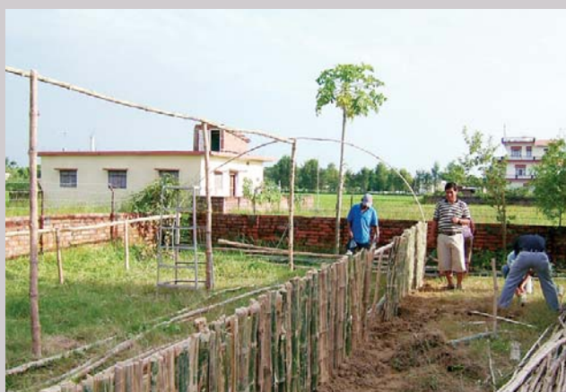
Figure 4. Growing house under construction
