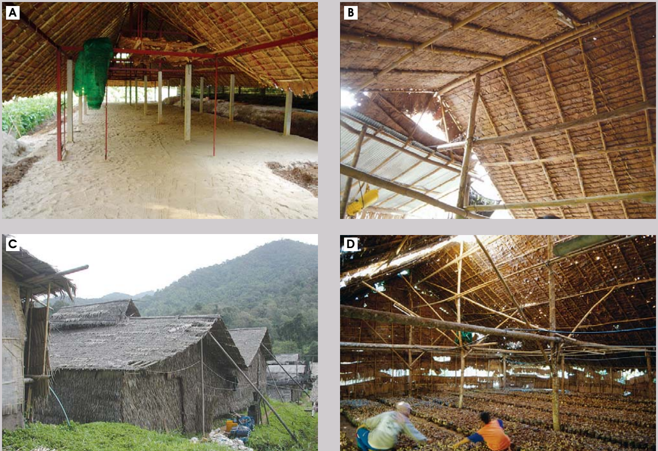
Figure 5. Recommendations for better growing houses A: Floor covered with sand B: High roof to prevent heat accumulation C: Ventilation opening on the roof D: Wall made of only local leaves
