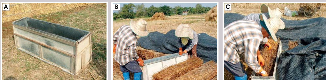
Figure 5. Making bed A: Steel bar & galvanized sheet frame B: Laying the frame C: Putting in straw
