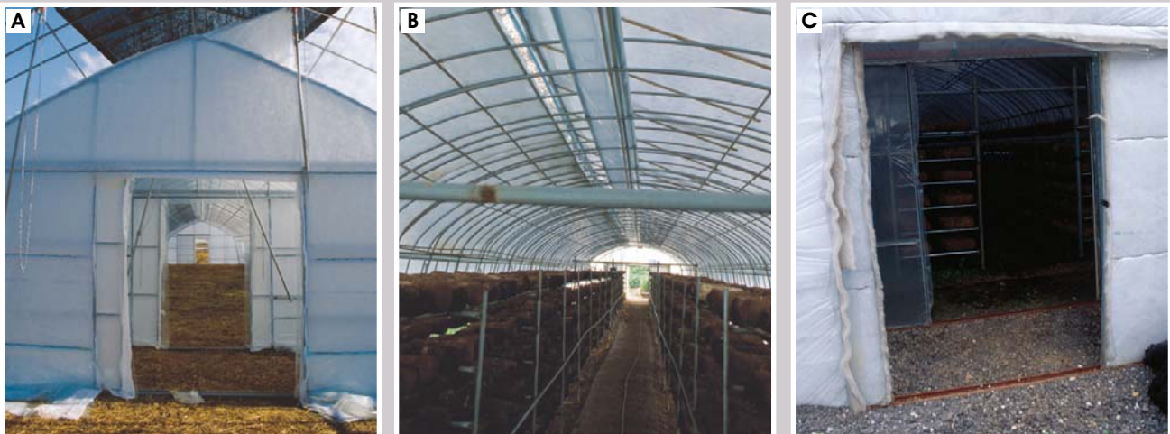
Figure 21. Growing house A: Triple structure of growing house B: The outer structure with partly open roof and the inner structure with plastic rolled up C: The outer structure made by two sheets of plastic cover and chemical cashmilon within
