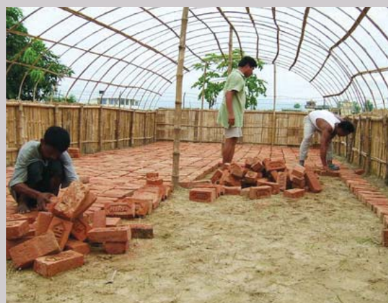
Figure 5. Floor work for growing house
