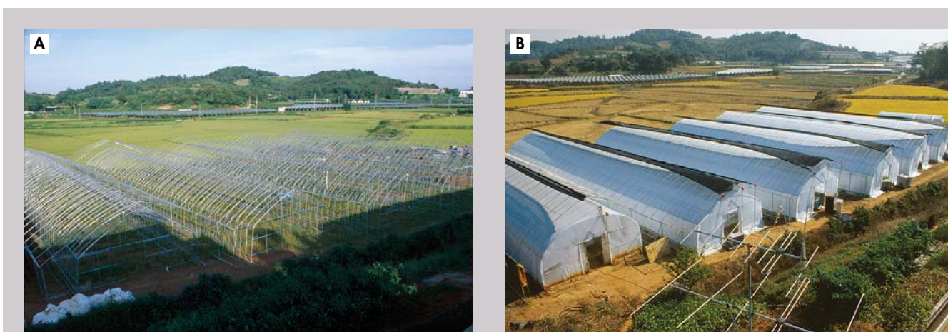
Figure 11. Growing houses with threefold structure under construction A: Completed framework B: Completed covering with plastic films and shading nets
