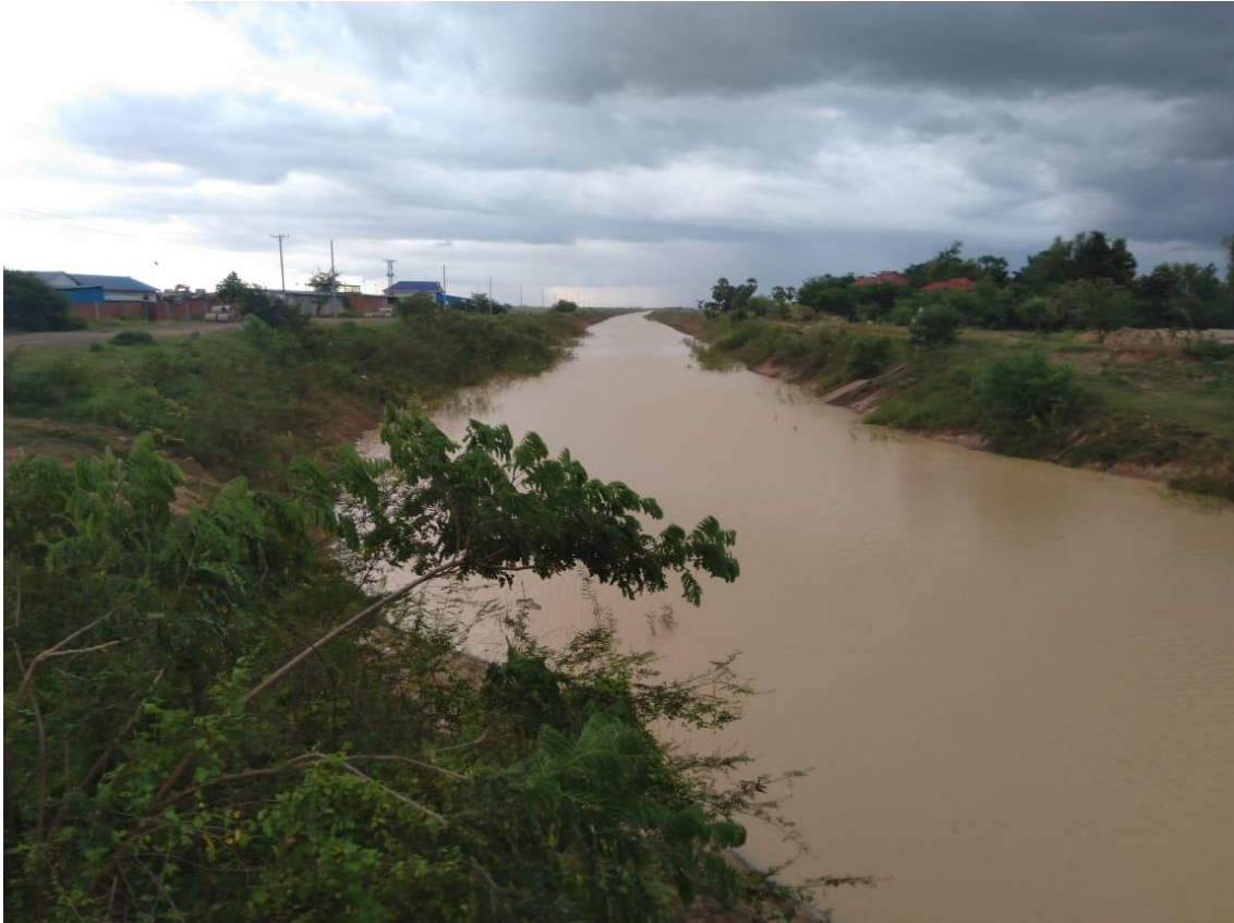
Figure 8-2. Photo of the Vaico main irrigation canals during the wet season
