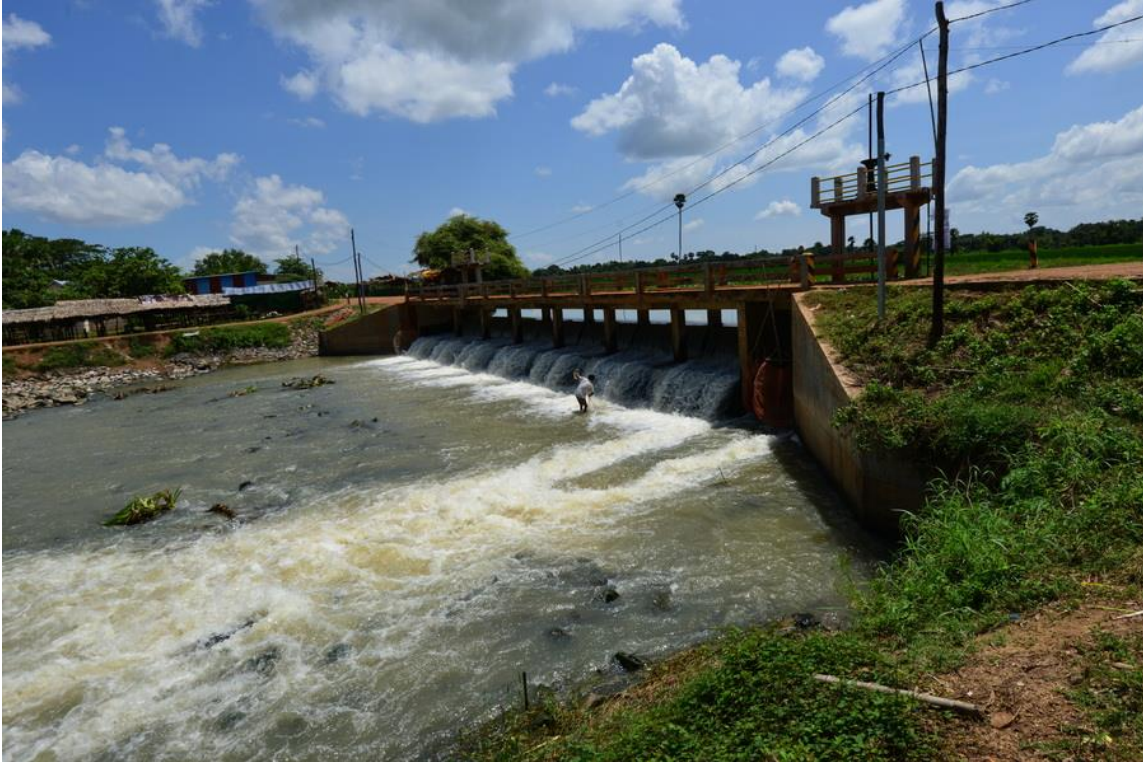
Photo 12: Tang Krasaing Dam, a typical small irrigation weir with no fish passage mitigation Fish cannot ascend the steep drop across the spillway, and cannot pass safely through the top-down water-gates.
