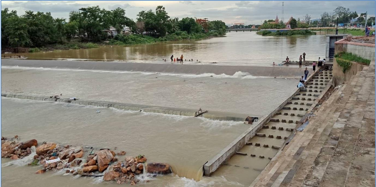
Photo 7: Cone fish-pass at Kbal Hong Irrigation Weir in Pursat in 2019 at low-moderate flow Note the lack of turbulence in the fish-pass. Unfortunately there is full access to local people who catch or disturb fish. Photo by Dr Tim Marsden, Australasian Fish Passage Services.
