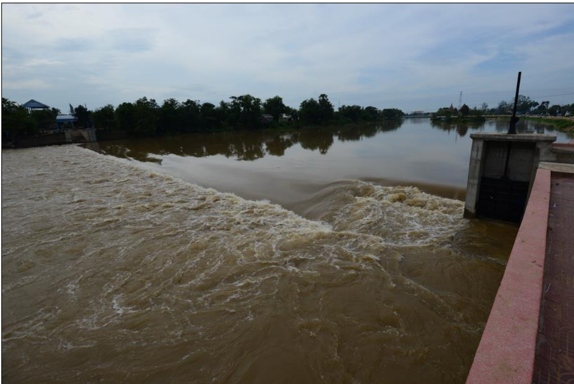
Photo 8: Kbal Hong Weir at moderate-high flows on 8-10-2019 The cone fish-pass is 'drowned out' in the right foreground next to the wall. Fish can likely pass freely under these conditions.
