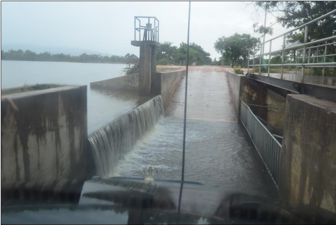
Photo 23: Damnak Kranh reservoir, new gate and spillway
