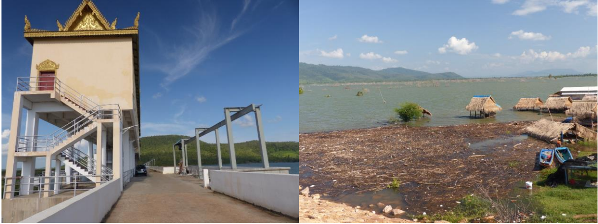
Photos 18a & 18b: Sek Sork dam, with sluice gate buildings (left); flotsam consisting of decomposing wood from remaining dead trees in background (right).
