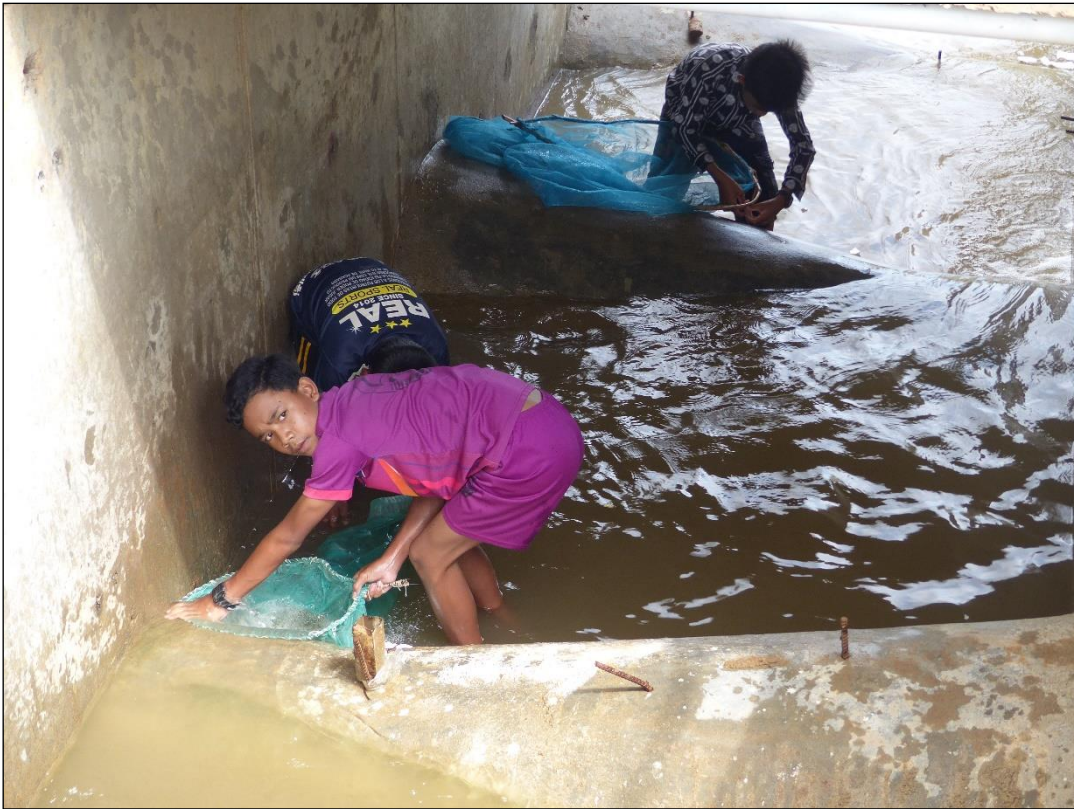
Photo 6: Ream Kon half-cone fish-pass looking downstream
