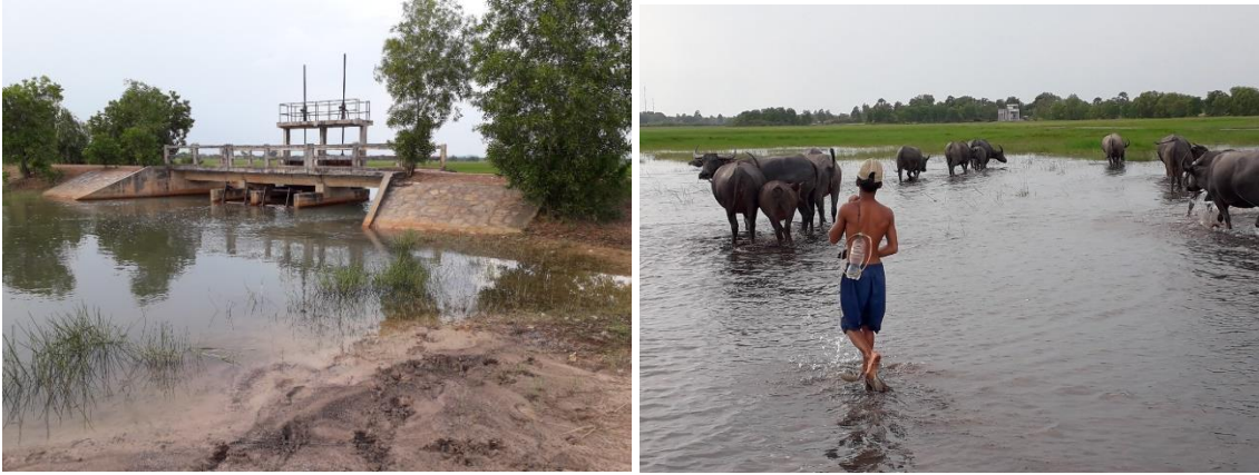
Photos 5a & 5b: larger sluice gates, with gates raised to allow freshwater enter the brackish water zone in foreground (left); buffalo grazing in brackish water zone, with visitors centre in background (right)
