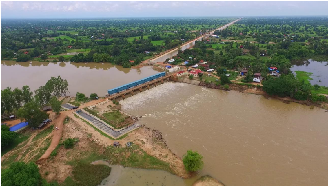
Photo 3: Damnak Ampil Dam, Pursat River The half-cone fish-pass is in the foreground, the irrigation offtake and canal are in the background.
