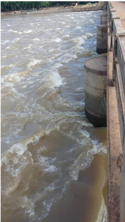
Photo 19: Charec Weir, Pursat River, moderate discharge on 8-10-19 Detail of high turbulence and fast flow downstream of the gates.
