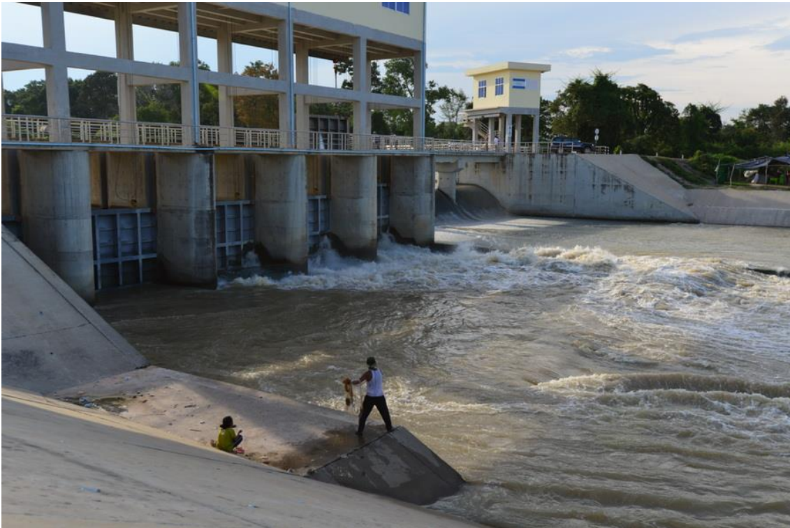
Photo 13: Achang Dam, Boribo R. There is no fish-pass at this site. Note the undershot water gates and fast shallow flow over spillway
