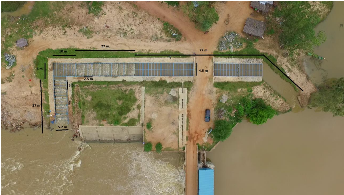
Photo 4: Half-cone fish-pass at Damnak Ampil Weir, Pursat River Plan view from drone video on 8 October 2019. Flow is from right to left. Note the high turbulence in the pools and the length of the inlet section.
