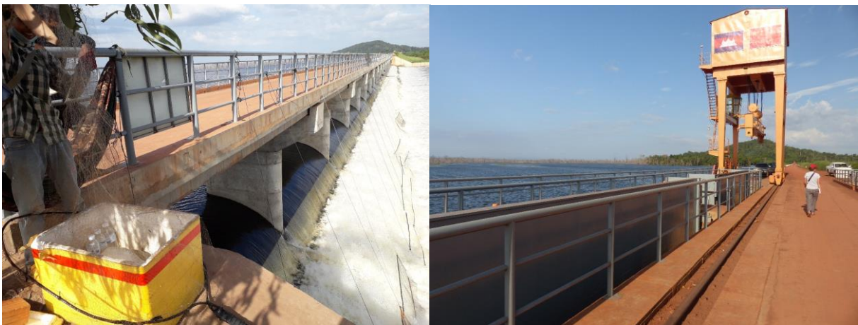
Photos 10a & 10b: dam spillway with many nets suspended (left); sluice gates at the far end (right)
