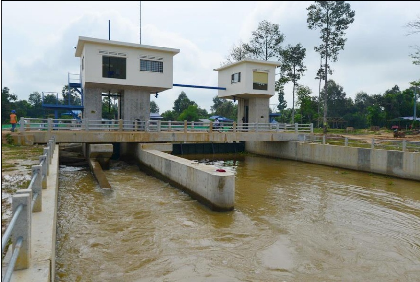
Photo 2: Wat Chre dam looking upstream Fish-pass is on the left of the photo
