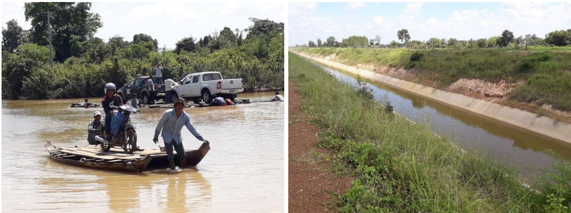
Photos 8a & 8b: makeshift ferry crossing on route from ATT to Stung Sreng I (left); link canal is located 8-10m below surface at part of route with low hills (right)
