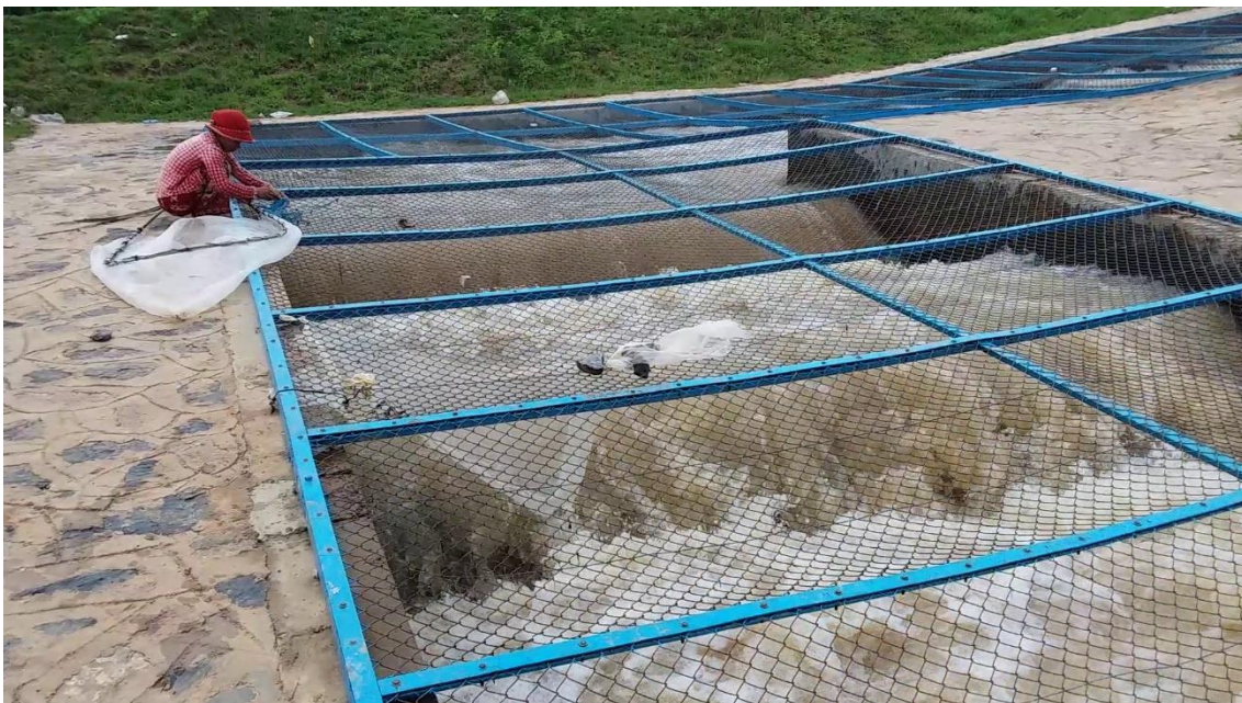
Photo 5: High turbulence and fast flow in the lower section of Damnak Ampil fish-pass on 8-10-19
