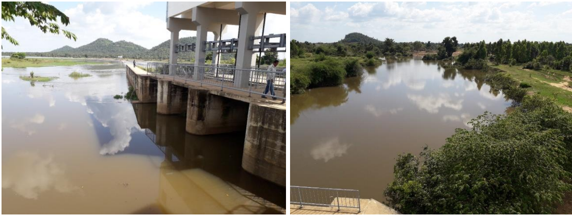
Photos 9a & 9b: headworks with sluice gates for release into river, plus spillway in background (left); Stung Sreng river (not in flood) just downstream of headworks (right)
