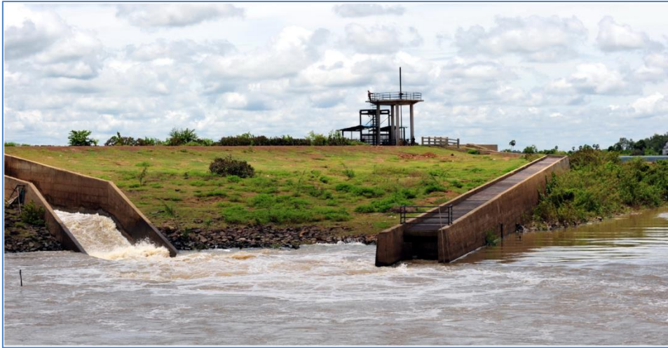
Figure 16: Stung Chinit Weir in Cambodia, downstream of the main dam wall
