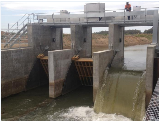
Figure 20: Overshot "lay-flat" water gates which can pass debris and pass fish safely
