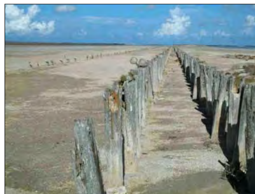
Old Railroad pilings at Bahia Grande.
