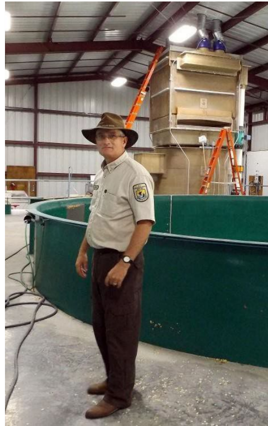
Figure 18: Hatchery Manager Craig Eaton in front of the gas equilibration tower (tan) under construction as part of the RAS system at the former Hagerman NFH.
