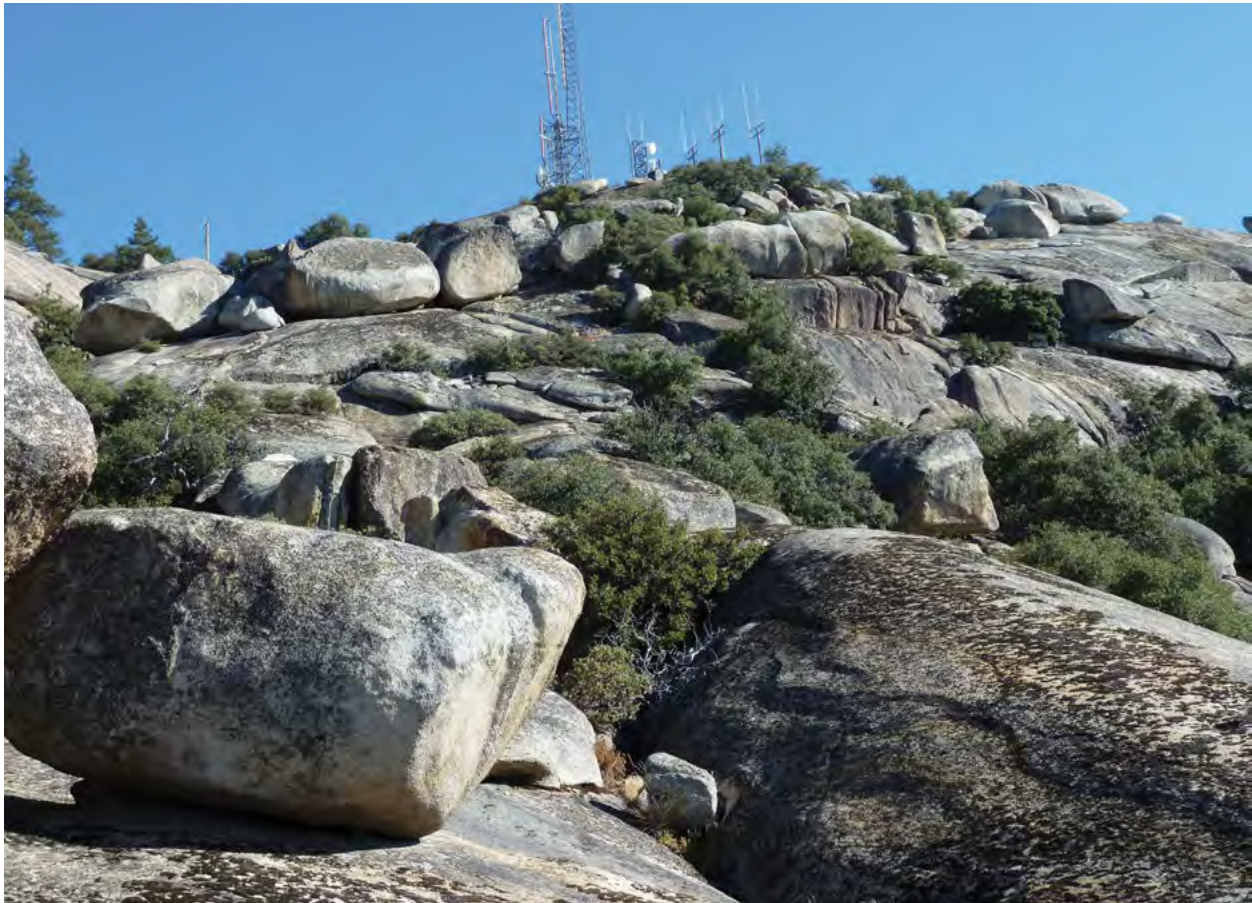
Communication towers at Blue Ridge NWR. Photo: USFWS
