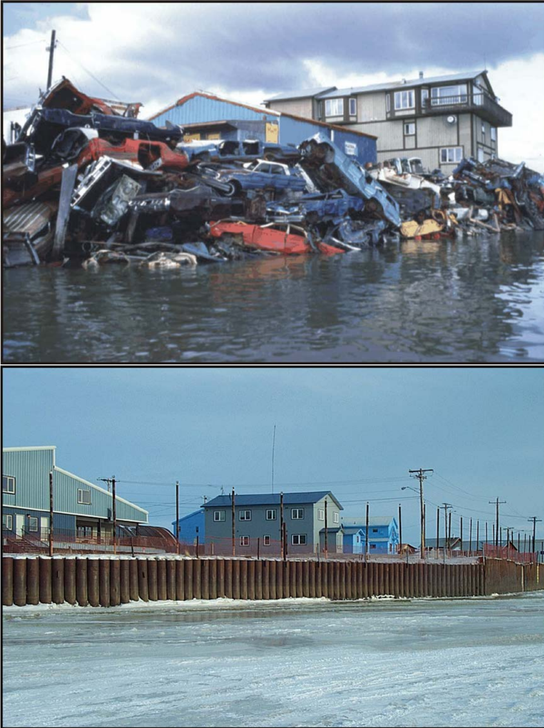
Figure 89. Historical bank stabilization efforts with old cars, waste barrels, and other debris piled over the banks on the Bethel waterfront (top image; photo by J. Barker). Similar situations can be encountered at smaller scales in many rural communities along the Yukon and Kuskokwim River drainages. By contrast, the modern waterfront in Bethel is more effective at preventing erosion and more ecologically sound (bottom image; photo by S.J. Miller, USFWS).
