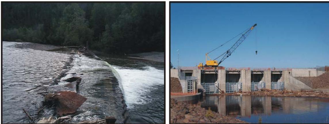
Figure 20. Two dams within the Tanana River drainage. The Chatanika River dam was constructed in 1925 to divert water from the Chatanika River into the Davidson Ditch, a 134 km (83 mile) canal that provided water to mining operations near Fairbanks (Spence 1996). It was later used to produce electricity and was eventually removed from the river in 2002. This photograph of the remnant dam (on left), courtesy of E. Mayer, USFWS, was taken shortly before removal. The Chena River flood control dam (right) was constructed in 1979 to divert water from the Chena River towards the Tanana River during times of exceptionally high flows and prevent flooding in the community of Fairbanks (Rozell 2003). This image, courtesy of M. Osborne, USFWS, is of driftwood removal at the dam shortly after a flood event.
