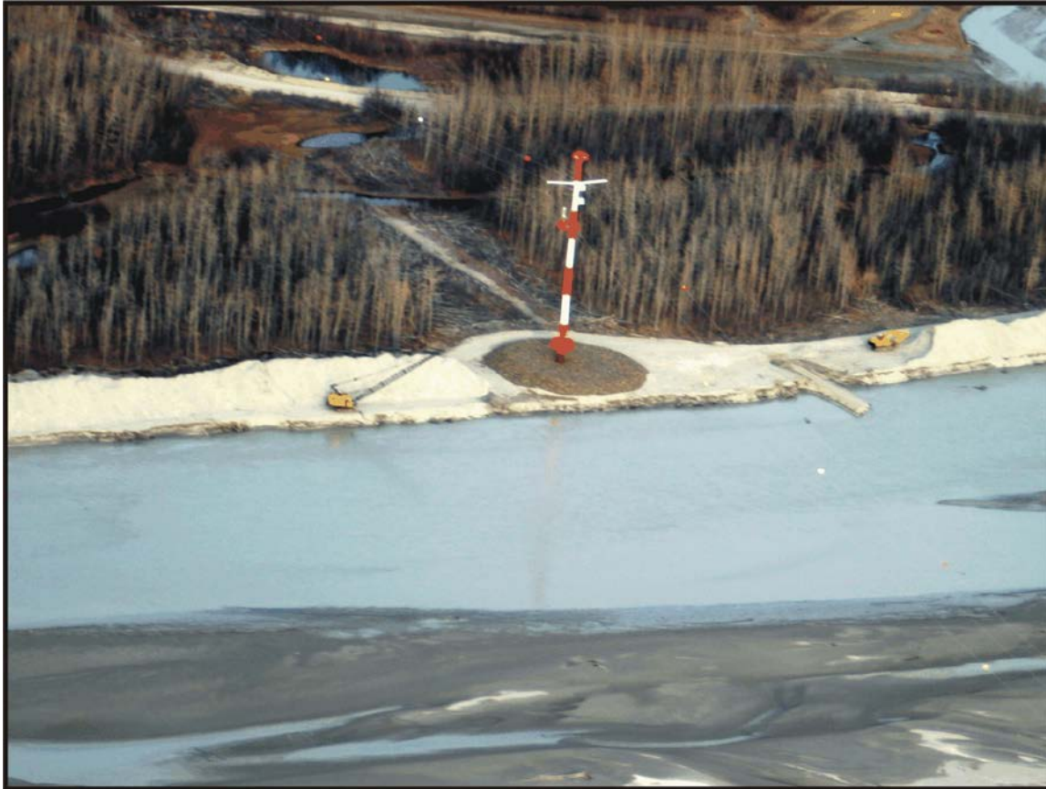
Figure 15. Streambed gravel mining with dragline dredges is a common practice in the Yukon and Kuskokwim River drainages. The bucket is slung into the River with the crane and drawn back to the shore full of gravel scraped from the river bottom. This image is of a gravel mining operation in the Tanana River drainage near Fairbanks. Photo by R.J. Brown, USFWS.
