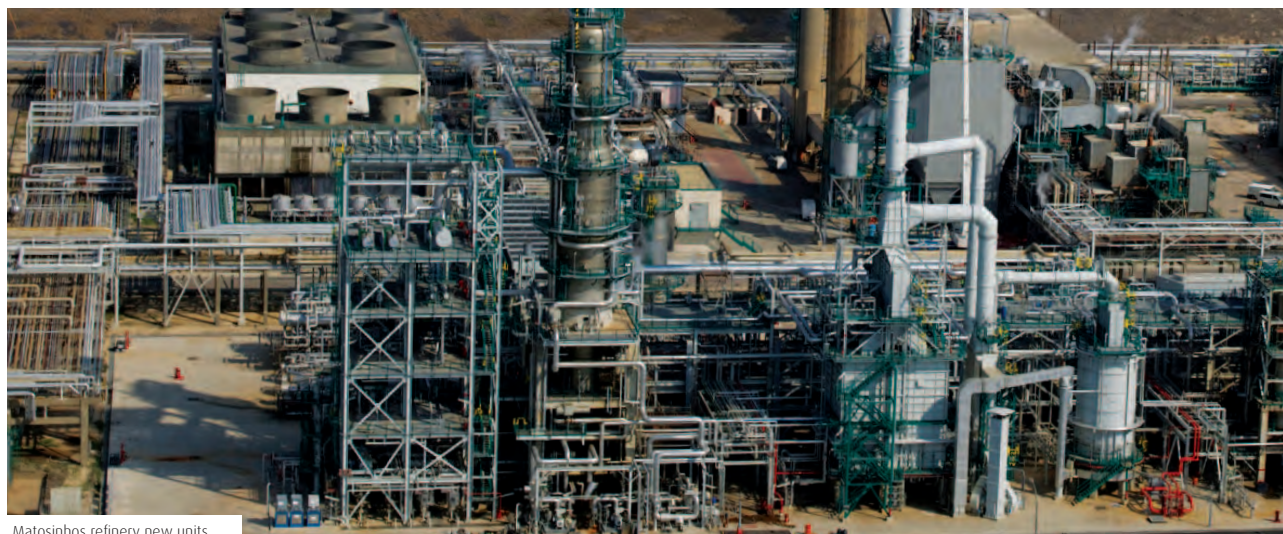
Matosinhos refinery new units
