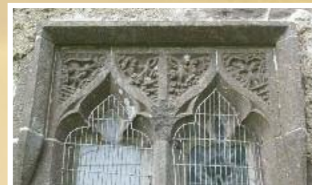
Figure 23 A double light ogee headed window in the chancel of Clonfert Cathedral.
