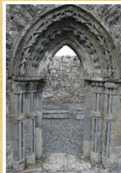
Figure 20 Transitional doorway with undercut chevron and animal heads at Drumacoo.
