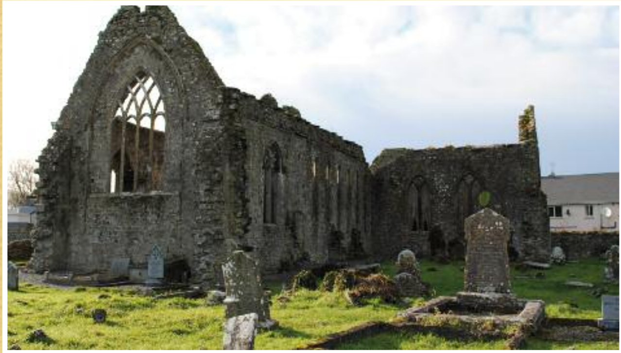
Figure 24 Athenry Dominican priory, the first phase of which was built in 1241. The large window with switch line tracery in the east gable is of fifteenth-century date while the tall lancets in the south wall are of late thirteenth early fourteenth-century date.
