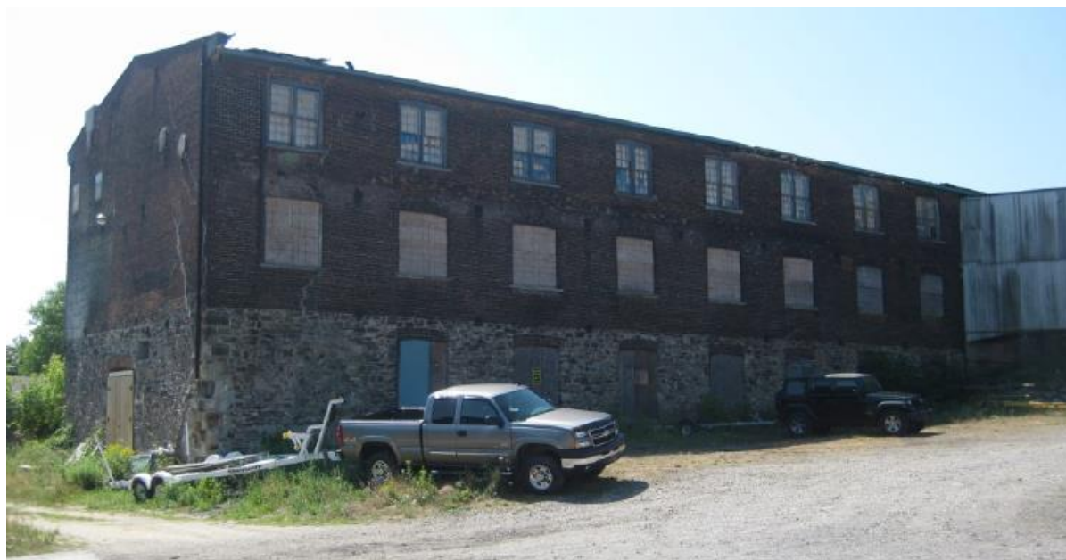
Figure 10: 185 Mill Street Brick Building viewed from the northeast, north elevation on the right and east elevation on the left, with the raised, sheet-metal clad link on the far right (source, "185 Mill Street and 15 Clarence Street," Heritage Impact Statement, March 2014, p. 6).
