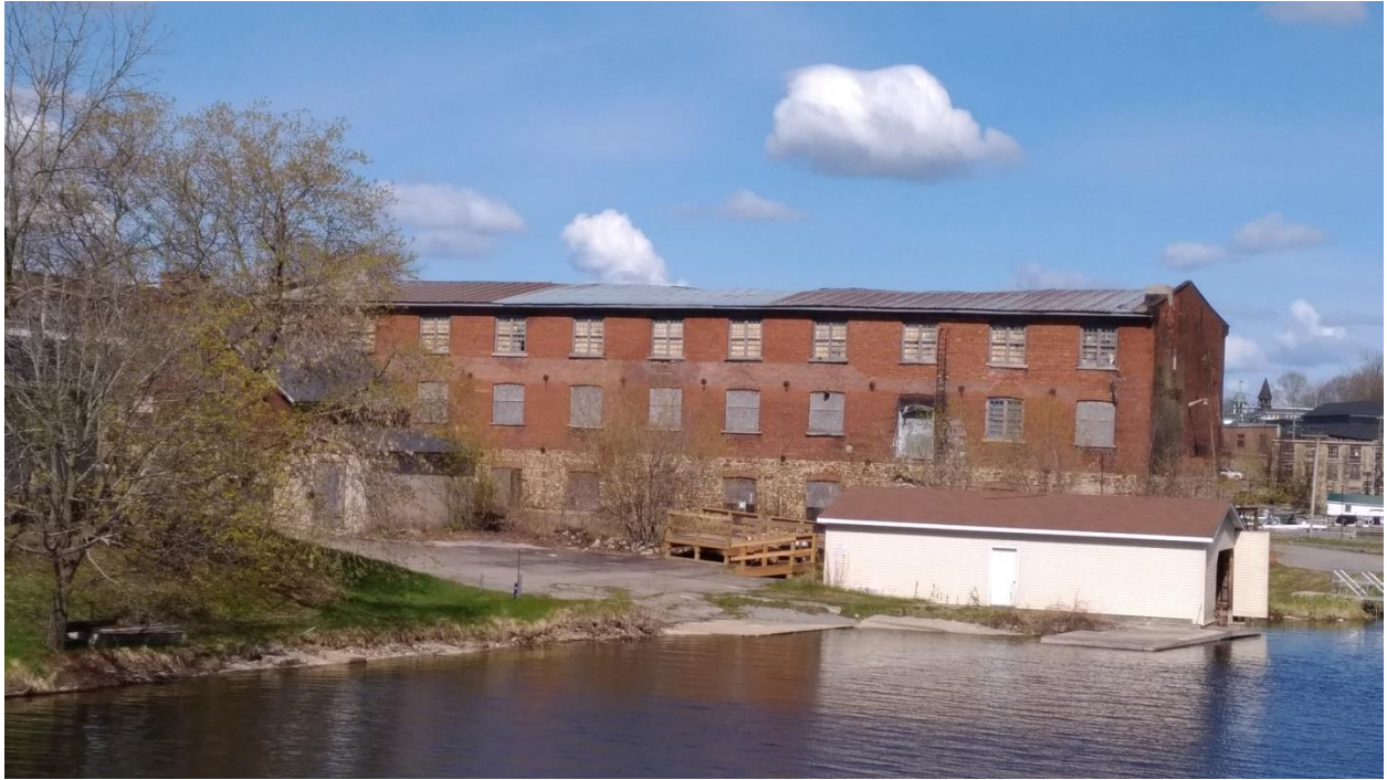
Figure 12: Brick Building, 185 Mill Street, viewed from the southeast (E. Tumak, May 2020).
