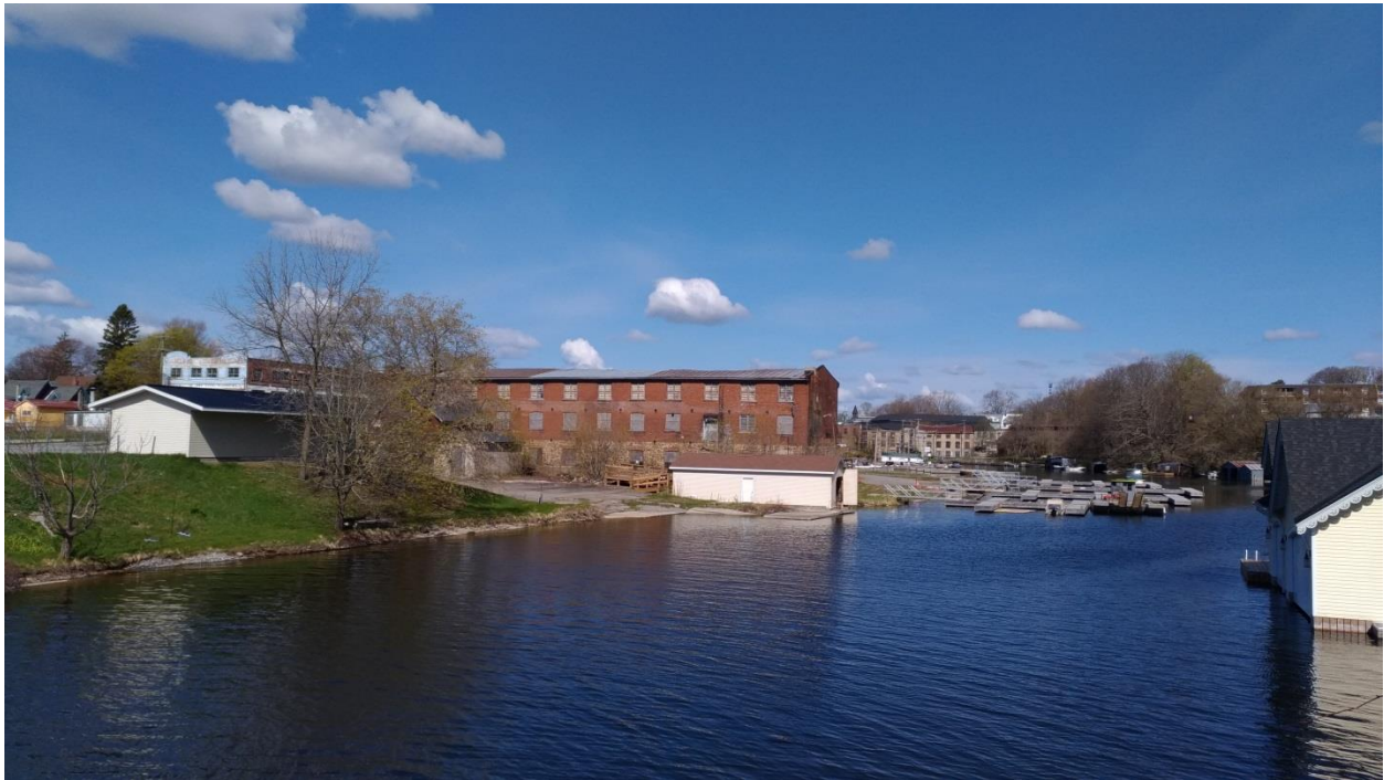
Figure 39: 185 Mill Street viewed from the southeast from the Swing Bridge (E. Tumak, May 2020).
