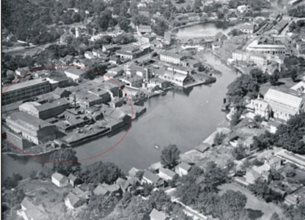
Figure 29: Aerial view from the southeast, 1920, showing 185 Mill Street in the lower left circled in red. The Brick Building is in the far left centre and the Stone Building to its immediate right/north, with the three-storey former Parmenter & Bulloch/Textron Building immediately to the west/left. In this image there are structures to the immediate east/right, north, and west/left of both the Stone and Brick Buildings (LAC, PA-30656).
