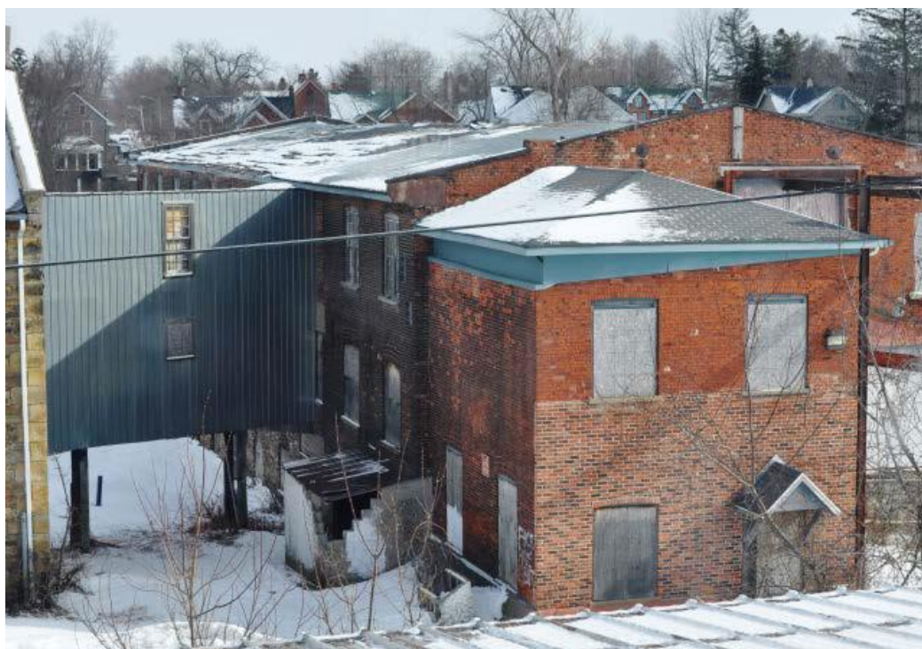
Figure 9: View from the east, showing the sheet-metal clad link between the Stone and Brick Buildings, ca. 1951 (source, "185 Mill Street and 15 Clarence Street," Heritage Impact Statement, March 2014, Appendix A, p. 48).
