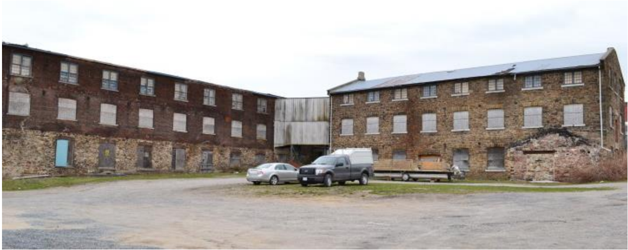
Figure 6: 185 Mill Street, viewed from the northeast, prior to renovation interventions, with the Stone Building on the right/north and the Brick Building on the left/south (source, Mark Thompson Brandt Architect and Associates, Peer Review: Heritage Impact Statement, “Mill St. & Clarence St. Development, ‘Riverstone,’ Gananoque, ON,” 2014).
