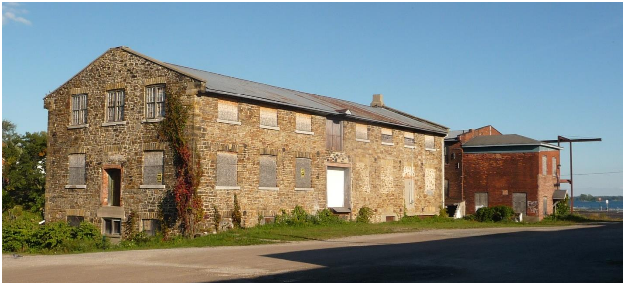
Figure 5: 185 Mill Street, viewed from the northwest prior to recent renovations showing more traditional opening arrangements, but with a combination of temporary closures and areas filled in with stone (E. Tumak, Oct. 2013).
