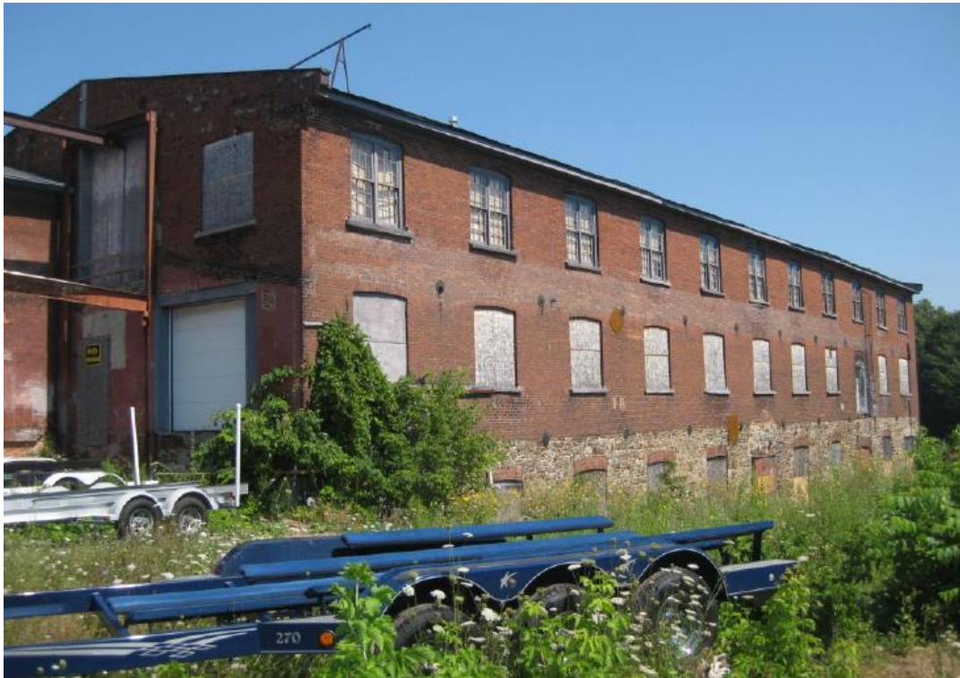
Figure 7: 185 Mill Street Brick Building viewed from the southwest, south elevation on the right and west elevation on the left (source, “185 Mill Street and 15 Clarence Street,” Heritage Impact Statement, March 2014, Appendix A, p.23).
