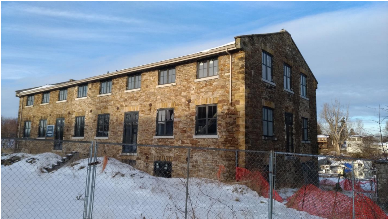
Figure 4: 185 Mill Street, Stone Building, viewed from the southwest after recent renovation interventions affecting the fenestration and entrances (E. Tumak, Jan. 2020).
