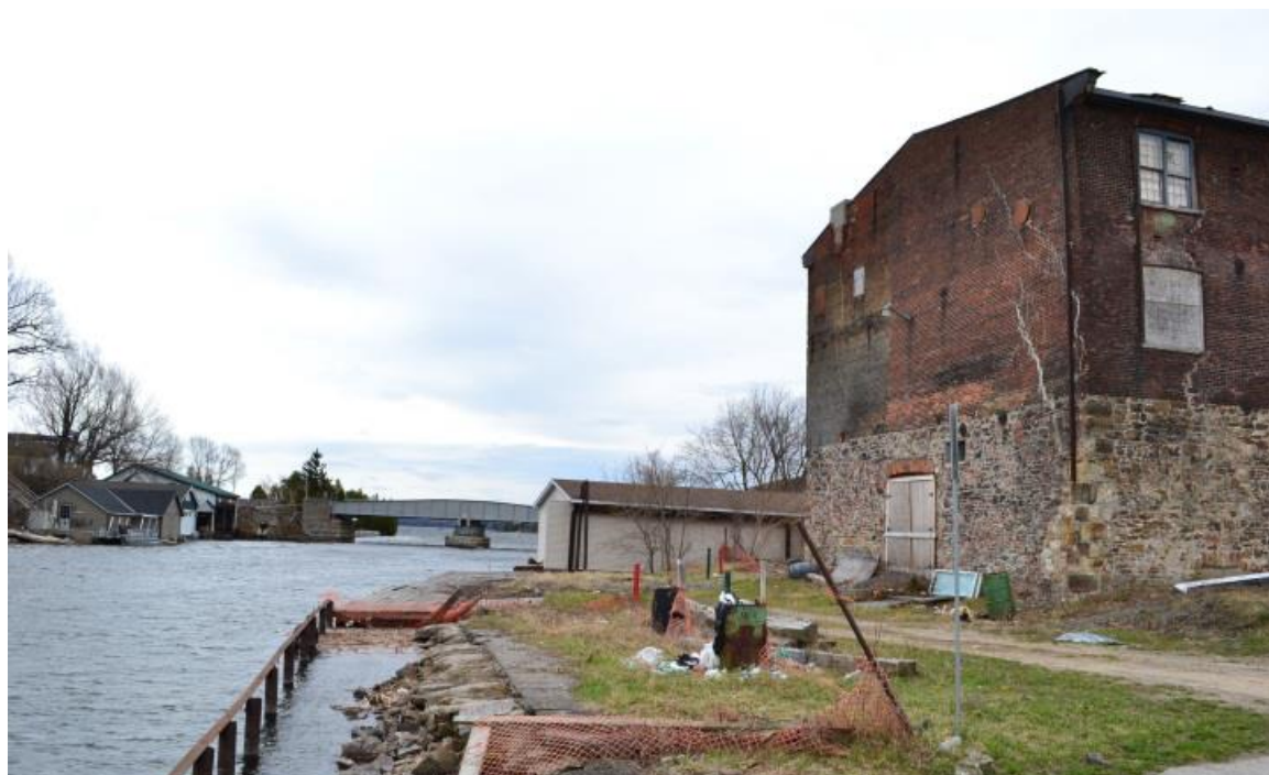
Figure 11: Brick Building, 185 Mill Street, waterfront/east elevation, showing the caps for interior metal tie rods between the main and upper levels on the west/left and north/right elevations (source, Peer Review: Heritage Impact Assessment, 2014, p. 3.)
