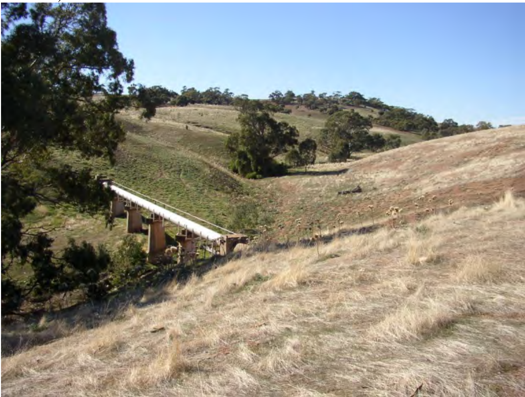
Photo B2: Main watercourse on site, eastern reach, looking east.
