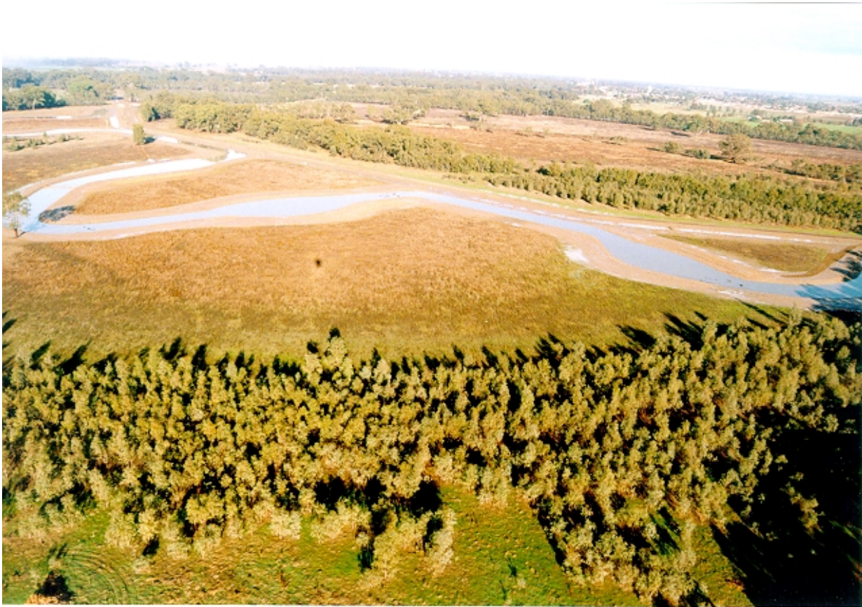
Figure 5: Meandering flow path of the Muckatah Surface Water Management Scheme as it passes through Kinnairds Wetland. The design of this section of drain incorporates constructed wetlands, siltation sumps and more natural aesthetics (Photo: G-MW 1999; view looking south-west).
