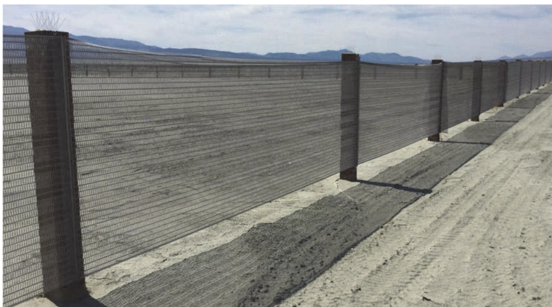
FIGURE 4-13 Sand fence at Owens Lake.
