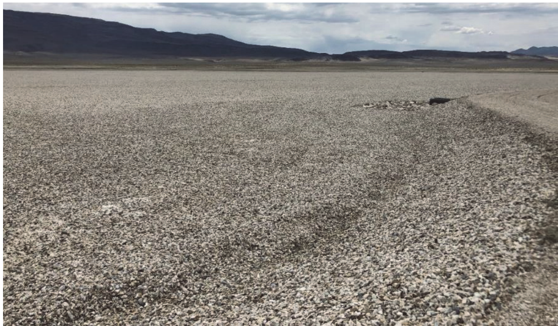
FIGURE 4-9 Dust control using the gravel BACM.
