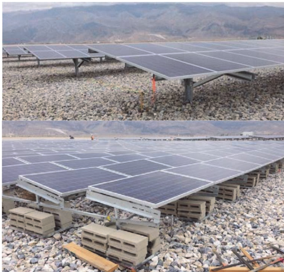
FIGURE 4-14 Solar panel testing installed on gravel at Owens Lake using pile-driven mounts (top) and squat ballast mounts (bottom). SOURCE: Schaaf, 2019.
