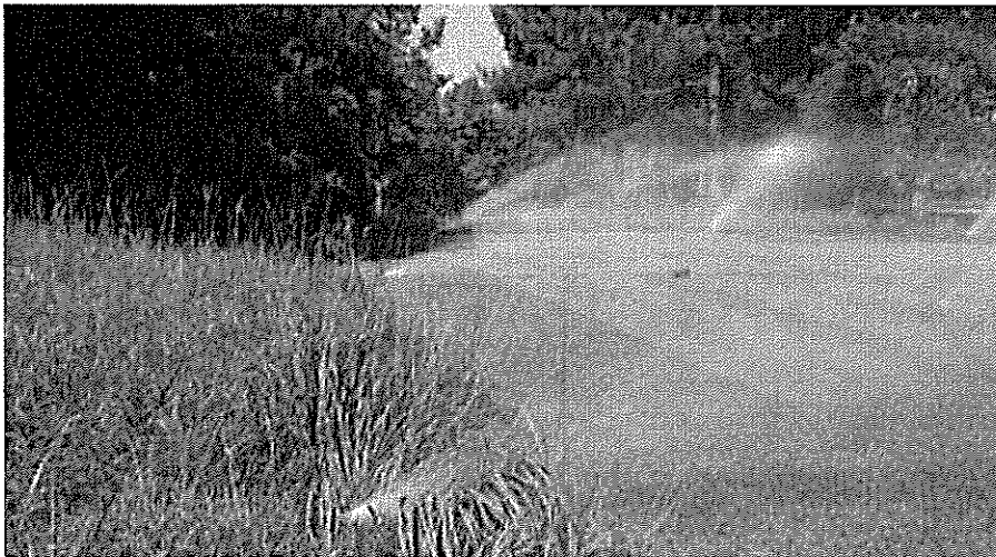
Turf can grow over sprinklers and disrupt irrigation coverage, especially in rough and naturalized areas. Check and trim turf around sprinklers every month.
