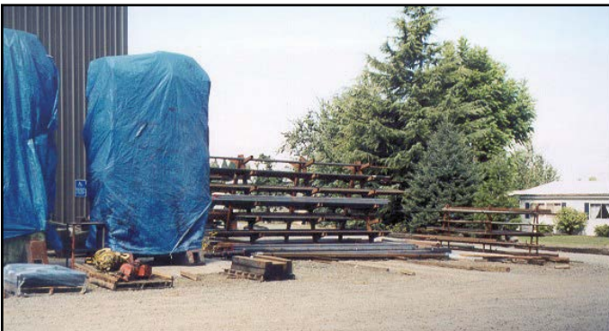
Figure 2b Wastes due to inefficient storage of raw materials.
