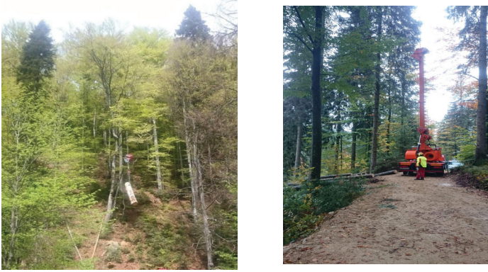
Figure 12. Using skylines in primer transport
