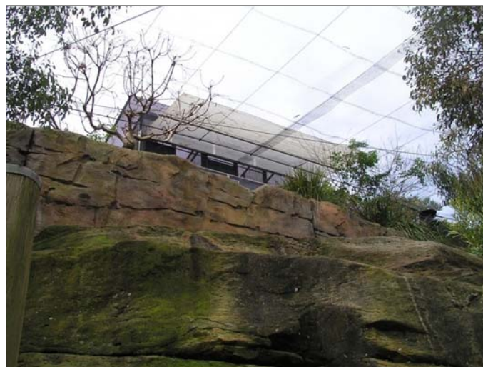
Figure 4.6: Aviary structure of top part of enclosure, showing upper feeding station structure Wollemi Exhibit Taronga Zoo. Photograph L Fragar
