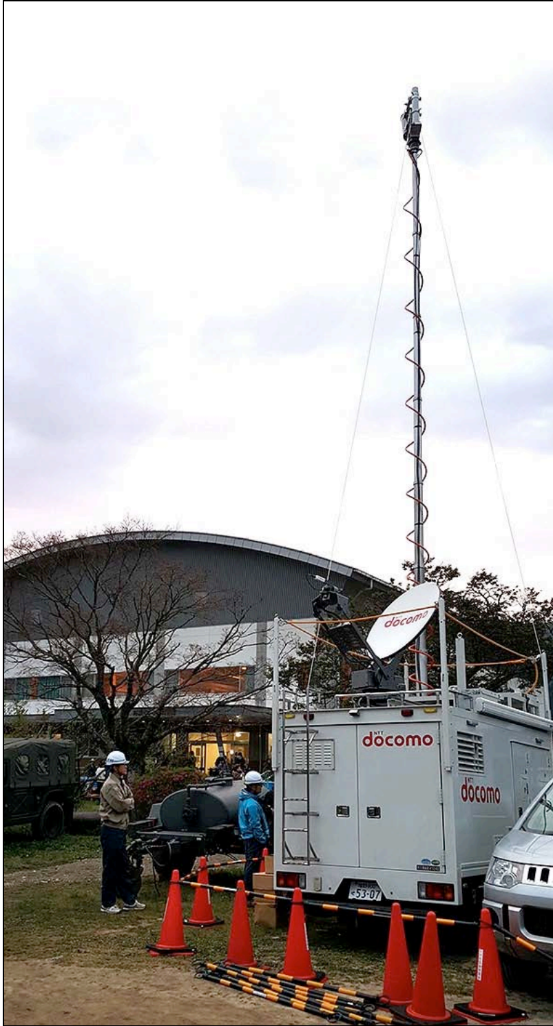
Figure 4-14. DoCoMo satellite truck outside of the Aso City Gymnastic Hall providing transmission link for damaged underground cable at cell sites
