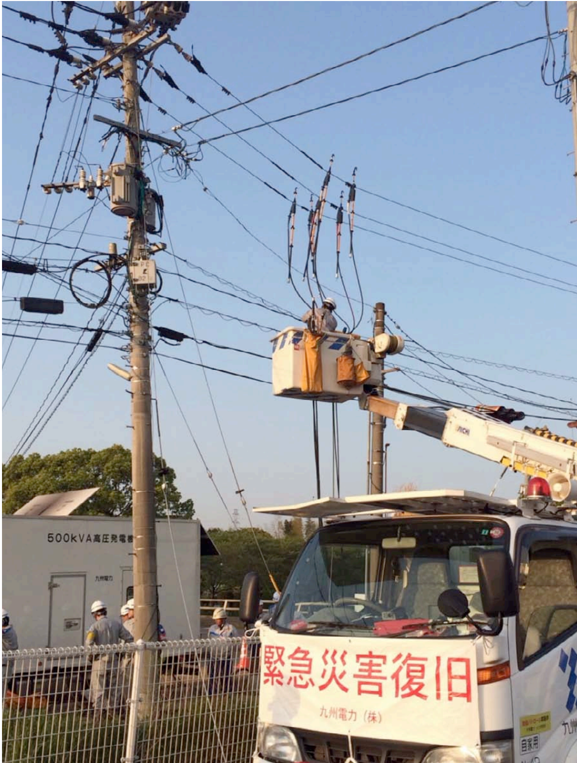
Figure 3-58. Hooking up an Emergency Generator to a Distribution Primary
