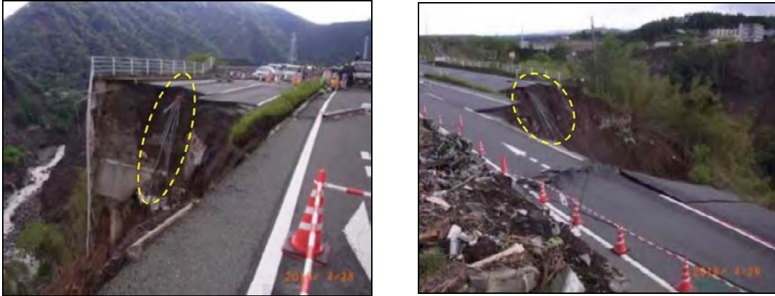
Figure 4-6. The two ends of the buried optical fiber cable bundles were severed by landslide ( 32.885^{\circ}\text{N} , 130.9866^{\circ}\text{E} ). The distance was about 500 meters. (Courtesy: MLIT Kyushu)
