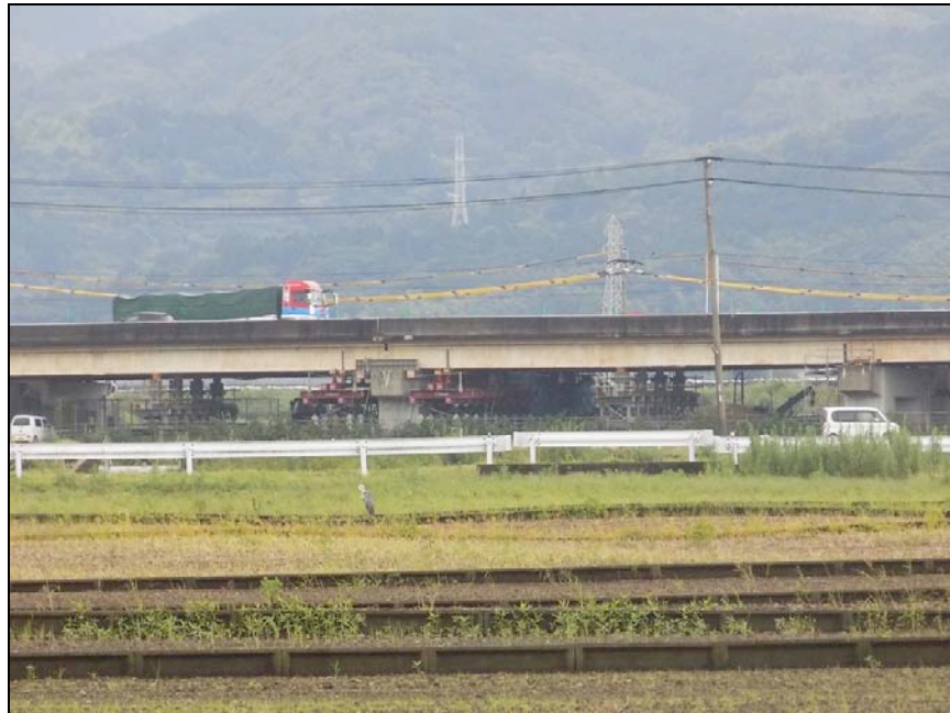
Figure 9-15. Some brace supports were needed to raised the deck to repair the bearings (Tang)
