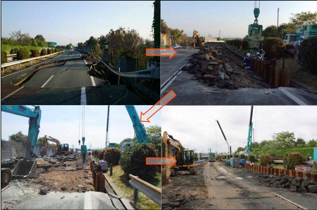
Figure 9-12. Repairs in progress
