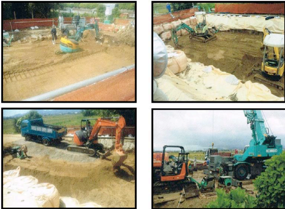
Figure 5-22. Completing Repair of 1350 mm Steel Pipe
