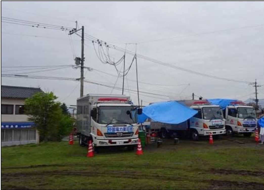
Figure 1-3. High power generating truck provided power to circuits that were disconnected from power source (MLIT)
