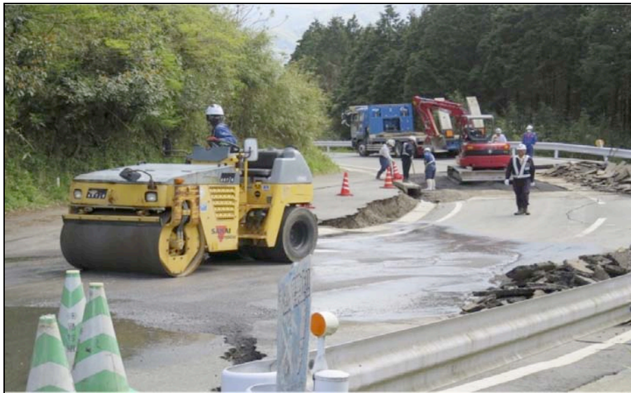
Figure 9-96. Prefecture Route 149 damage repairing in progress
