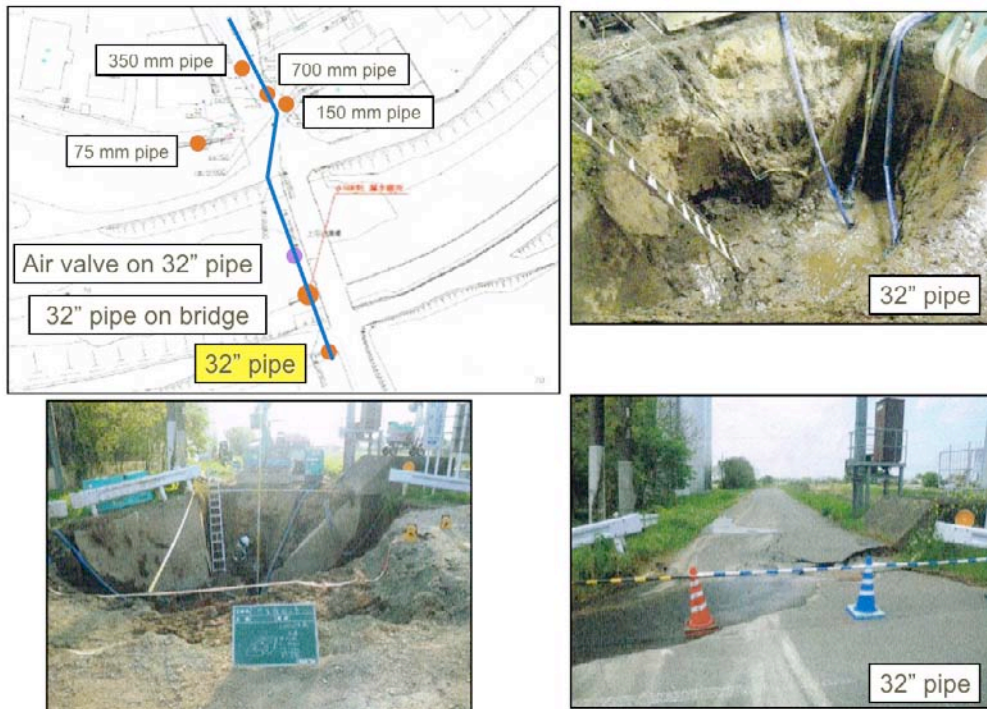
Figure 5-25. Repair of 800-mm steel pipe south of the bridge
