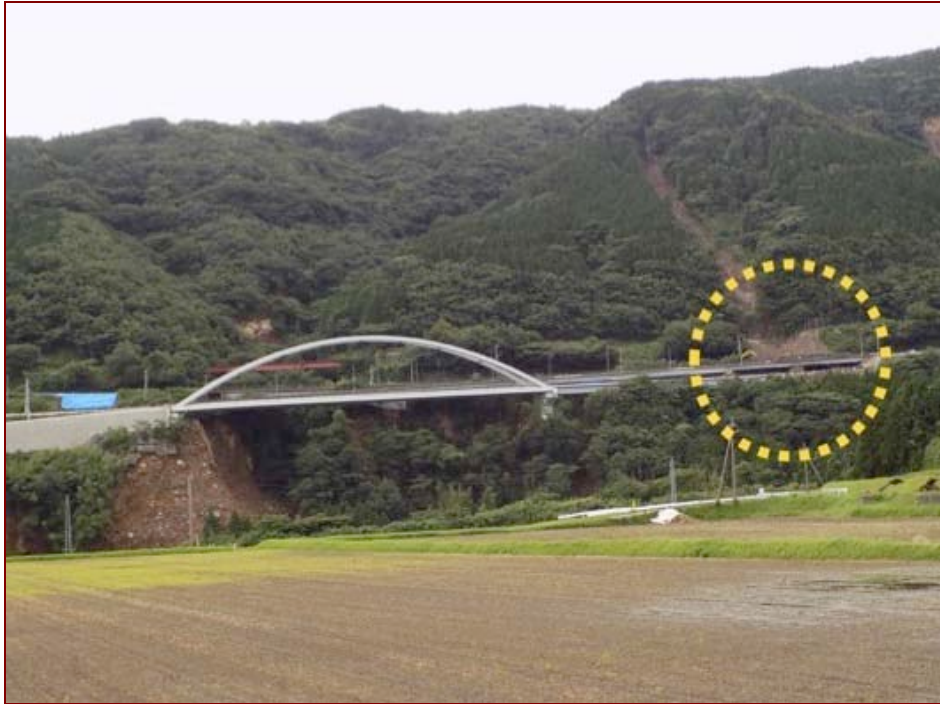
Figure 9-89. Heavy rainfalls initiated this landslide that covered the tracks. (N32.87685° E130.94996°)
