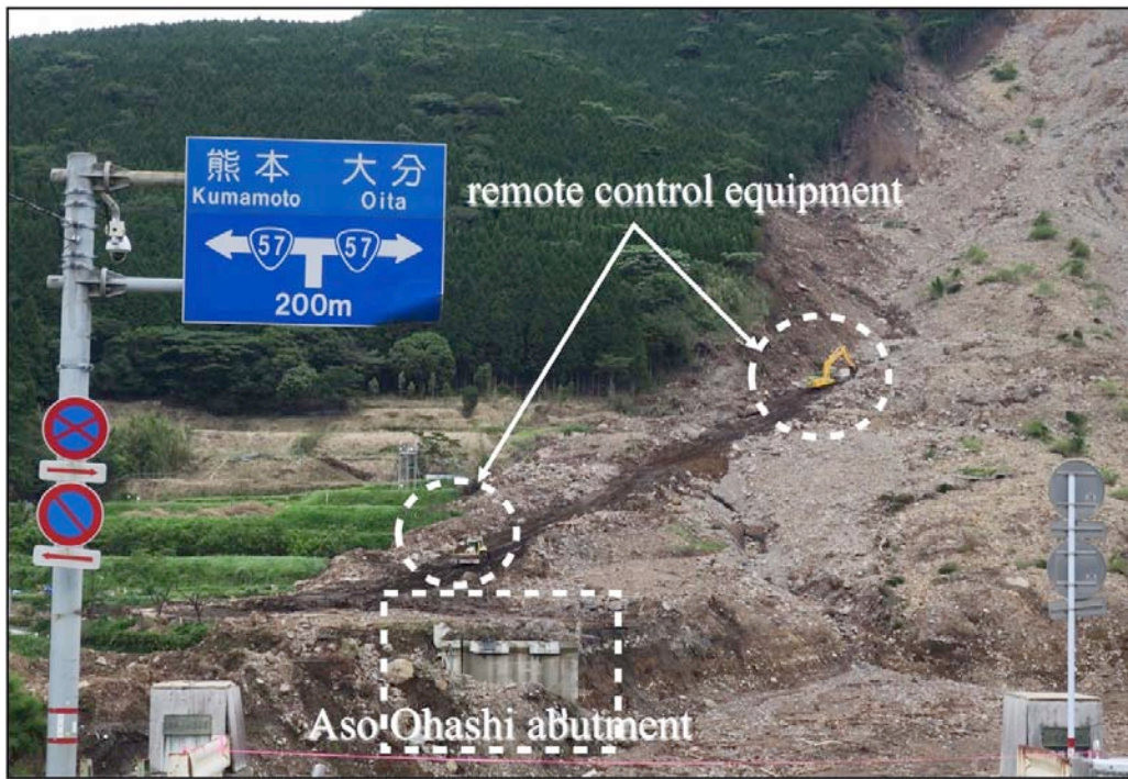
Figure 9-30. Remote controlled bulldozers were used to remove landslide material (Tang)
