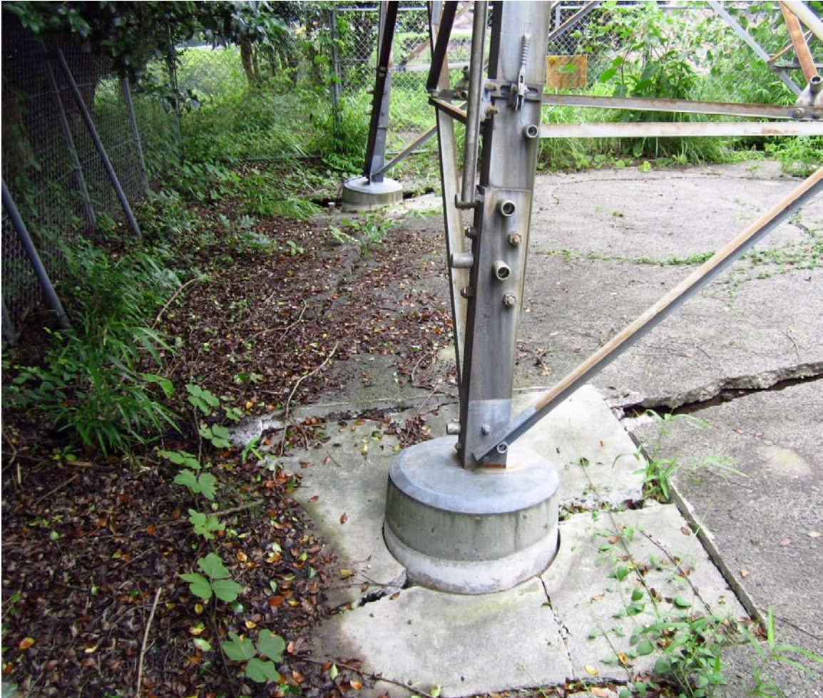
Figure 3-13. Old Tower 8 Foundation
