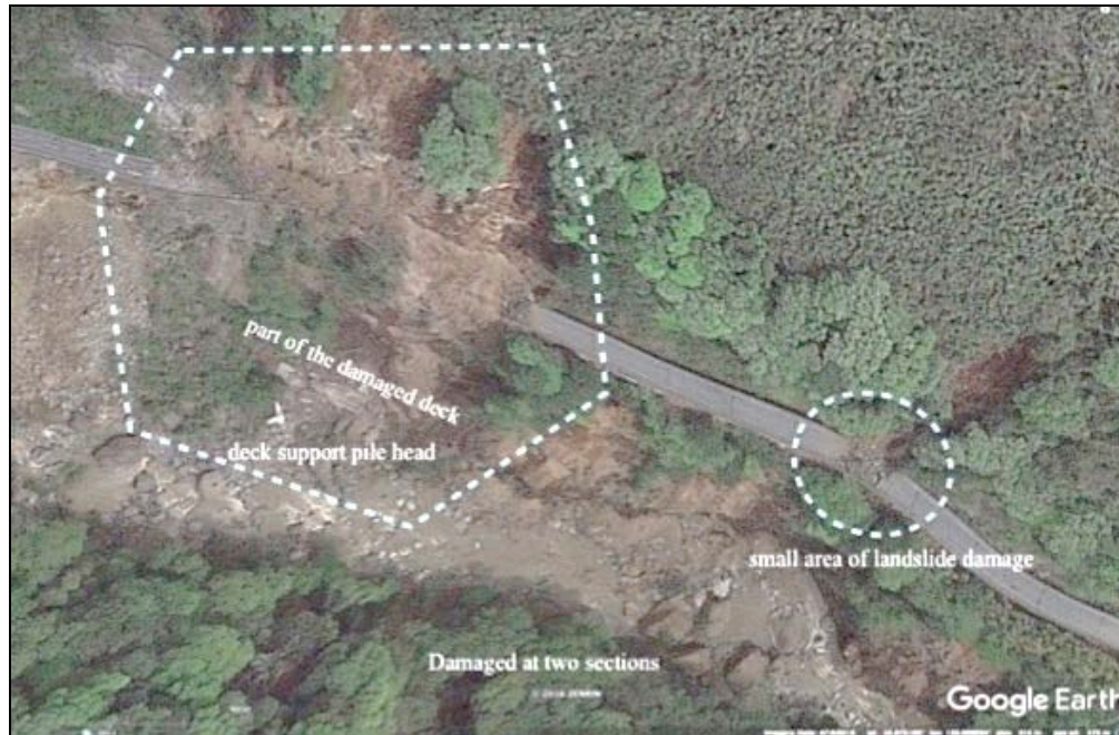
Figure 9-51. The bridge damage on the left hand side was about 60 m. The damage of the deck was small on the right hand side. (Source: Google Earth)
