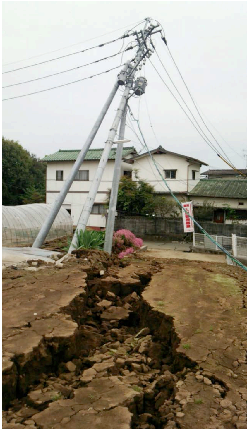
Figure 3-52. Distribution Pole Exposed to Surface Faulting
