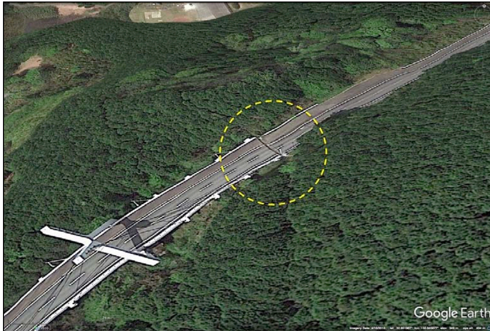
Figure 9-38. The circled area shows the abutment failure. (Source: Google Earth)
