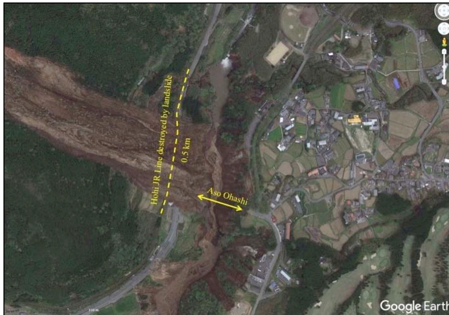
Figure 1-7. Hoho JR Line destroyed by landslide
