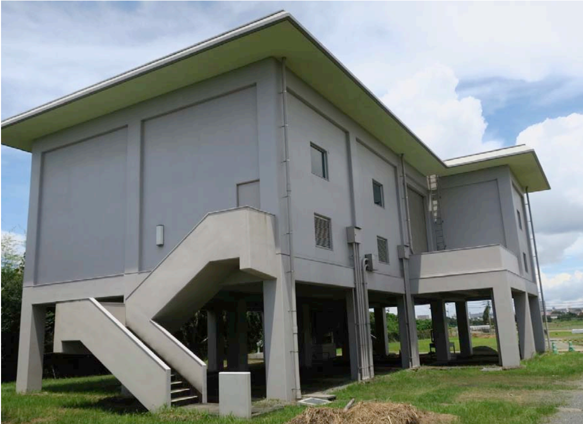
Figure 5-34. Pump Station Building
