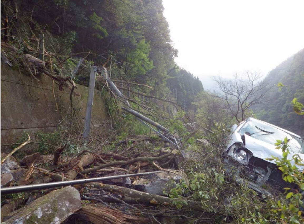
Figure 3-57. Distribution Pole Collapse
