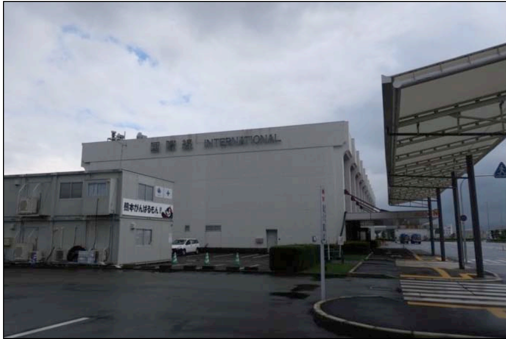
Figure 7-13. Exterior of the International Terminal
