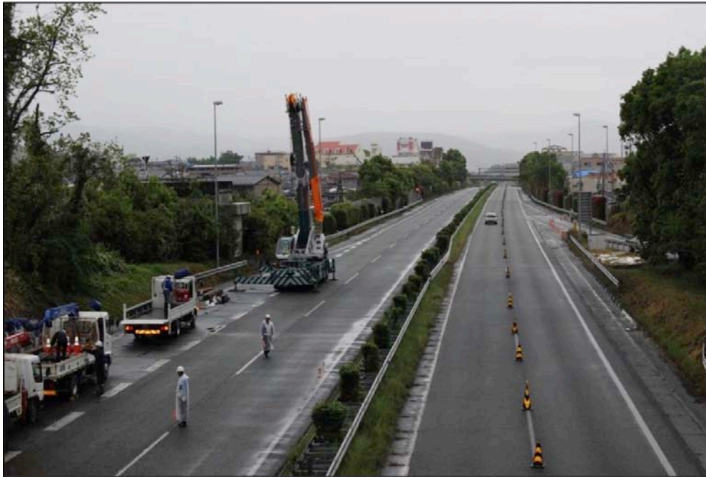
Figure 9-8. Road surface being prepared for reopening after the bridge removal
