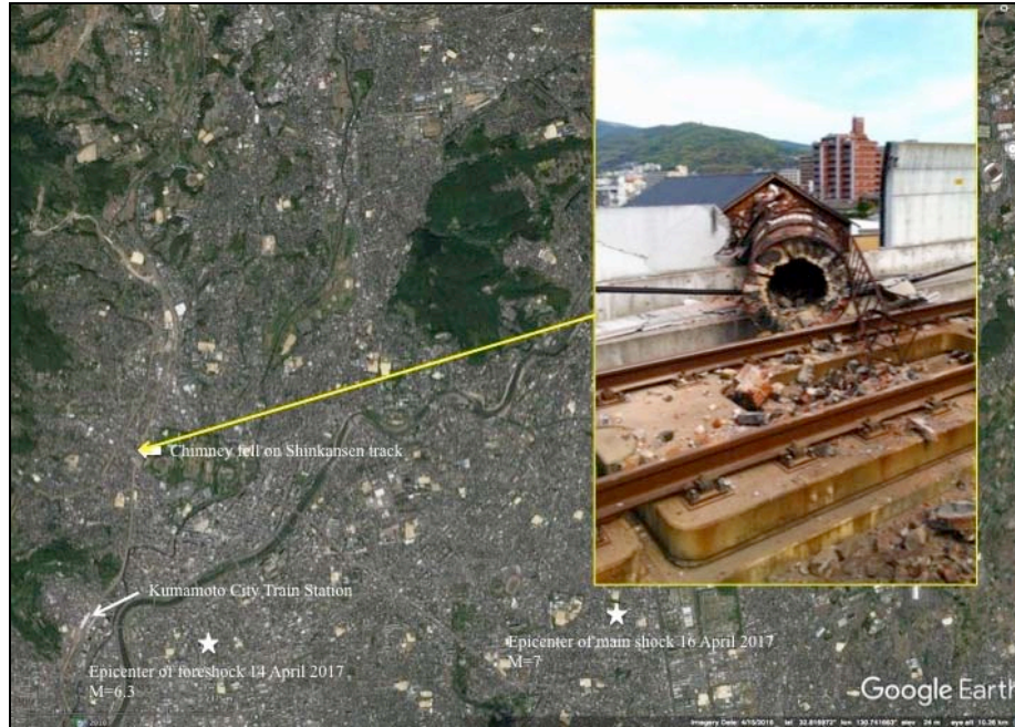
Figure 9-78. The chimney broke apart after falling on the raised track. Luckily it did not damage the rails; only the sound barrier was damaged. (Source: Google Earth and Fukuoka MLIT)
