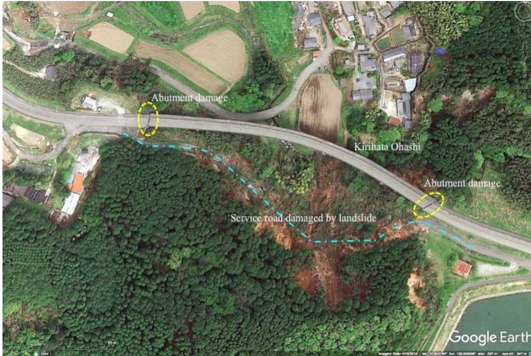
Figure 9-33. The circled areas were the damages observed. The blue color dashed line indicates the bypass road covered by landslide (Source: Google Earth)
