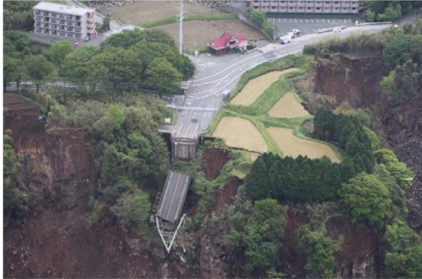
Figure 9-27. The east side of the Aso Bridge after the main shock on 16 April
