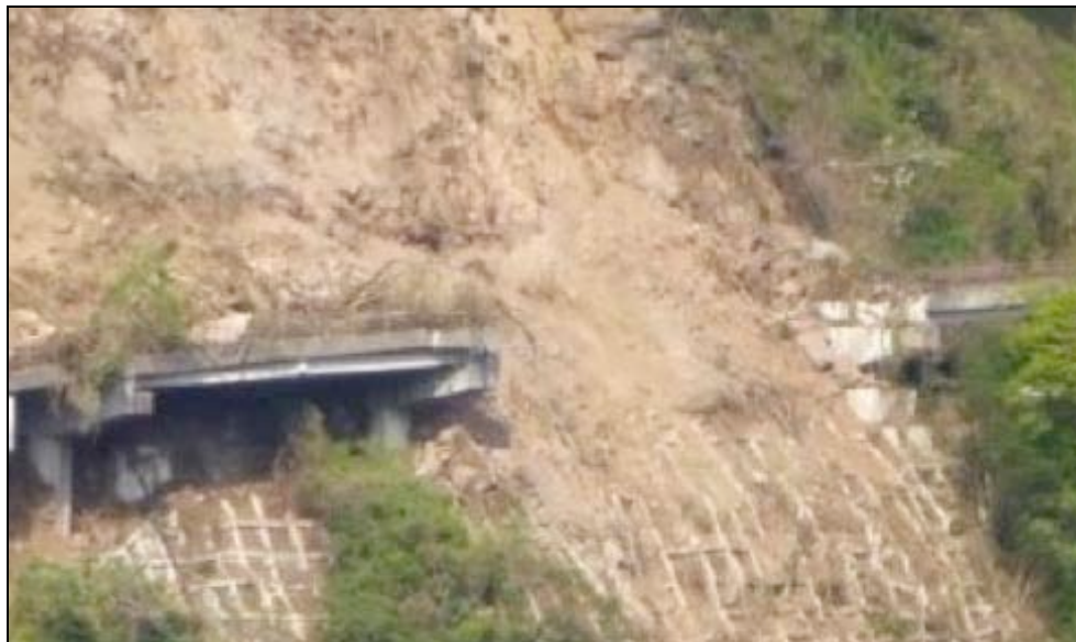
Figure 9-53. A close up view of the landslide
