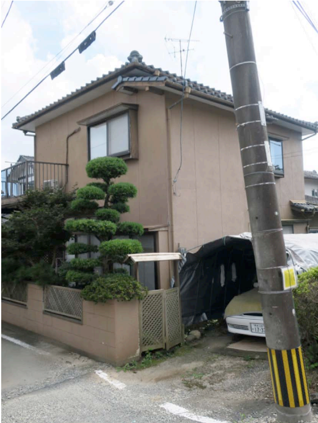
Figure 2-38. Tilted Power Pole
