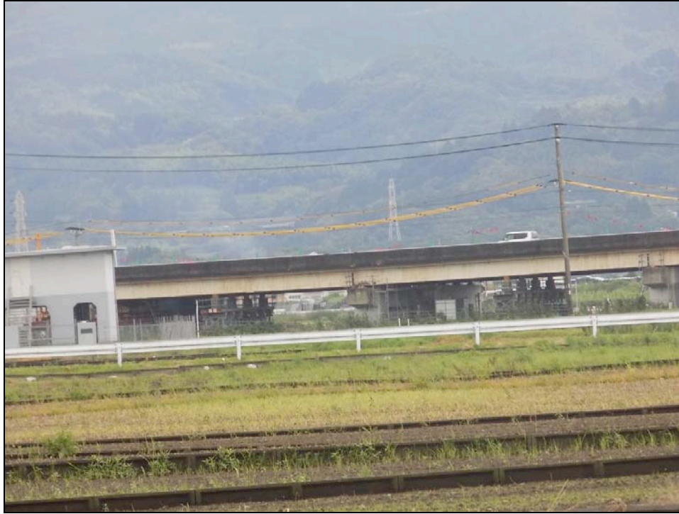
Figure 9-14. Additional shoring to support the bridge deck (Tang)
