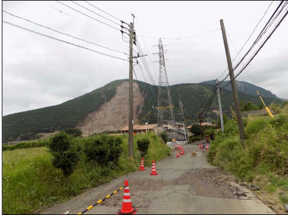
Figure 9-60. Slight road surface damaged. In the background is the major landslide described in Section 2. (Tang)
