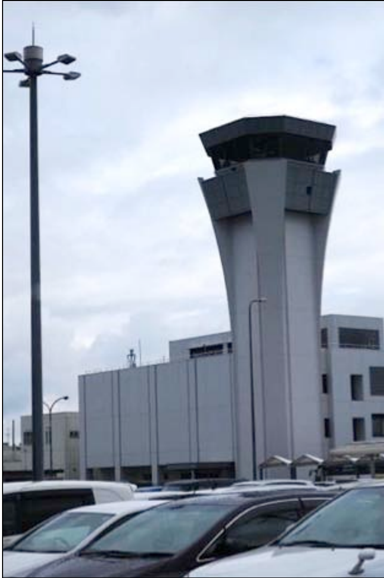
Figure 7-16. Exterior view of the Kumamoto Airport Control Tower.
