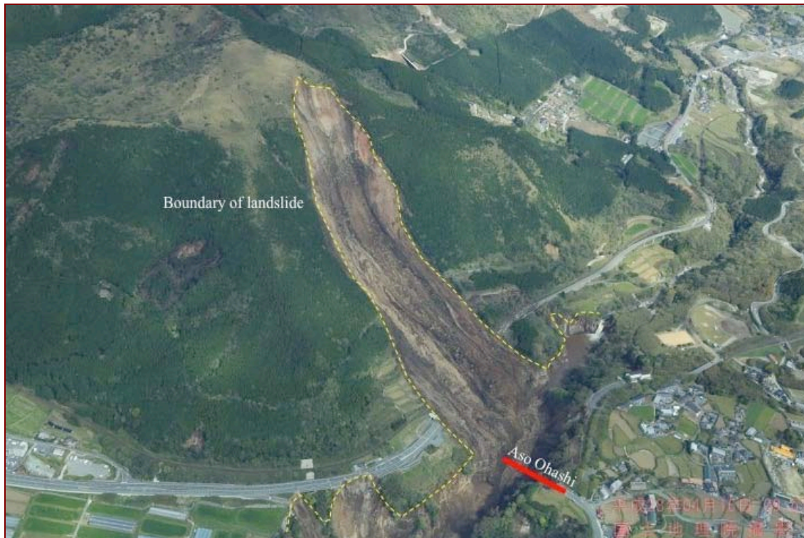
Figure 9-3. Aerial view of the landslide that caused the collapse of Aso Bridge (Source: Geospatial Information of Japan)
