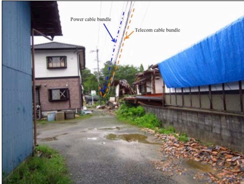
Figure 4-5. In Mashiki town these aerial cables (power and telecom) dropped almost to the ground and they were touching one another at the lowest point ( 32.7888^{\circ}N , 130.8205^{\circ}E ).
