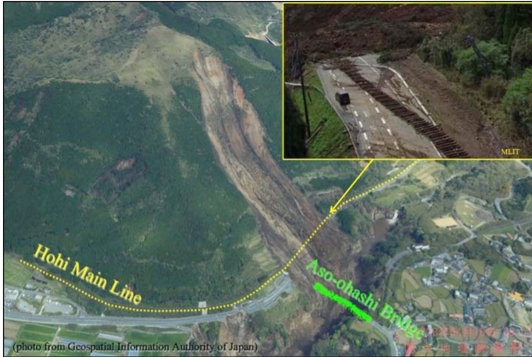
Figure 9-88. This is the great landslide site, the signature failure of this earthquake. A long section of the Hohi Main Line was damaged and covered under tons of mud and rocks. The insert shows the dislocation of the train tracks to route 57 below it, caused by the landslide. (N32.88387°, N130.98705°)
