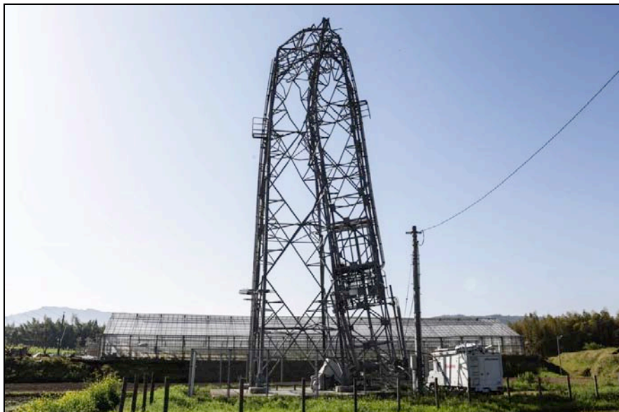
Figure 1-5. Ground level photo of the collapsed cell tower. (Courtesy: Guardian News & Media Ltd)
