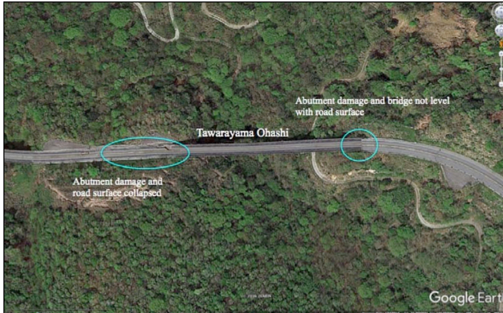
Figure 9-42. Aerial view of the failures of Tawarayama bridge. (Source: Google Earth)
