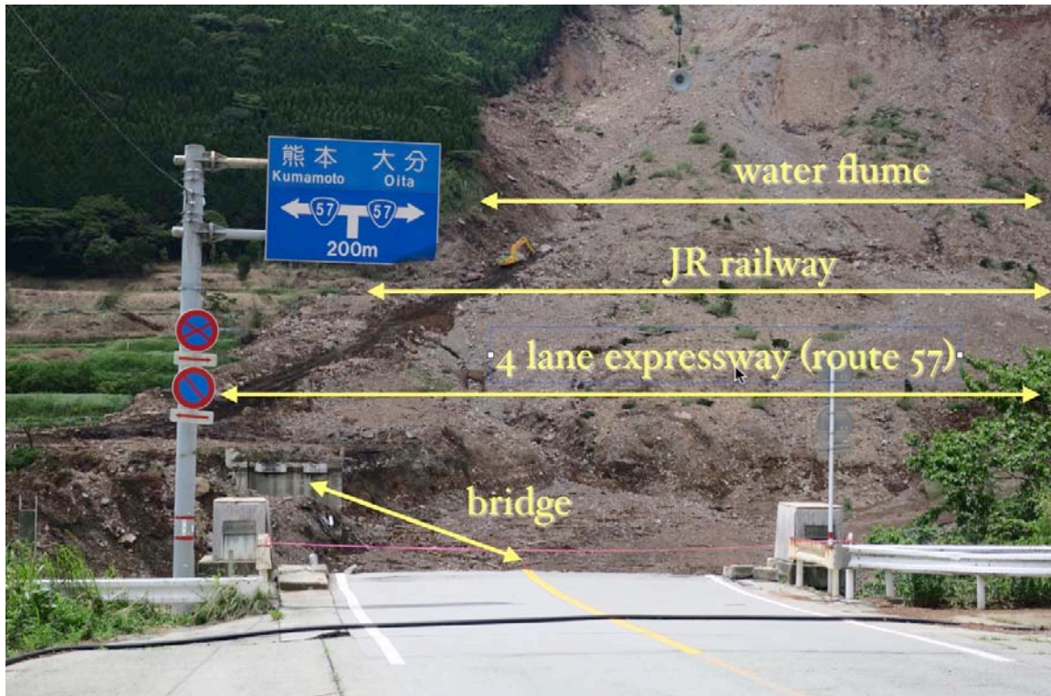
Figure 2-23. Landslide and Failed Infrastructure – East Facing Slope
