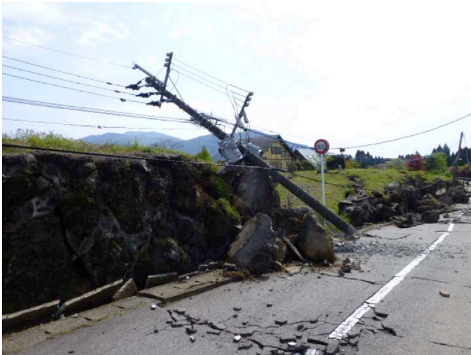
Figure 3-54. Distribution Pole Collapse
