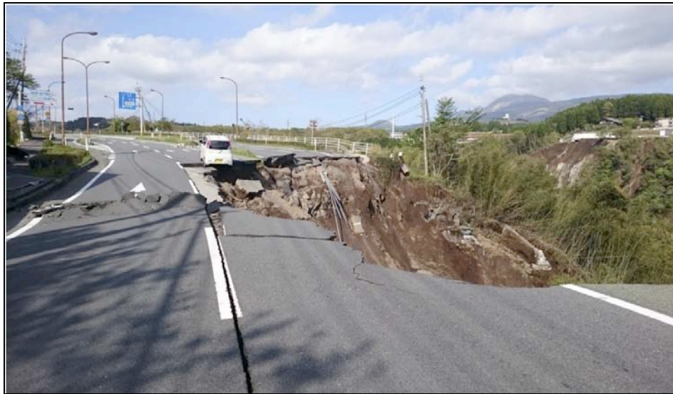
Figure 9-65. Slope failure took this part of the road (Route 57) down the slope
