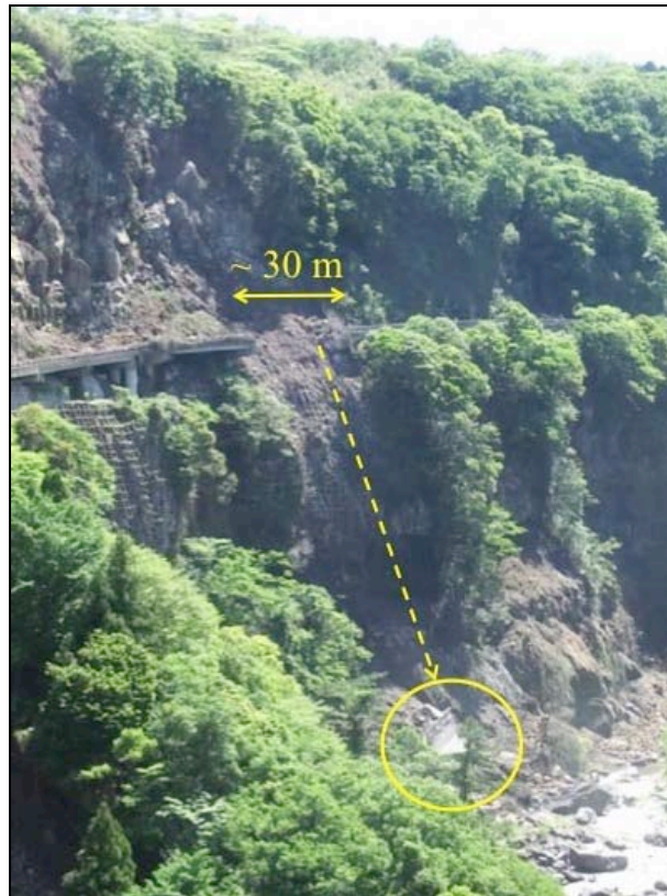
Figure 9-54, Another view showing the landslide that destroyed the bridge deck. Note part of the deck about 100 m down the slope
