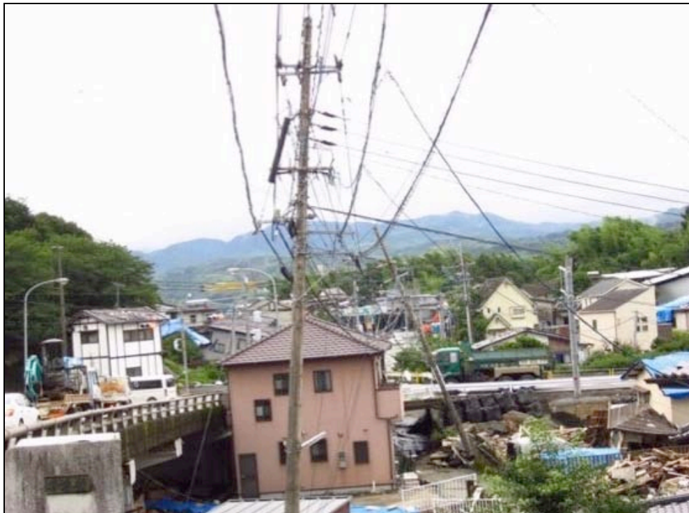
Figure 4-4. Many telecom and power cable poles were damaged in Mashiki Town (32.7901°N, 130.8209°E)
