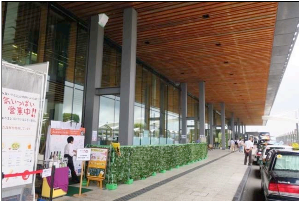
Figure 7-4. Exterior of Kumamoto Airport Domestic Terminal, the whole front wall is glass panel. There was signs of stress or displacement of the gasket around the glass panel.
