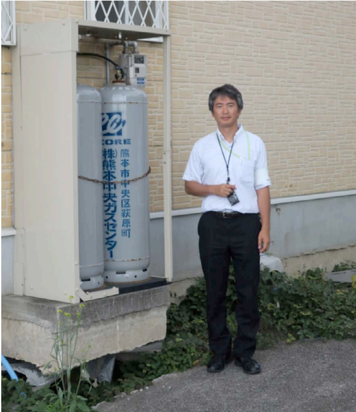
Figure 2-37. Differential settlement between pile supported house and propane tank pad and driveway (Prof. Shoji)
