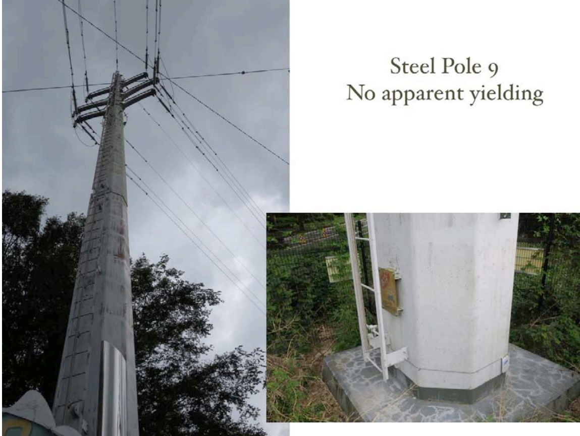
Figure 3-21. Tower 9 (Steel Pole)
