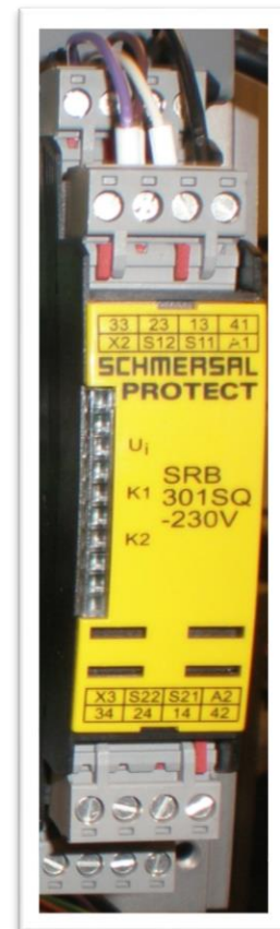
Figure 5.6.3 Emergency Stop Relay
