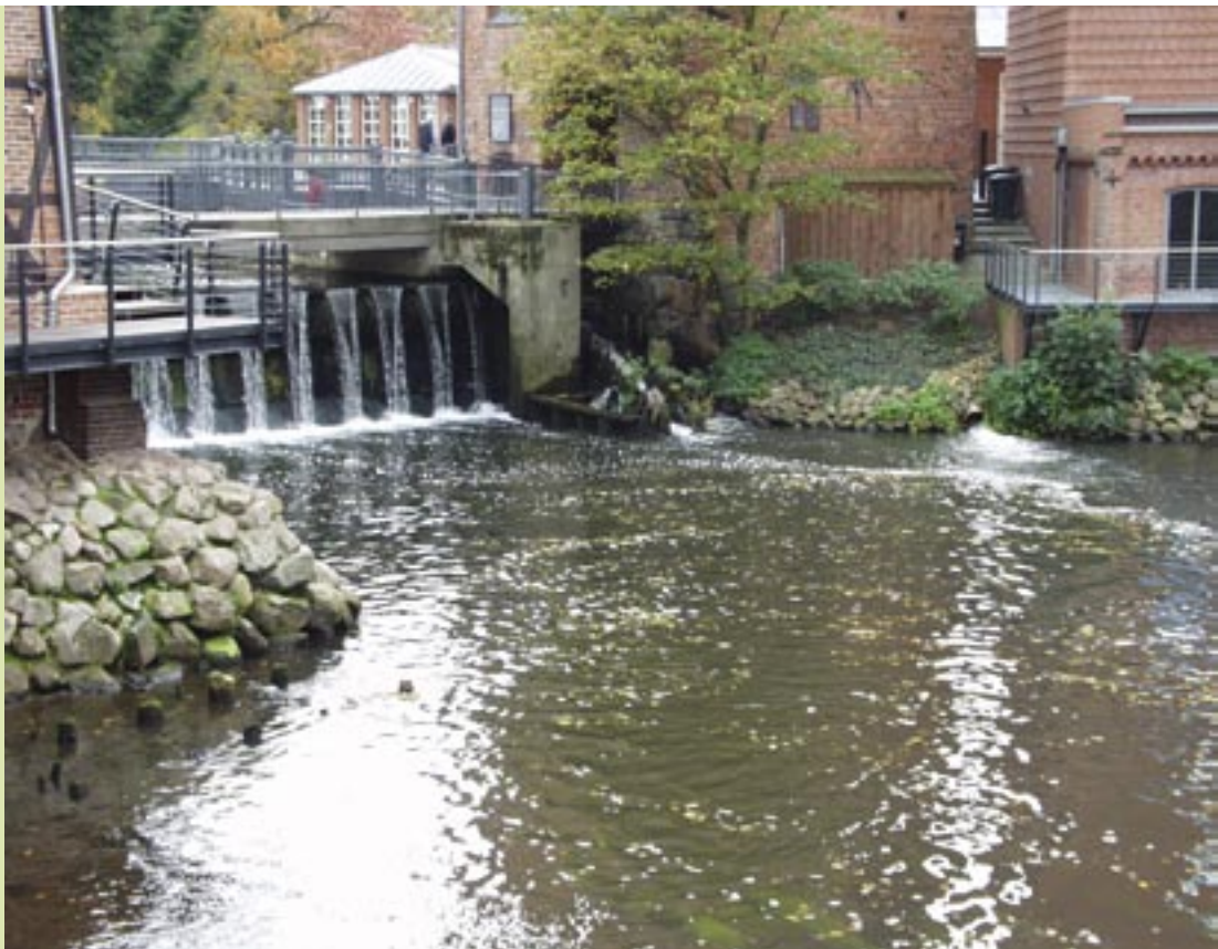
Weir in Lüneburg with fishway on the river Ilmenau
