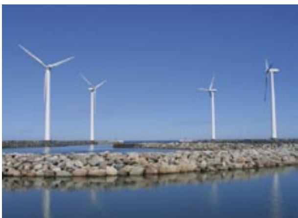
Wind power station
