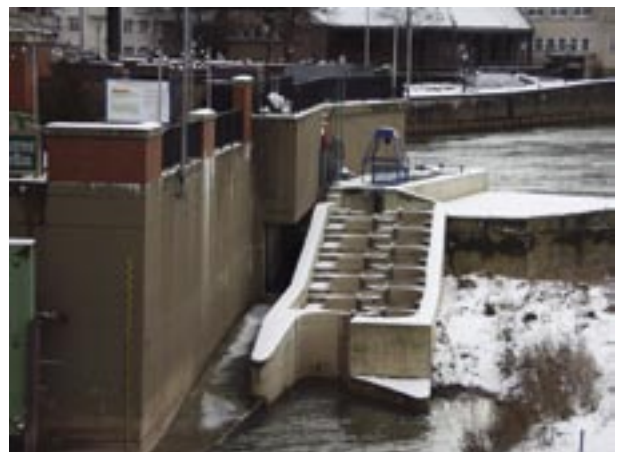
Fishpass at the Pfortmühle in Hameln
