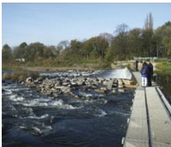
Fishpass and control station at Buisdorf/ Sieg
