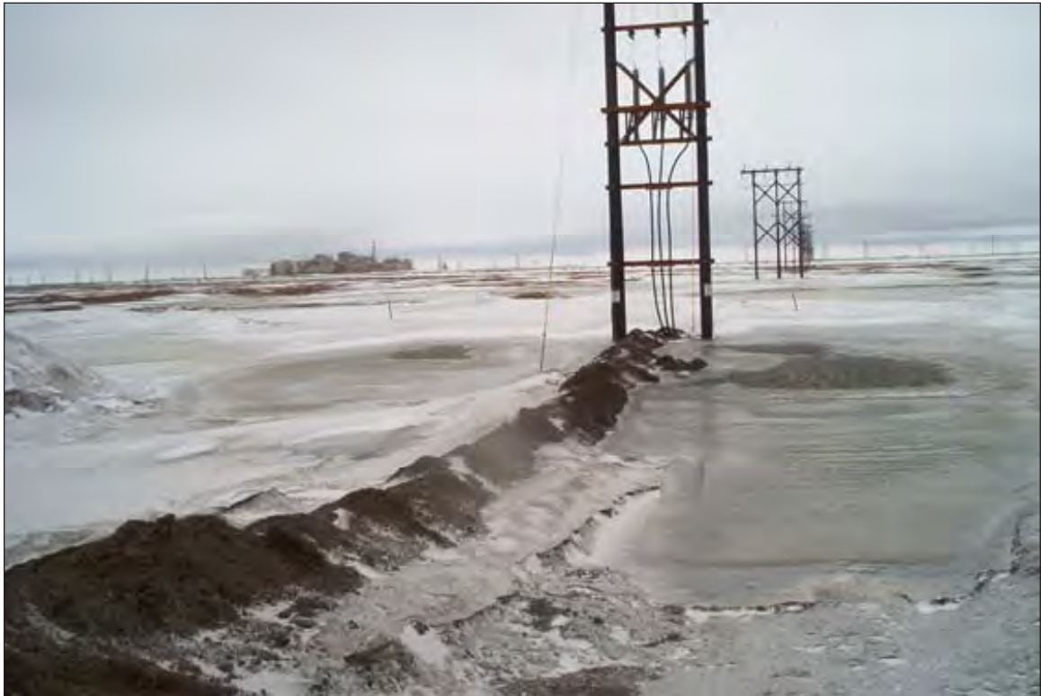
Figure D-20a. Power line trenching (near the pingo).
