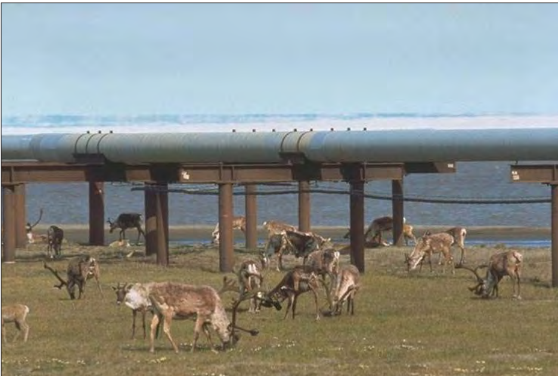
Figure D-5. Caribou and pipelines: Minimum height is 7 feet and separation from roads is 500 feet.
