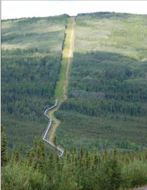
Figure 5. Pipeline transition between buried and elevated mode at permafrost boundary. Note shift from stunted spruce on footslope to taller trees. Photo by D.A. Walker.
