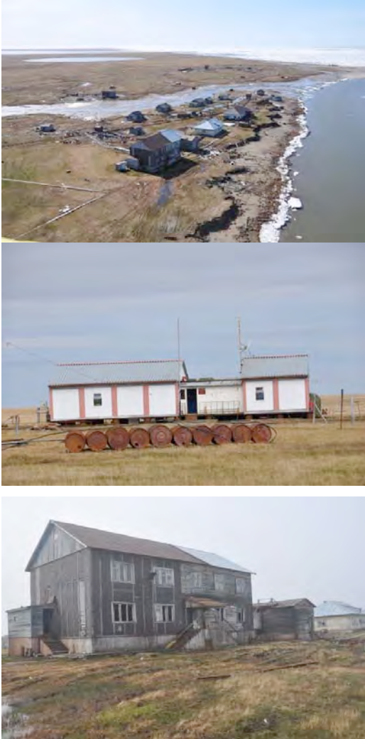
Figure 3. Ostrov Belyy facilities. Top: View of the abandoned portion of the polar meteorological at Ostrov Belyy. The house where the expedition stayed is in the foreground. Middle: Popov Meteorological station built in 2005. Bottom: Building where the expedition was housed. The house was built in 1986. Photos: D.A. Walker, d9009DSC_1256, 1347, 1721,
