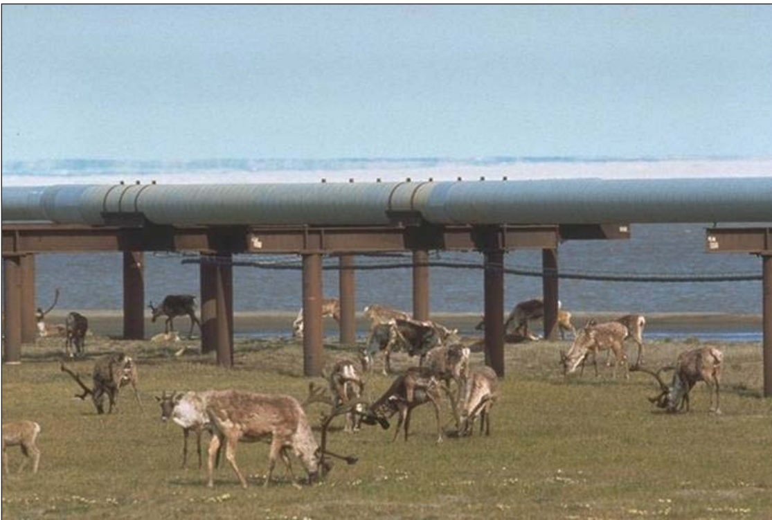
Figure D-5. Caribou and pipelines: Minimum height is 7 feet and separation from roads is 500 feet.
