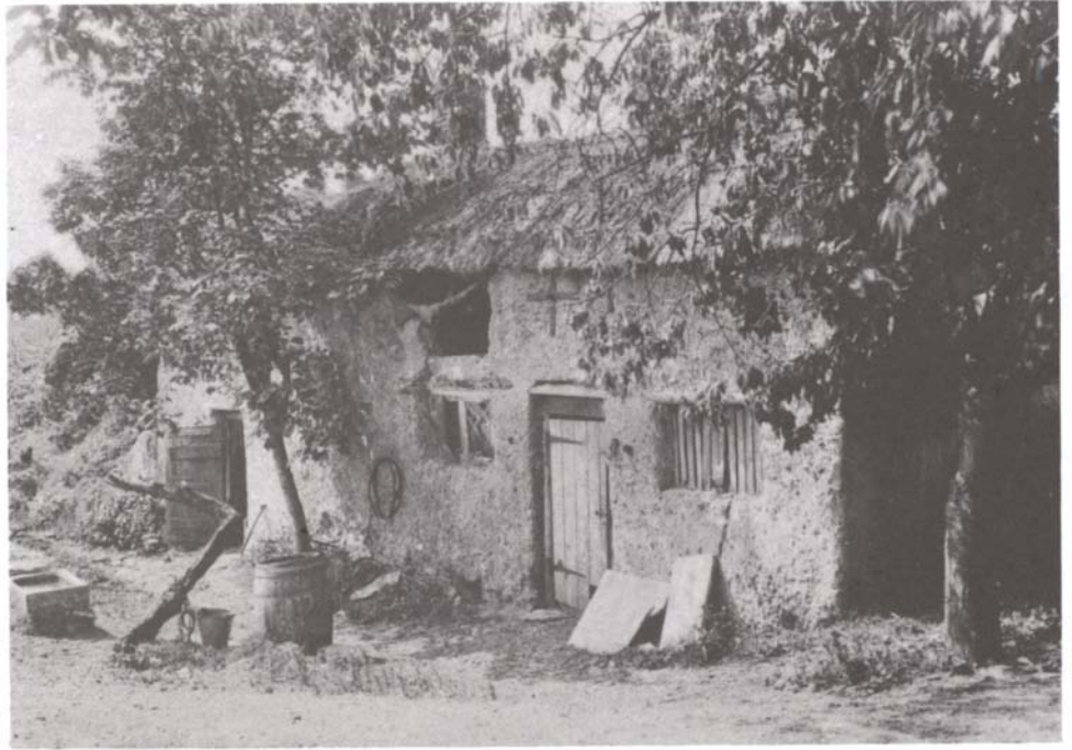
2. A nineteenth century basic monolithic cottage near Christchurch, Hampshire (now demolished). (Photograph reproduced courtesy of the Hampshire Museums Service)
