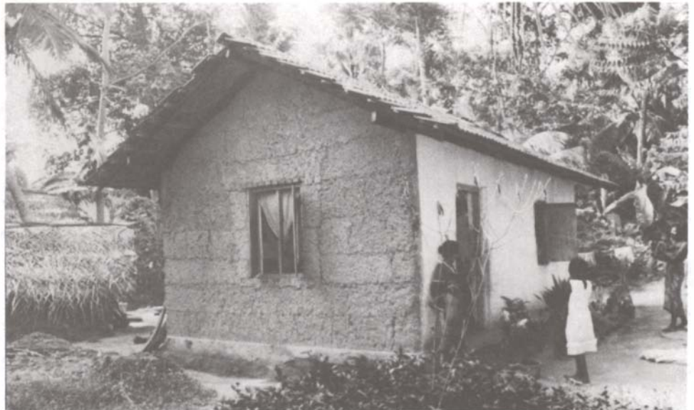
Figure 7. A completed house with rammed earth-walls and a tile roof with the front wall plastered and white-washed; the side-wall shows how the work progressed.
