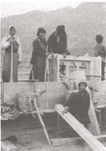
Fig. 4. Placing the windows.
