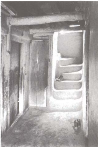
The entrance lobby of a typical traditional house showing the timber and mud interior finishes. This front lobby, located at the center of the house, is considered to be the safest place to go to during an earthquake. (Running out of the house is more dangerous.)
