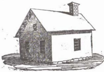
Fig. 10. Henry Ellsworth's rammed earth house in Indiana.
