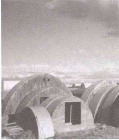
3. Plywood forms for arches. Photo: James Steele.
