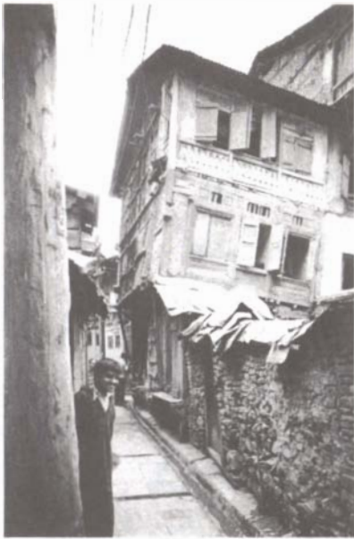
Many of the houses in Srinagar remain radically askew from weak soil and past earthquakes.
