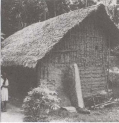
Figure 12. The exposed timber skeleton, of a wattle and daub wall, after the loss of the second coating of mud.
