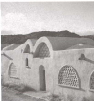
6. Cement plaster coating. Photo: James Steele.
