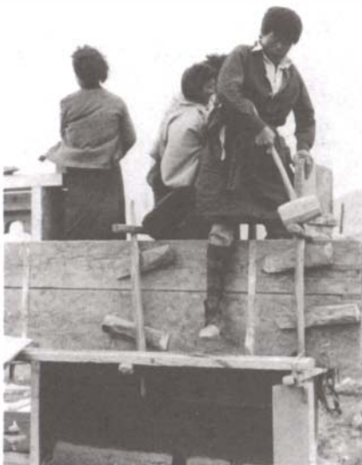
Fig. 3. Setting the planks.
