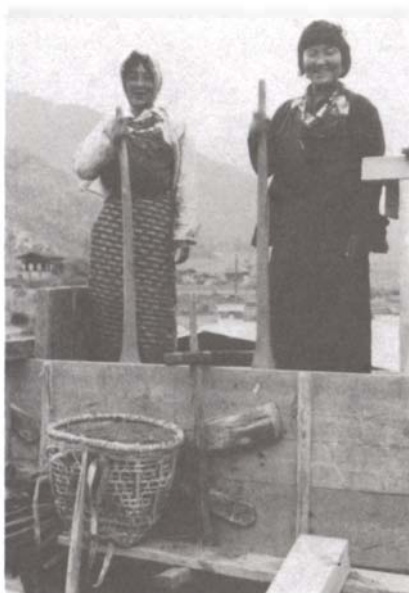
Fig. 2. Bhutan, process of constructing "pisé de terre".
