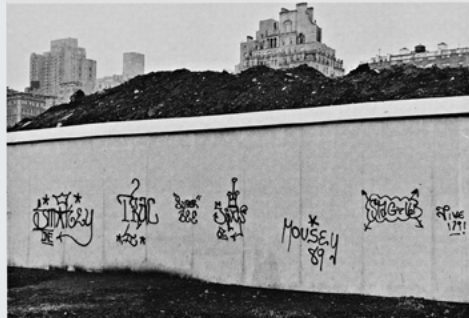
Central Park, 1972, construction site with goats behind the Metropolitan Museum of Art. All 1972 photographs by Robert Smithson and Robert Rauschenberg.
