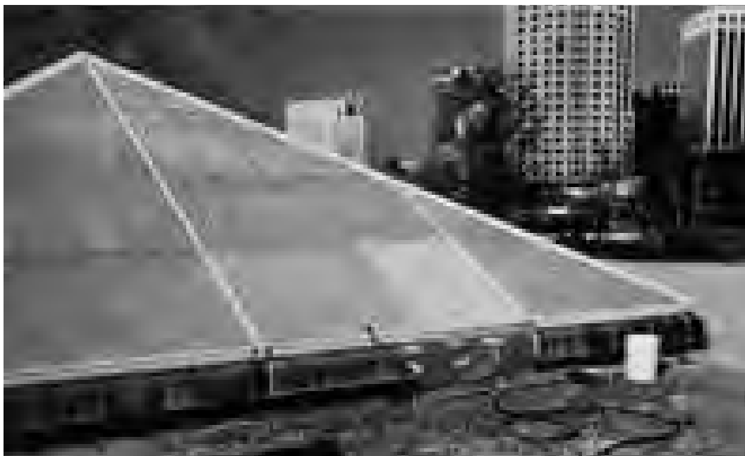
Figure 16.6. Unlike some plastics, fiber reinforced plastic can be repaired. Techniques range from resurfacing to cutting out and replacing the defective material. Translucent Kalwall panels that were damaged in a skylight installation have been resurfaced (bottom).
