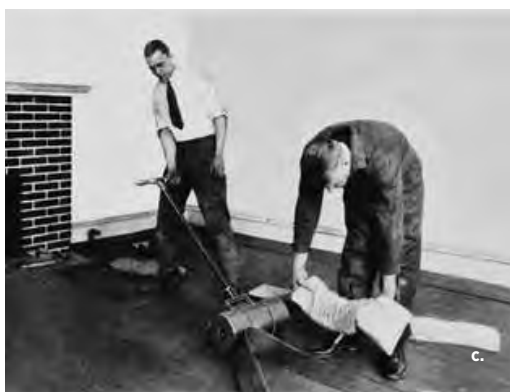
Figure 27.3a-c. a. Applying felt under linoleum with paste was a common installation practice by the late 1920s. b. When the linoleum was installed, edges of the adjoining linoleum overlapped and seams were subsequently cut with a special tool. c. Unpasted areas near the seams were sealed with waterproof cement and the linoleum was then rolled and seams were weighted with sandbags until the floor was dry.
