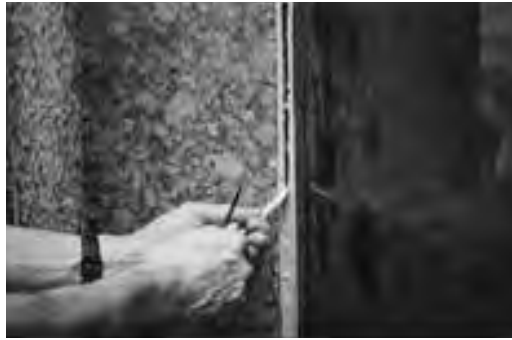
Figure 36.3. In-place field adhesion pull tests provide information about a sealant's adhesive, cohesive, and elastic properties.
