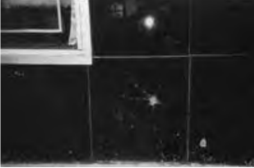
Figure 25.5. The most common causes of structural glass breakage include accidental impact and vandalism. This street-level panel requires replacement.
