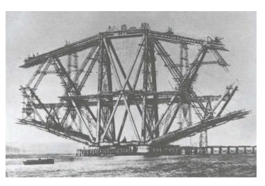
Fig. 55. BRIDGE OVER THE FIRTH OF FORTH, 1883–89 CONSTRUCTORS: JOHN FOWLER and [Sir] BENJ[amin] BACKER
