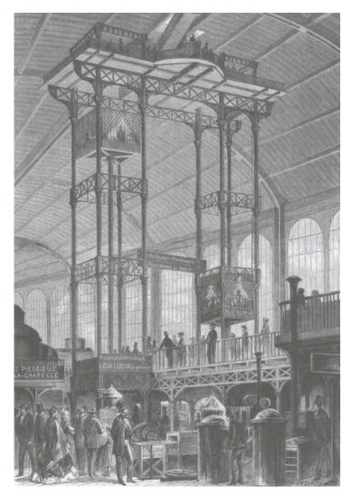
Fig. 36. EXHIBITION, PARIS 1867. GALERIE DES MACHINES Mechanical elevator to the roof platform.
