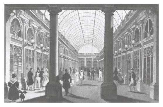
Fig. 9. [Pierre-François-Léonard] FONTAINE: Galerie d'Orléans in the Palais-Royal (Paris) 1829-31 Even FONTAINE, one of the founders of the Empire style, converted in old age to the new material. In 1835-36 he replaced the wooden floor of the Galerie des Batailles in Versailles with iron panels. Galleries like those in the Palais-Royal underwent further development in Italy. They represent for us the point of departure for new building problems: railroad stations, etc.
