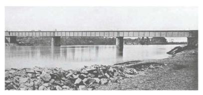
Fig. 31. Pont de Longon (Garonne) 1854-55 Span of 77 meters. Height of girders 5.5 meters.
