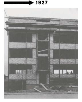
Fig. 42. The IRON SKELETON as HOUSING FORM. 1927. Apartment block of the Stuttgart Werkbundsiedlung by Mies van der Rohe. 1927 It took more than half a century before the importance of the iron skeleton for apartment houses was recognized. The conclusion to be drawn here
