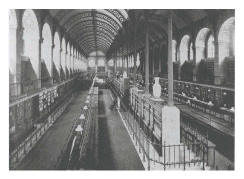
Fig. 13. H. LABROUSTE: LIBRARY OF SAINTE-GENEVIÈVE Reading room with cast-iron truss. The windows are placed high to allow continuous shelving.
