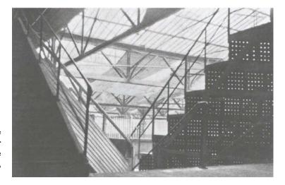
Fig. 65. VELODROME d'Hiver, Paris Gallery bleachers. The bleacher rows that are perforated and cut in order to achieve lightness enable new effects through light, structure, material variety.
