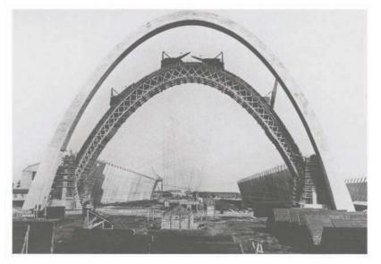
Fig. 66. LIMOUSIN AND COMPANY (Freyssinet Technique). ORLY HANGAR 1916 View of one vault ELE-MENT in a finished state and of another with scaffolding. Each element has a span of 80 meters, width 7.5 meters, height 56 meters. One arch was erected every eight days.
