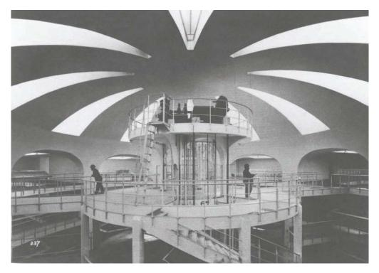
Fig. 136. BRICE & SAINRAPT. VAULT (TOUR FORTE) of the BANQUE DE FRANCE Ten stories. Underground. Height 32 meters. Diameter 50 meters. Closure by means of movable concrete wings.
