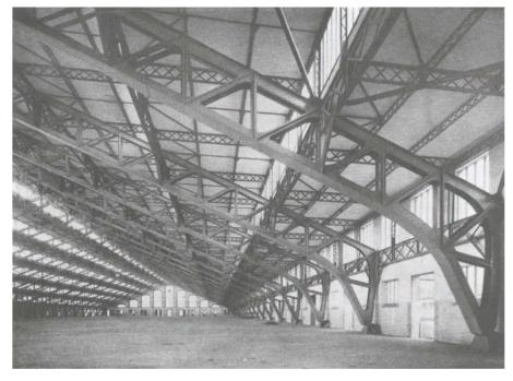
Fig. 54. TONY GARNIER: SLAUGHTERHOUSE IN LYONS Dimensions: WIDTH 80 meters, LENGTH 210 meters.
