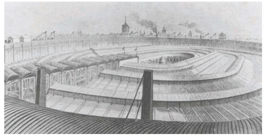
Fig. 34. VIEW FROM THE PLATFORM of the seven-ring gallery of glass and corrugated sheet metal.
