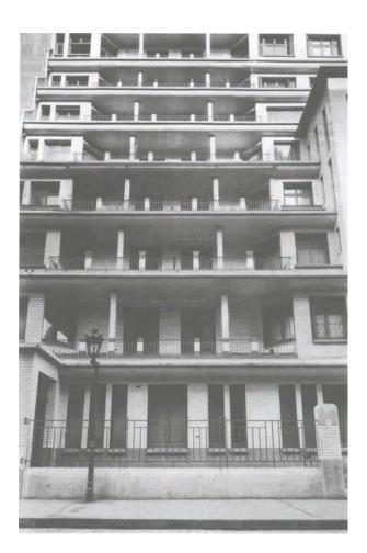
Fig. 124. HENRI SAUVAGE. RUE DES AMIRAUX 1925 The balconies are recessed in order to
