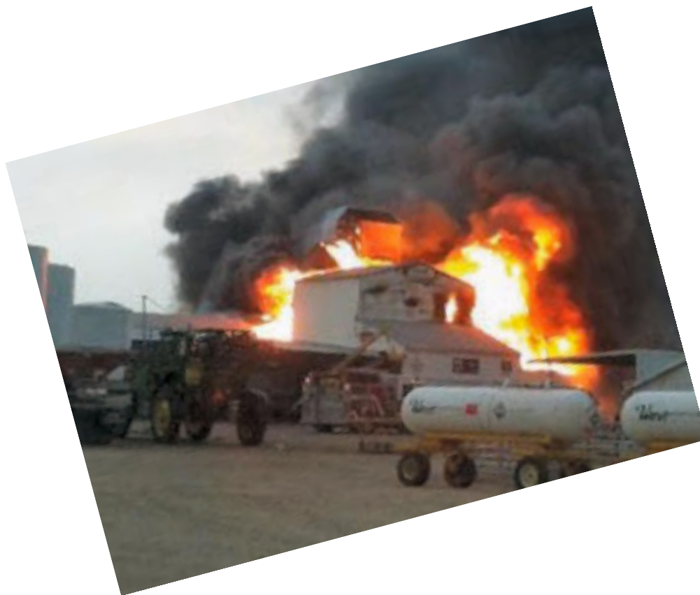
Figure 7: Close up of the Seed and Fertilizer Building during fire (viewed from east)
