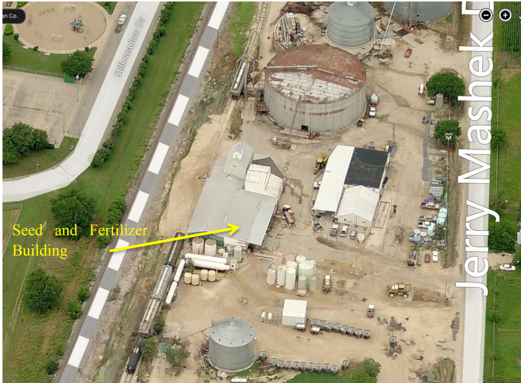
Figure 2: West Fertilizer Facility – viewed from the south
