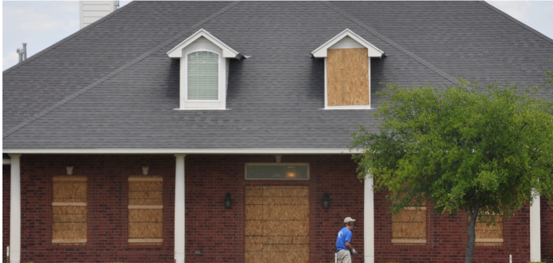
Figure 20: House with windows broken approximately 1 km from the incident
