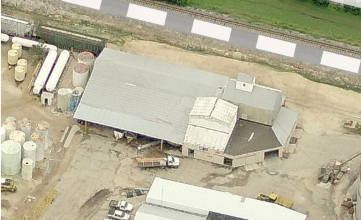
Figure 5: Close up of the Seed and Fertilizer Building (viewed from east)
