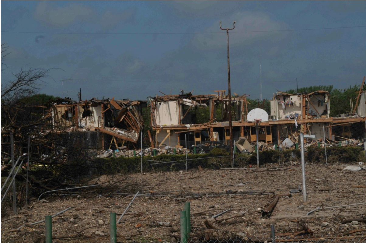
Figure 18: Blast damage to the basketball court and apartment complex west of the plant
