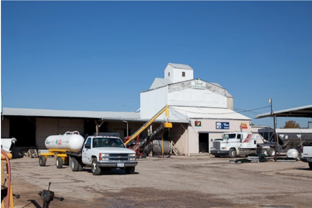
Figure 6: Close up of the Seed and Fertilizer Building (viewed from east, ground level)
