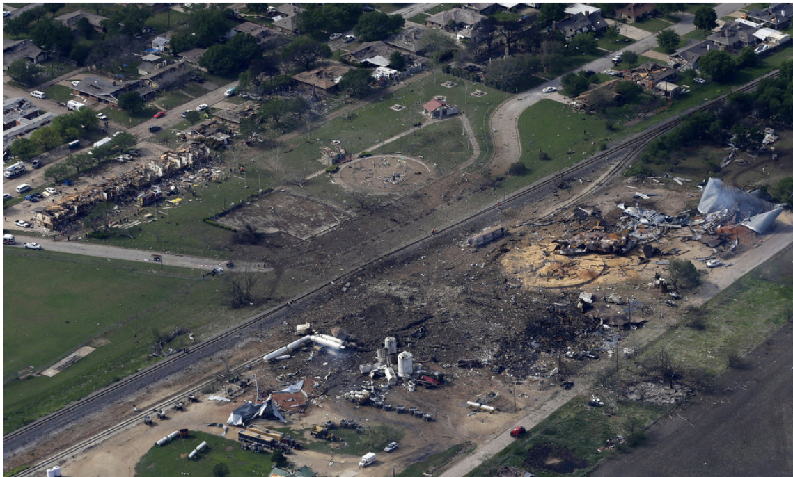
Figure 14: Blast damage as viewed from the southeast
