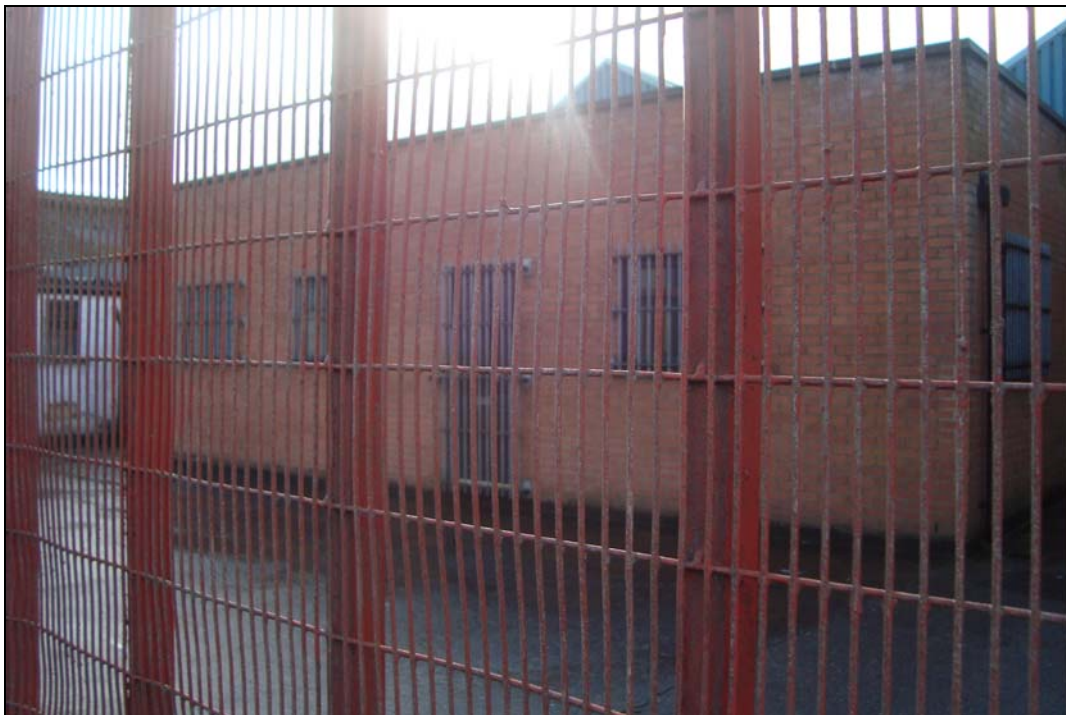
Plate 81: Battery charging block
