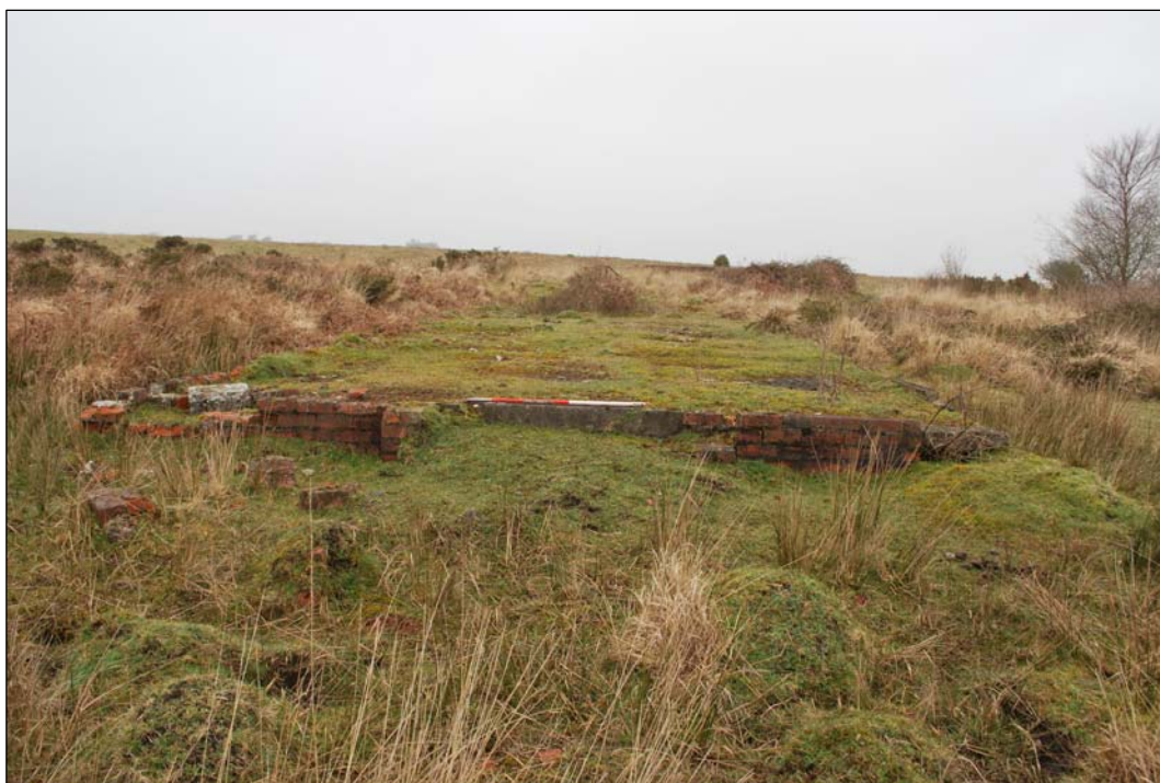
Plate 26: Brick platform with the remains of a concrete step at the front of the building
