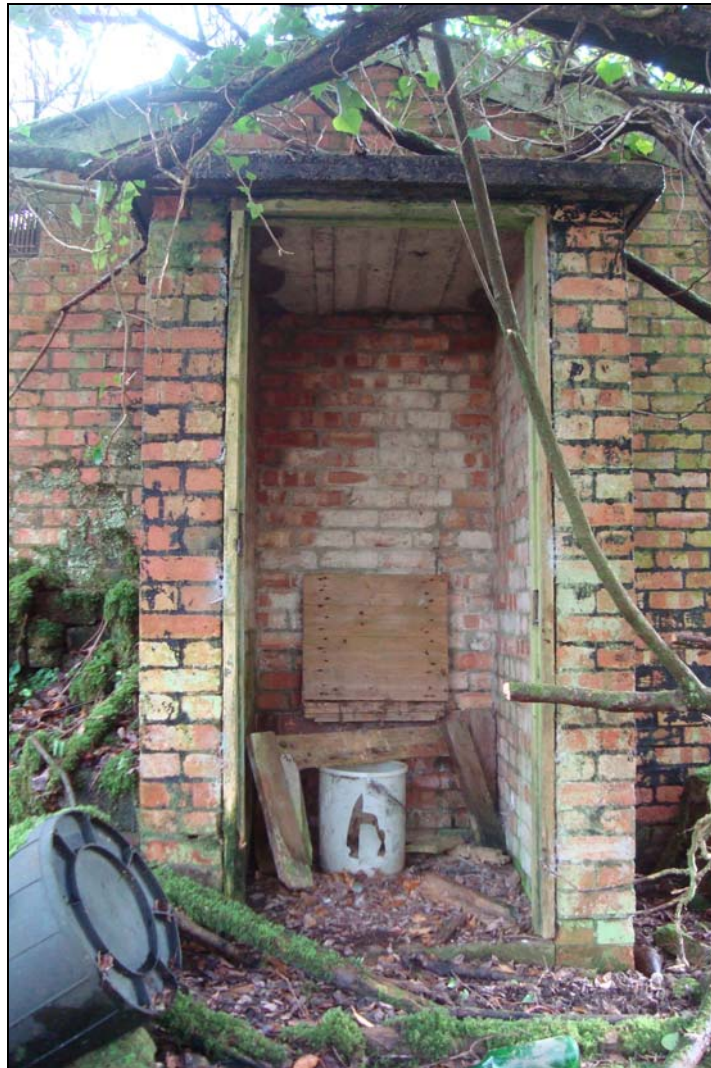
Plate 11: Latrine. Note the in situ wooden Elsan toilet lid and surround
