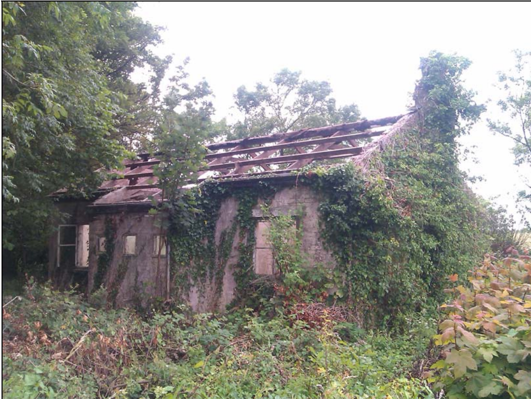
Plate 66: Rear elevation of the Satellite Station Watch Office. Note the latrine extension with its three square windows
