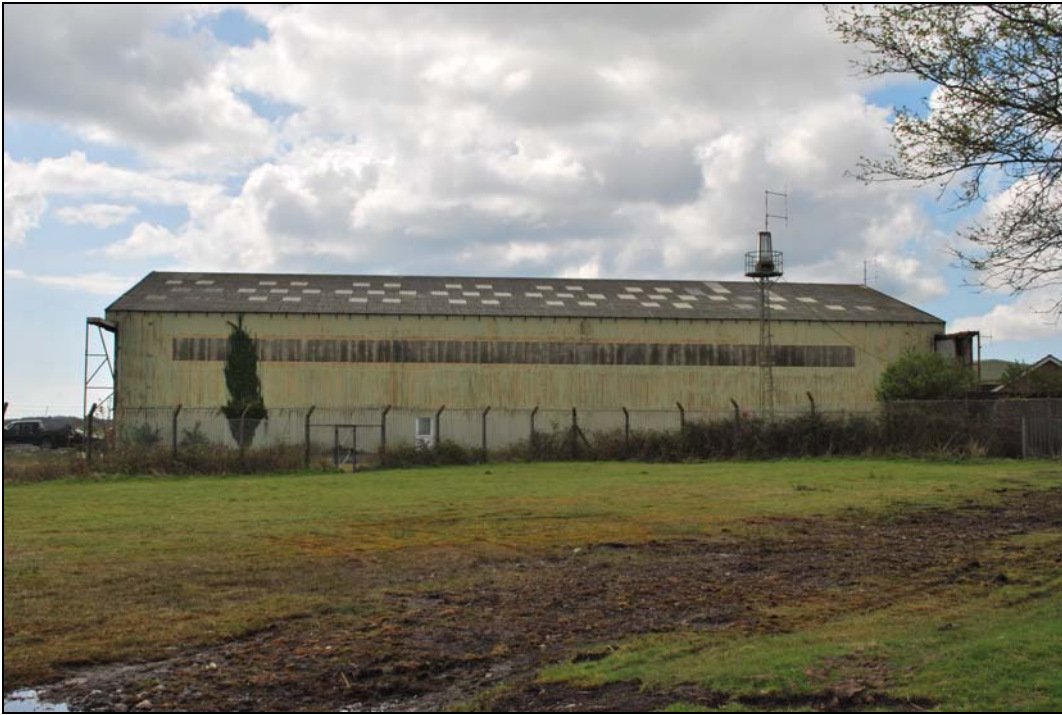
Plate 37: The surviving Bellman hangar. View to the southwest
