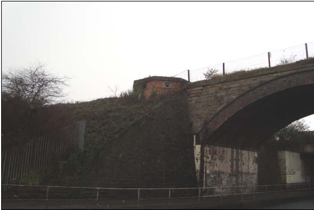
Plate 82: The pillbox protecting the airfields western area.
