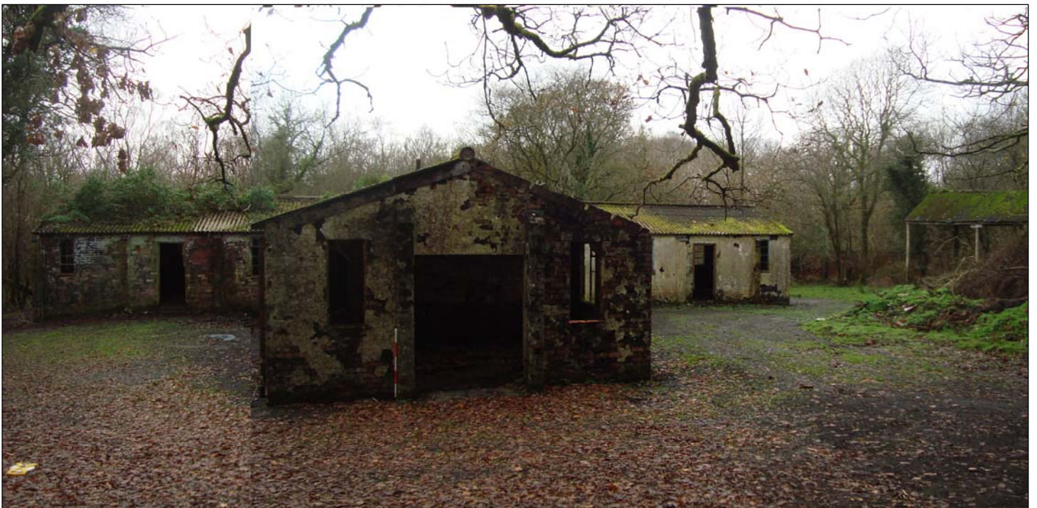
Plate 8: Flight Office complex (southwest elevation)
