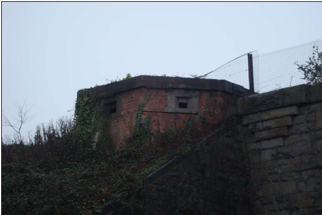
Plate 83: Close-up of the pillbox on the railway bridge's eastern flank
