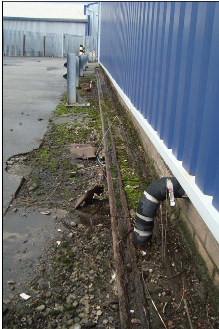
Plate 80: The original door runners at the front of the hangar
