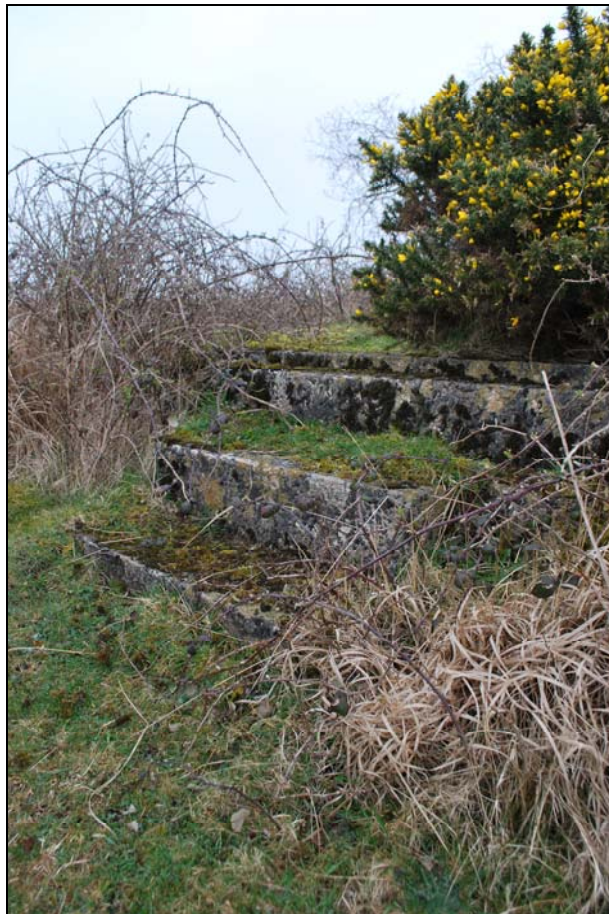
Plate 34: Set of three concrete stairs used to access the building
