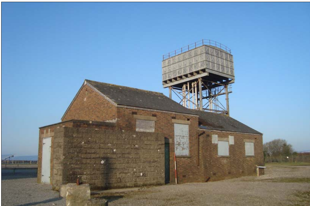
Plate 55: Side elevation (northwest facing)
