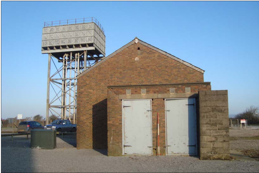
Plate 54: Front of the sub-station PRN 06340m (north facing elevation)
