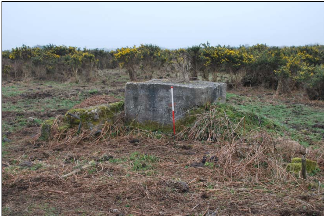
Plate 18: Concrete block surrounded by assorted concrete rubble
