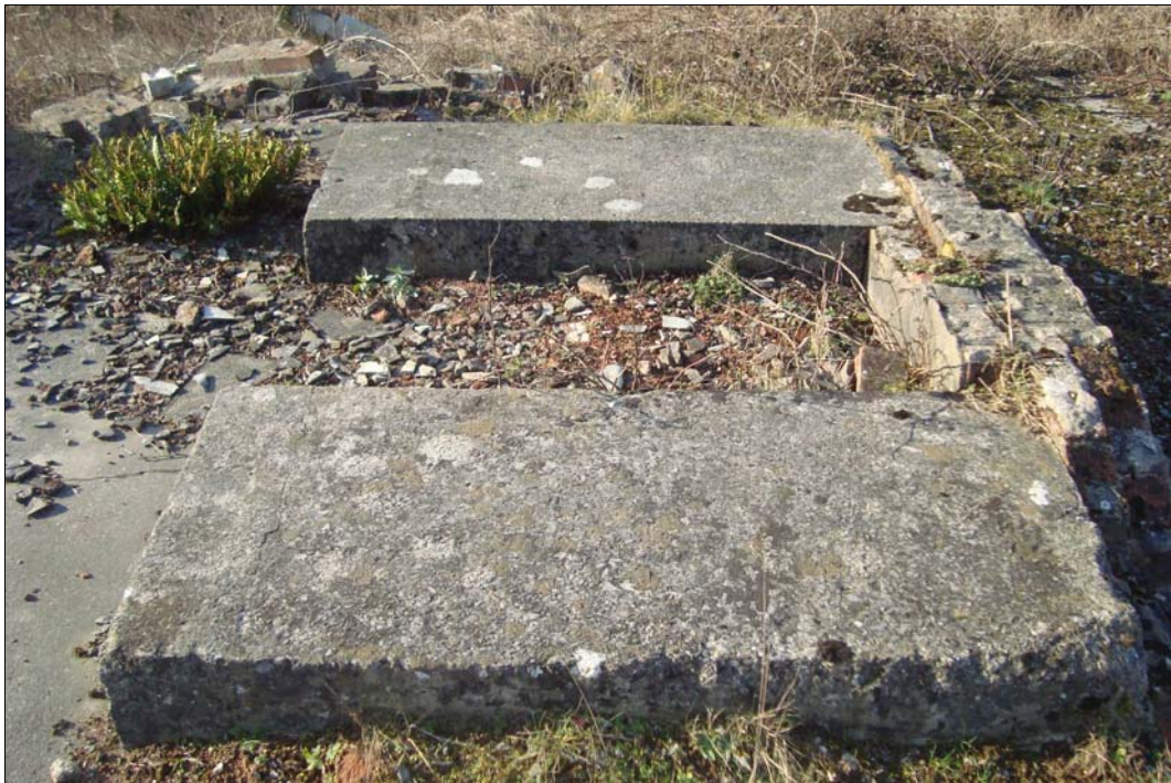
Plate 49: The concrete footings for the projection equipment
