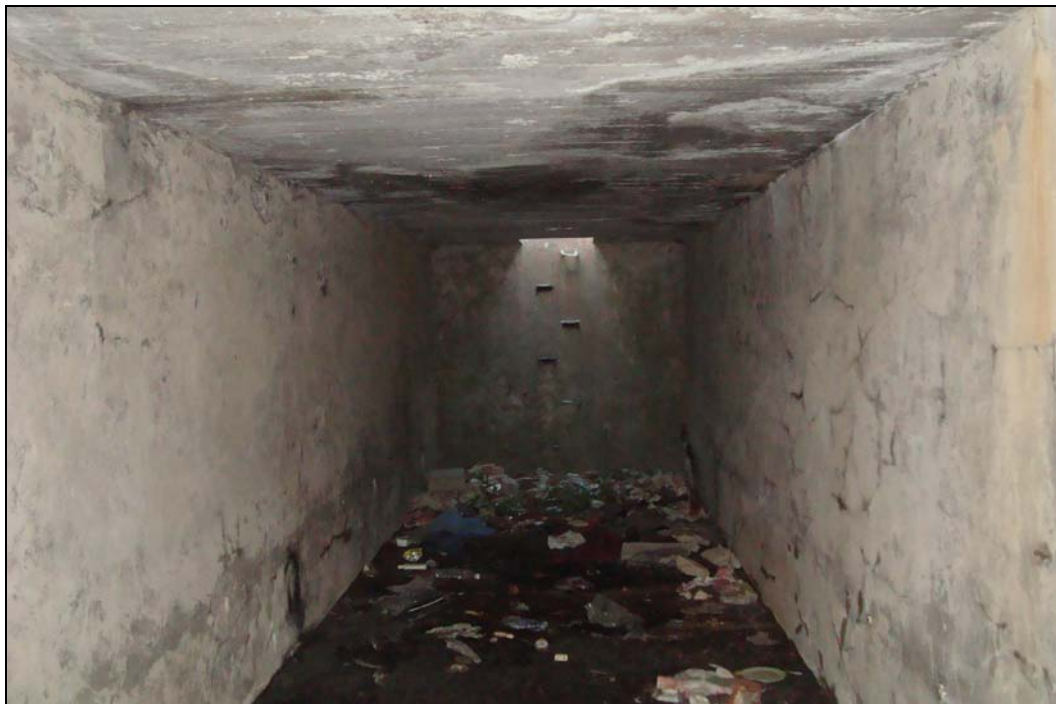
Plate 62: Interior of the store. Note the 'C' ring style rungs at the rear of the structure
