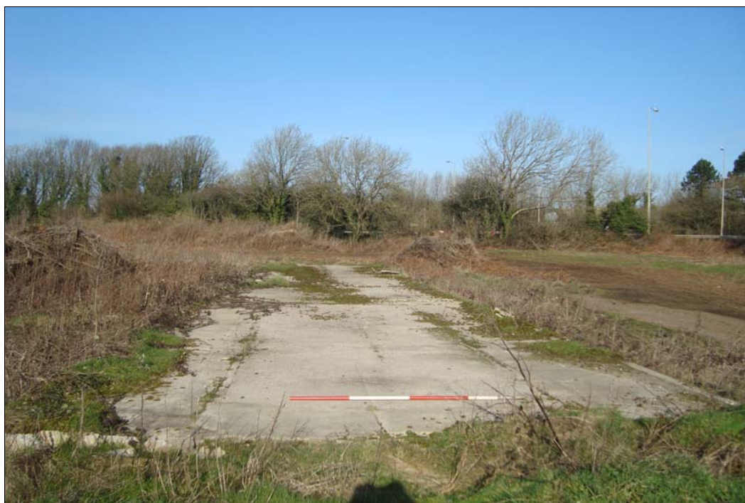
Plate 46: The remains of the WAAF combined dining room and institute
