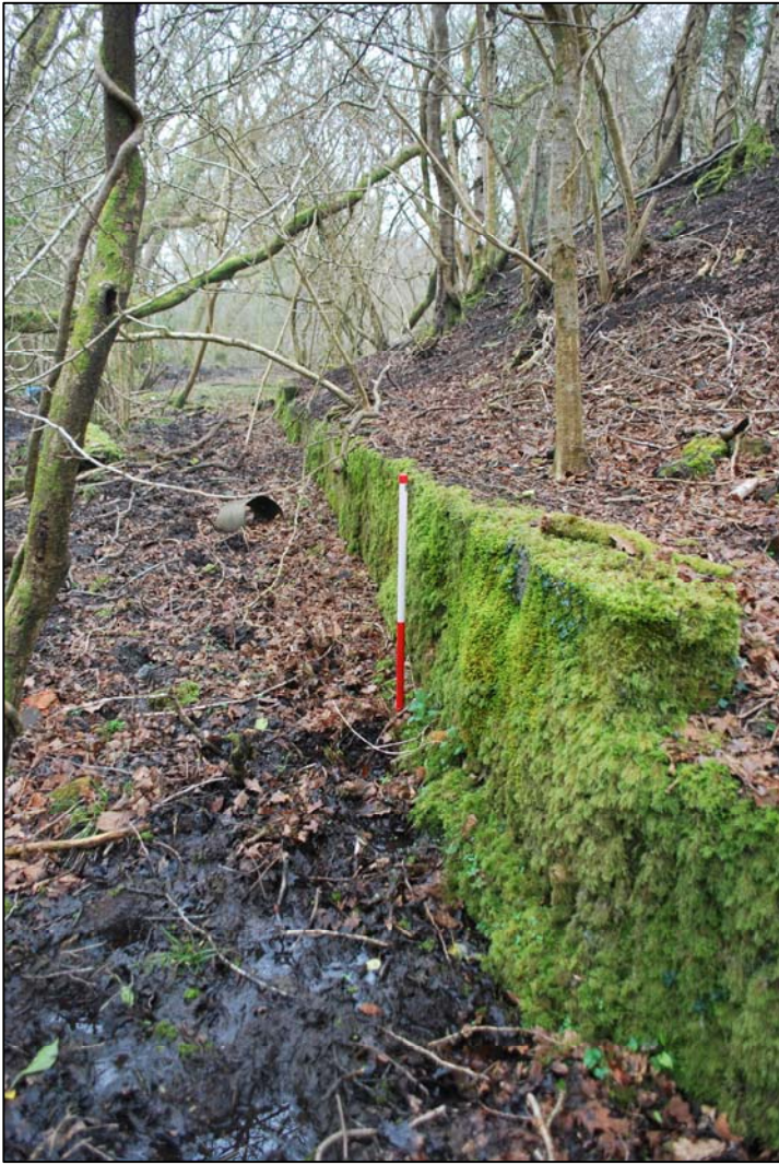
Plate 3: Retaining wall around the base of Fighter Pen 5
