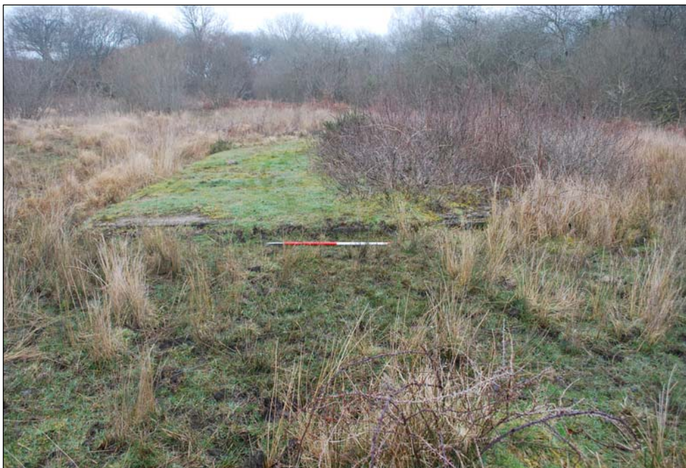
Plate 4: The concrete base is all that remains of S S A Store
