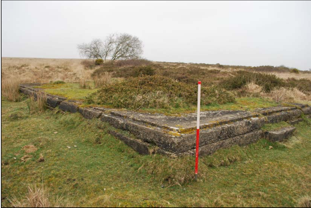
Plate 31: The concrete building base. Note the single front step at the front of the structure.
