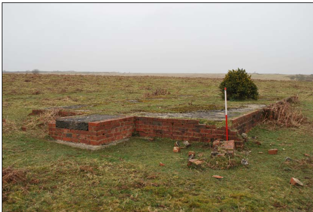
Plate 28: Brick building. View to the northeast
