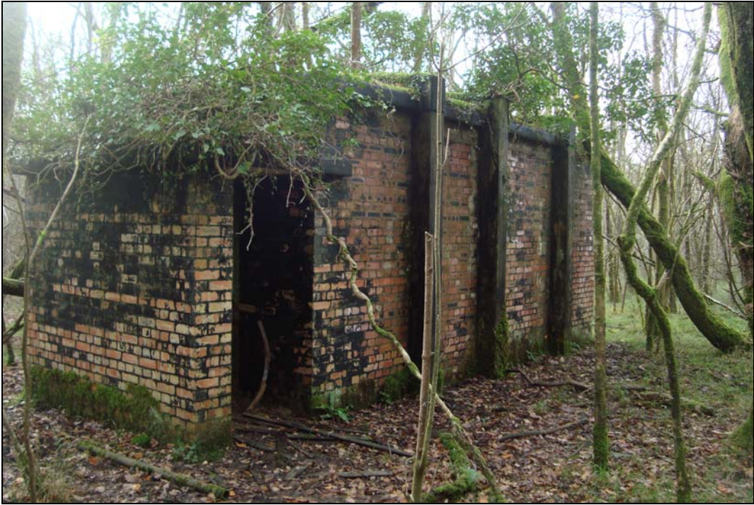
Plate 12: Hardened Sleeping Shelter. Note the reinforced bands and blast porch
