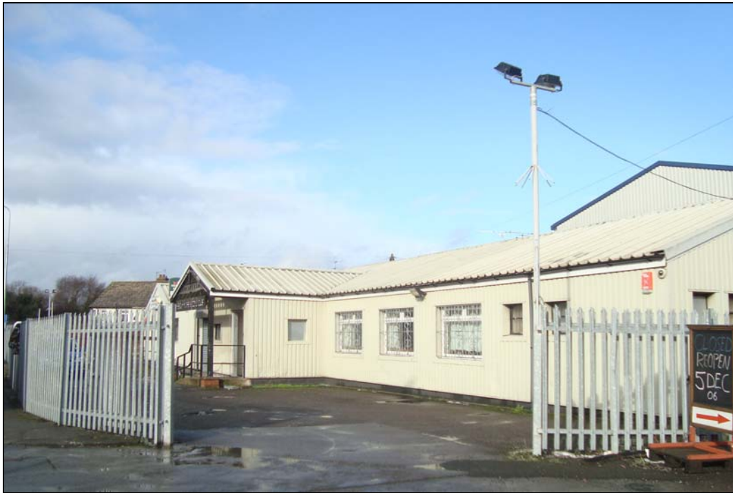
Plate 74: Station Headquarters looking northwest showing the amount of alteration carried out
