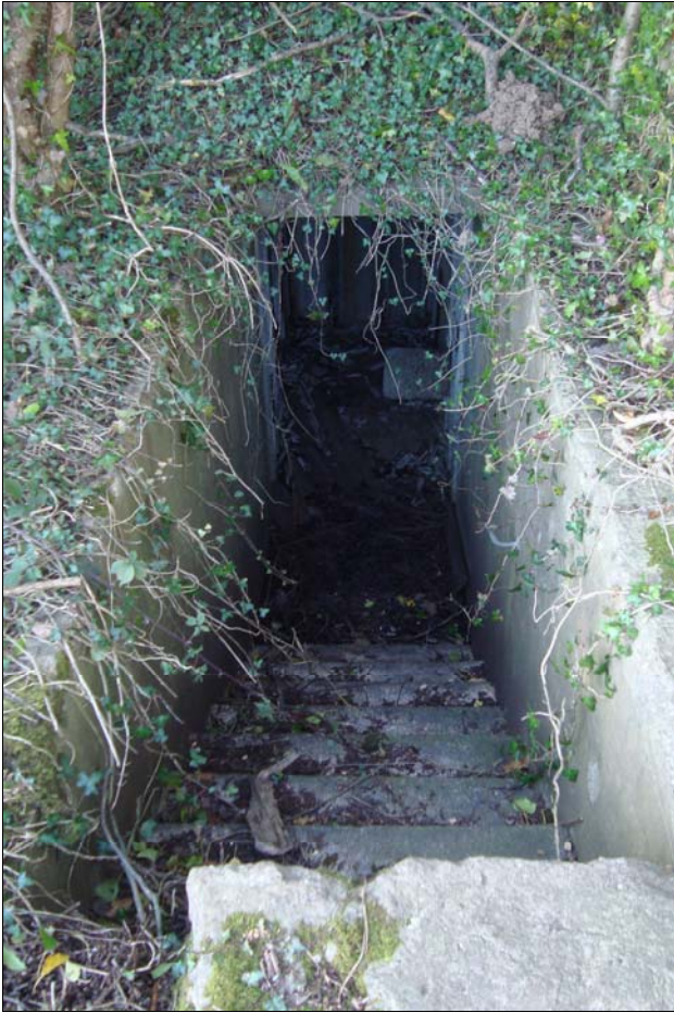
Plate 54: entrance to the shelter
