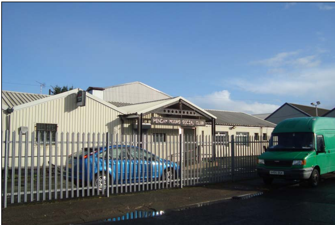
Plate 75: Station Headquarters showing the amount of alteration carried out
