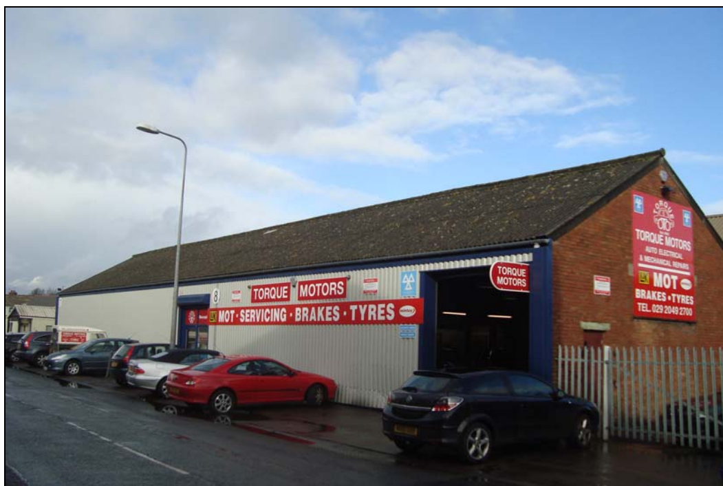
Plate 76: MT Shed and Offices looking northwest
