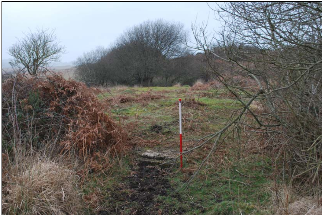
Plate 21: Edge of the two tier building platform
