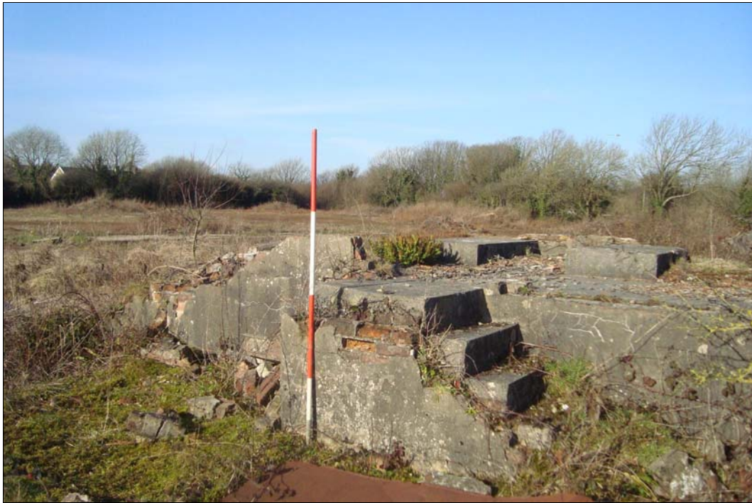
Plate 50: Steps leading to the projection booth extension at the rear of the building
