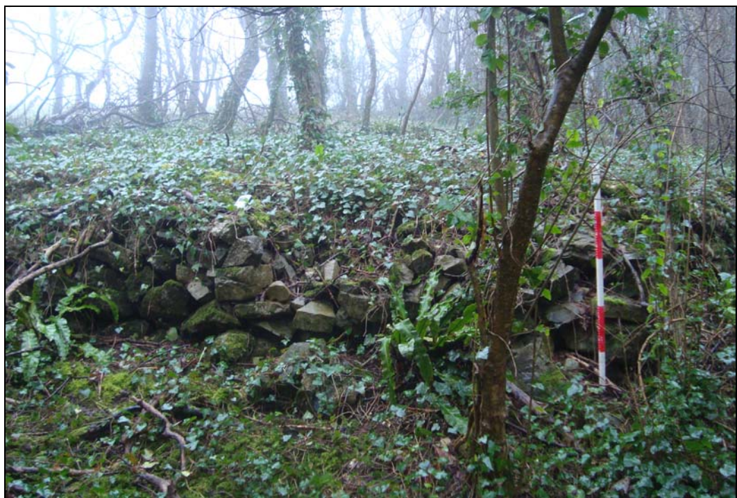
Plate 71: Dispersal platform showing construction technique (south facing elevation)
