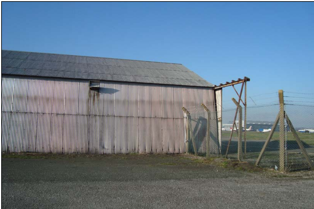
Plate 73: Southeast facing section showing the corrugated panelling construction
