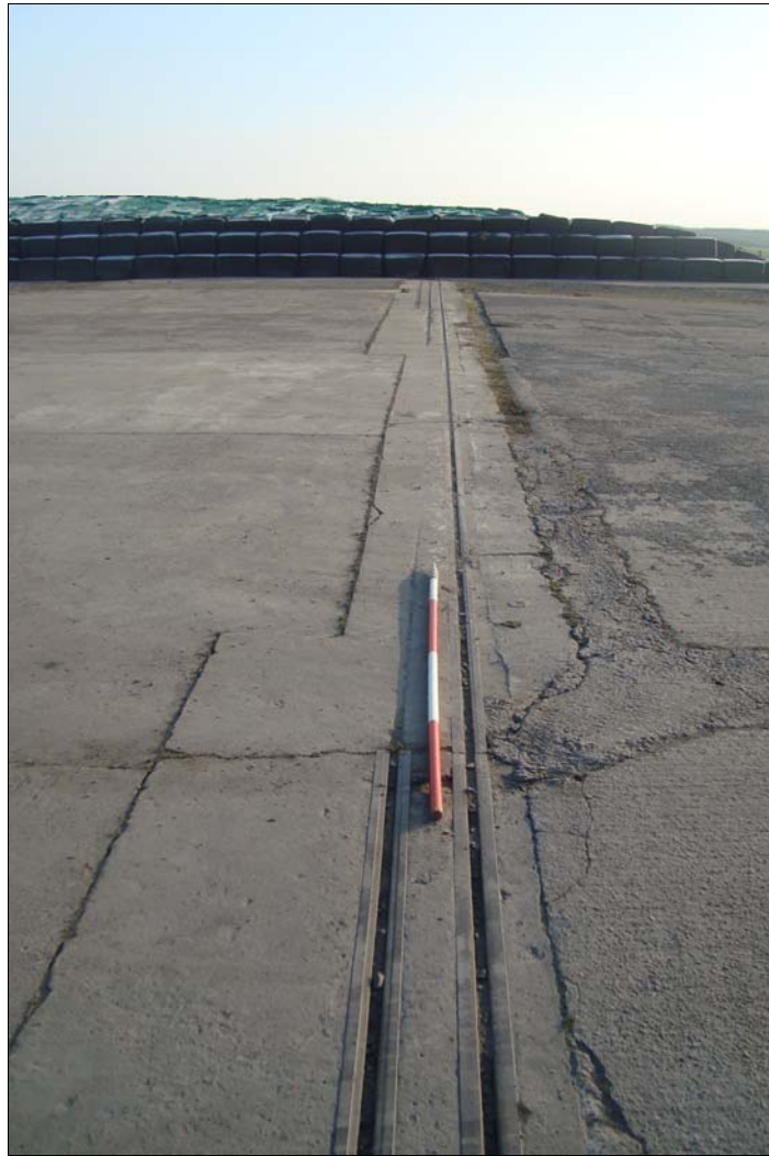
Plate 59: All that remains of the Bellman hangar are the door runners
