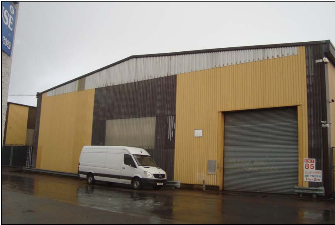
Plate 77: The main entrance to Hangar 115 showing the alterations
