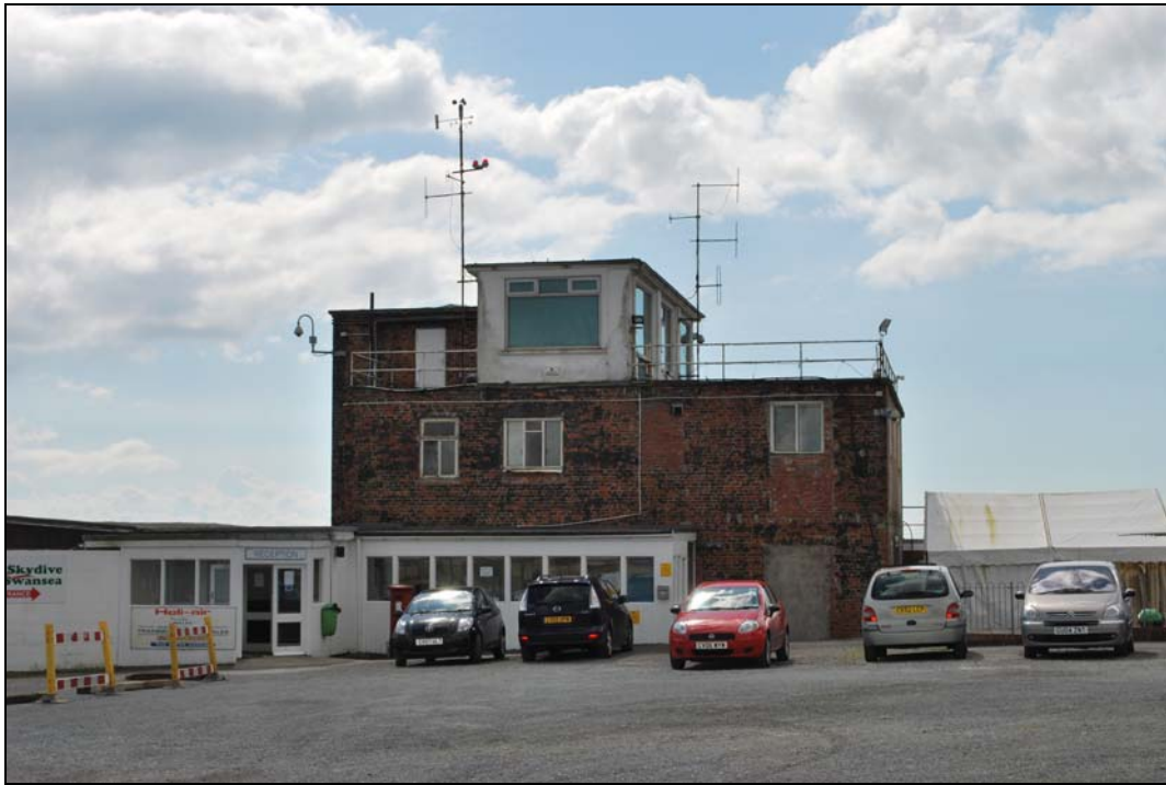
Plate 38: The Control Tower at RAF Fairwood Common (northeast facing elevation)
