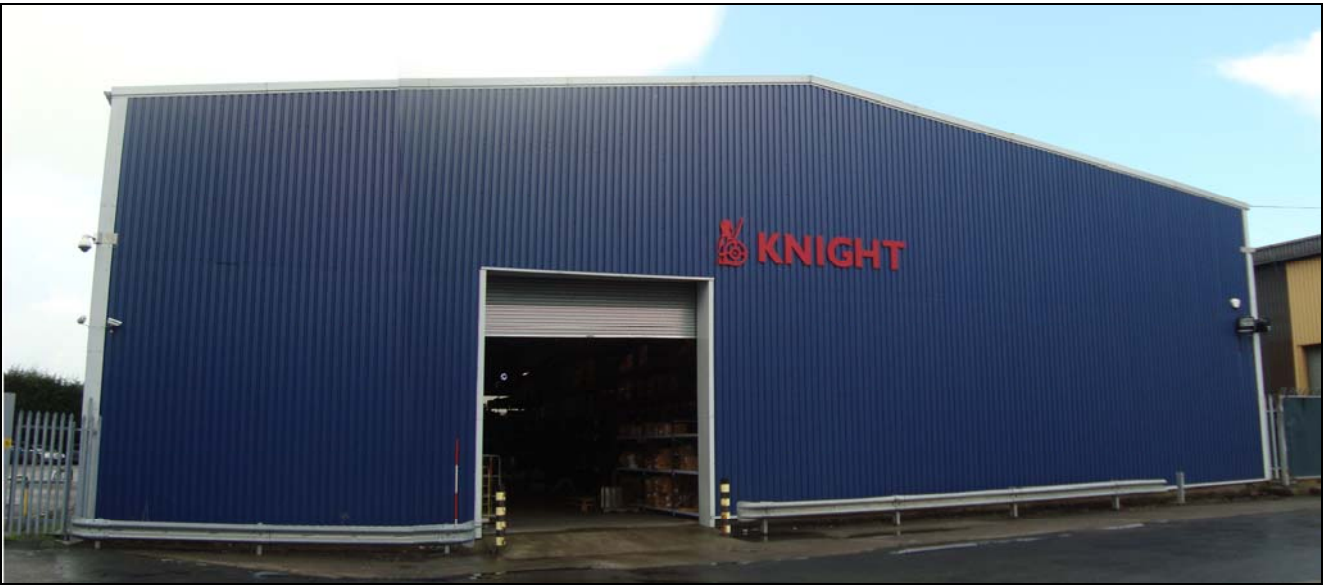
Plate 78: Front of hangar 116 showing the cladding and alterations
