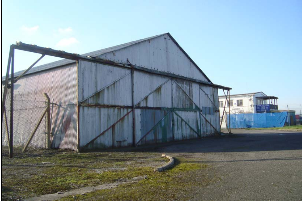
Plate 72: Robin hanger 2204/41. Front of hangar shows the surviving door gantry
