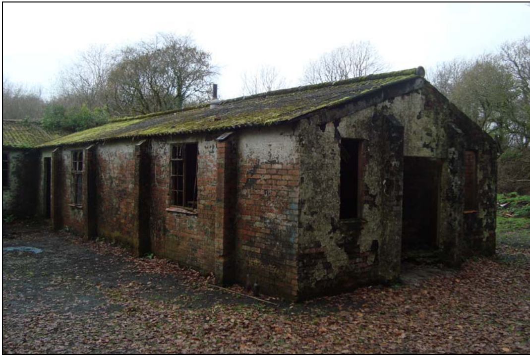
Plate 7: Flight Office. View to the west.
