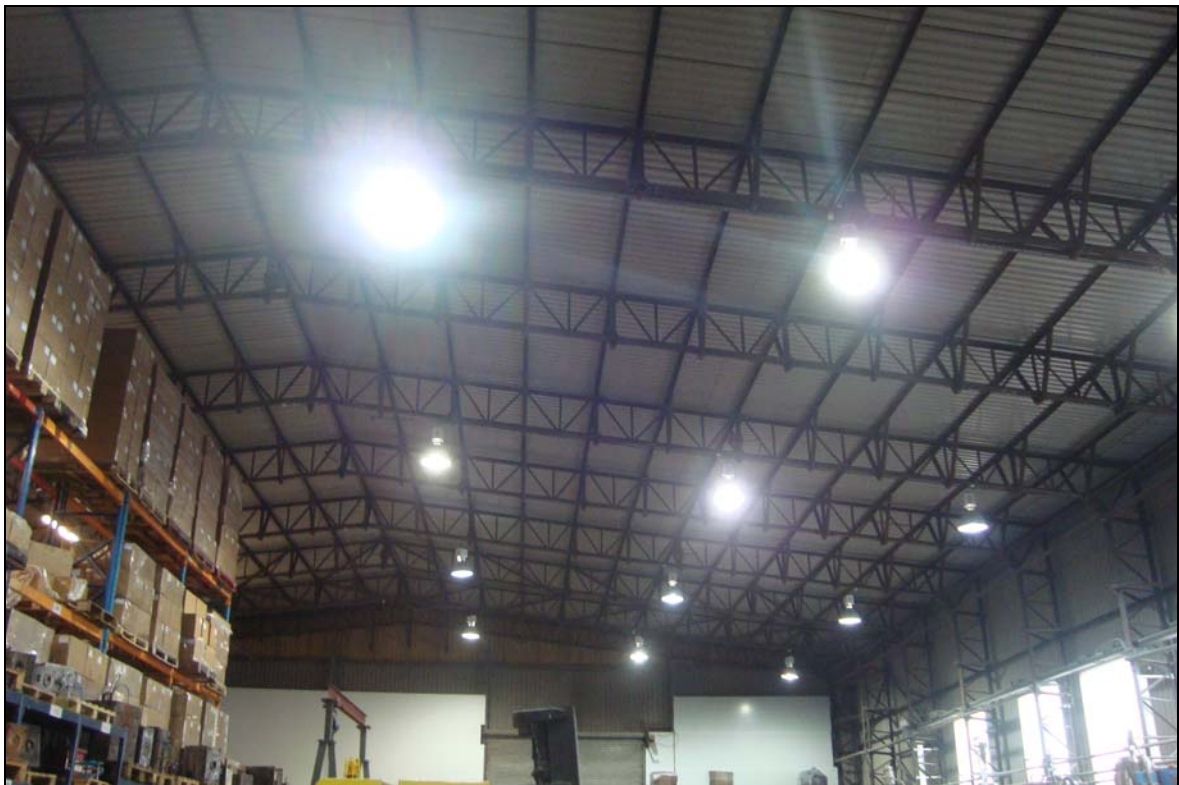
Plate 79: Internal steel frame structure of hangar 116.
