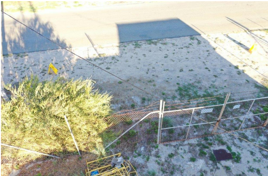
Figure 5 Existing access to subject site Source: Ventia 2021
