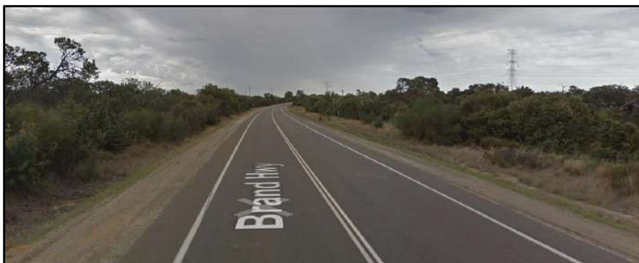
Figure 8 - Brand Highway Cross-section (Wannamal Road West intersection Looking South)
