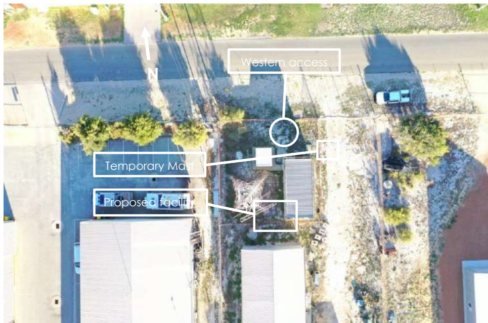
Figure 4 Existing access to subject site Source: Ventia 2022
