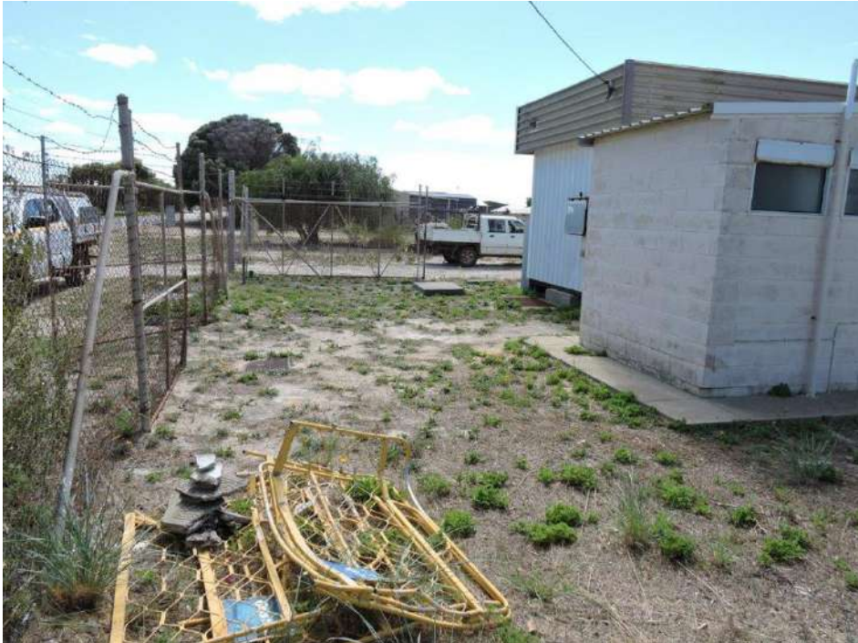
Figure 7 View north of site access gate Source: Ventia 2021
