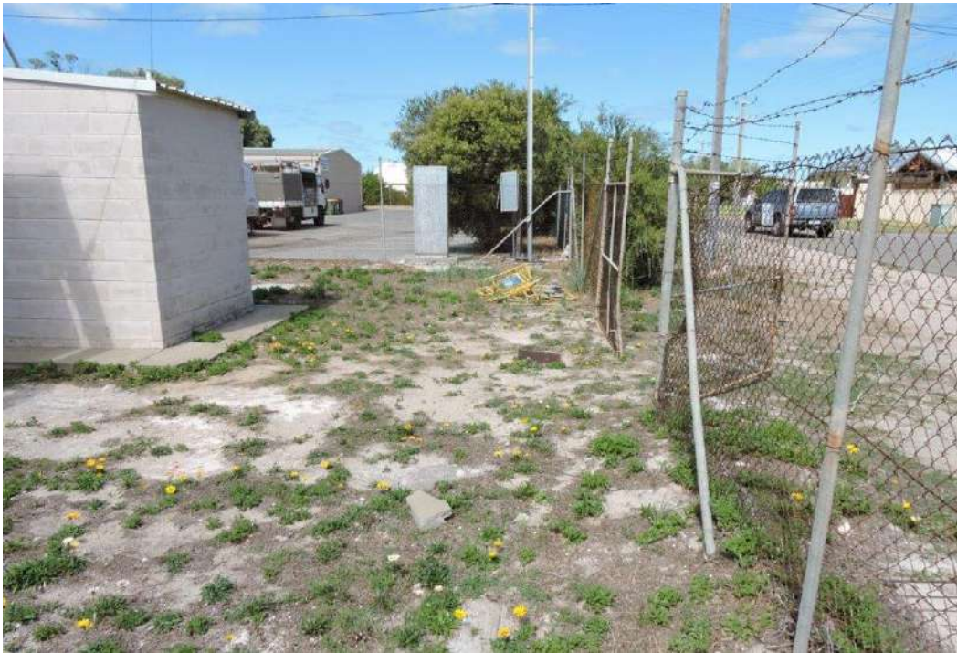
Figure 9 View south of site access gate Source: Ventia 2021
