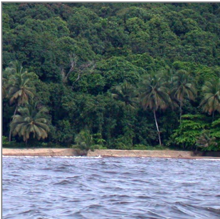
Plate A.3.2: Eroding section of beach near Ebodjé
