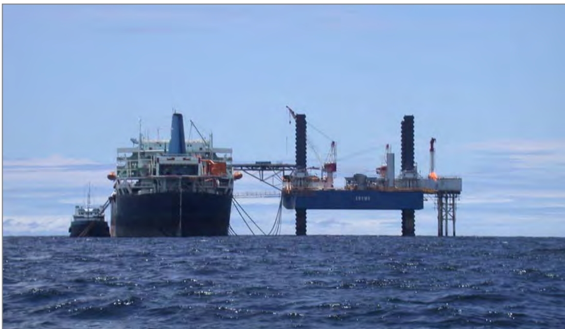
Plate A.2.1: Perenco's Ebomé platform situated offshore of Cameroon's southern coastline.
