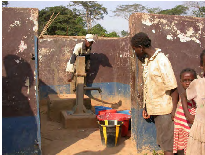
Plate A.3.3: Shallow (14 m) borehole with handpump supplying a village in the Lom and Djerem district.
