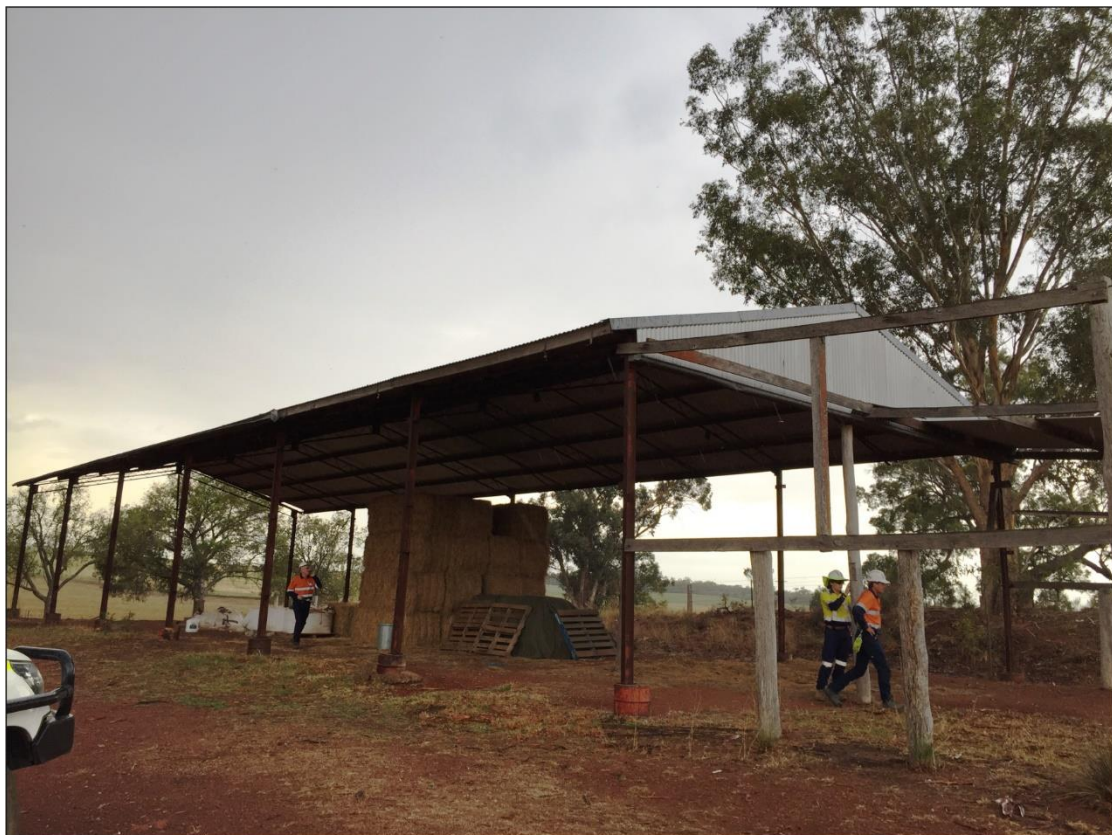
b) Overview of hay shed structure.
