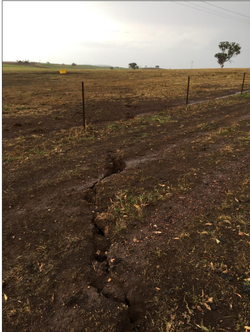
Figure 7: Cracking adjacent to Irrigation Road.
